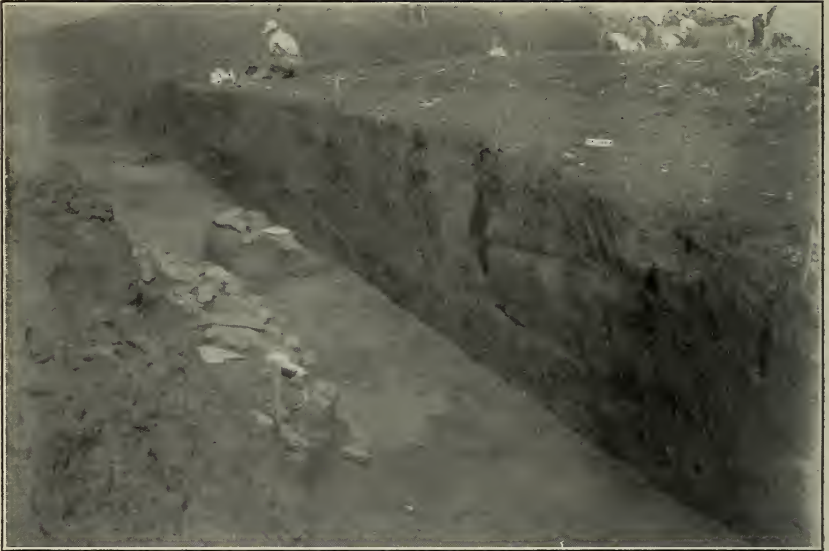
a. Wall 5.0-5.6 from southeast. Site No. 19.
