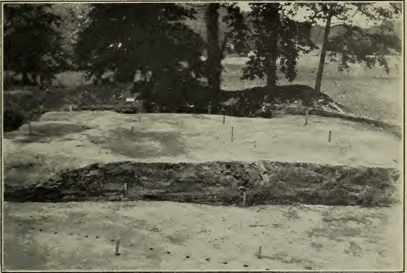
a. Post-mold pattern. Mound No. 2, Site No. 17.
