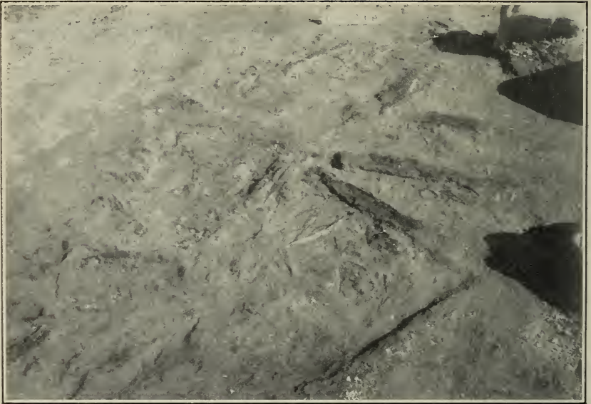
a. Burned structure. Feature No. 4, Site No. 11.
