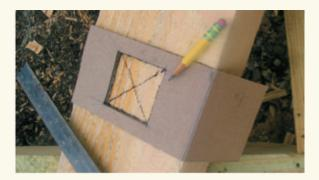
• With an electric drill and <sup>3</sup>/<sub>4</sub>" auger bit, bore out most of the waste material from the mortises, and finish with a 1<sup>1</sup>/<sub>2</sub>"
