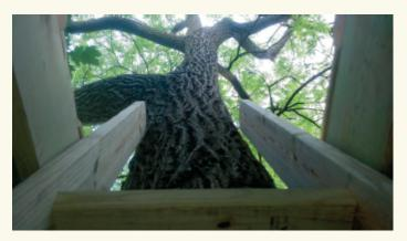
There's more than one way to build a treehouse in a single tree. If your tree isn't big enough or the right shape to enclose a house, you can supplement the tree trunk using other supports: either braces attached to the tree trunk, or posts that allow you to build a more substantial overhanging deck.
