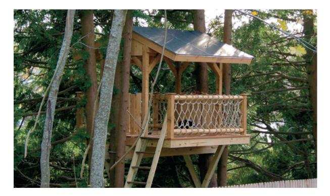
The treehouse is supported by girders under the floor joists, and by "V" braces under the side headers.
