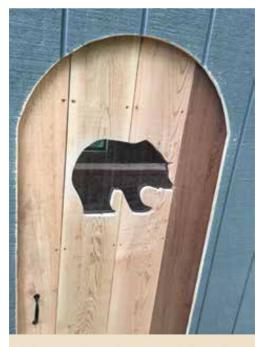
Silicone caulk on the outside helps seal this custom opening in the door.
