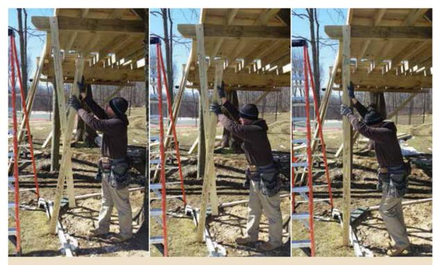
Left to right: Attach 2x4s together with RSS screw or single bolt. Push 2x4s to line them up, which lifts the beam or joist. Tack a second screw through both 2x4s to keep them from springing back while you work.
