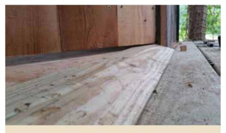
Homemade threshold beveled at 10 degrees to shed water outward
