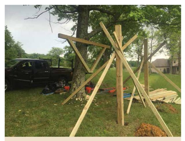
Holding a post plumb with temporary braces while stone or concrete is added
