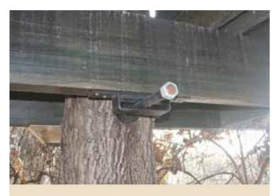
A slotted bracket allows trees to sway in any direction.
