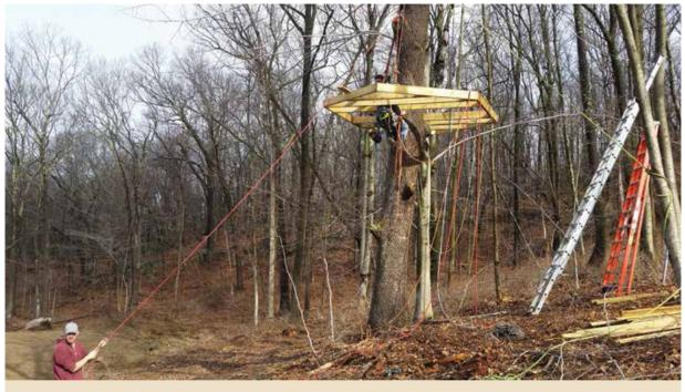
Lifting platform joists as one, using a 5:1 system and 1:1 balancing line
