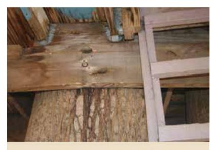
Tree pushing board over bolt head. New bolt was installed afterward.
