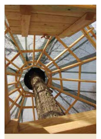
Smoke-tinted polycarbonate roofing over lath on gazebo roof frame
