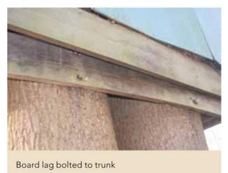
A pin attachment is where a wooden beam or joist is set flat against the tree bark and bolted or screwed directly into the tree. When an object touches a tree, one of two things will happen: The tree will envelop the object or push it away as the tree grows. When a structural beam is pinned to the tree, either option eventually leads to an
