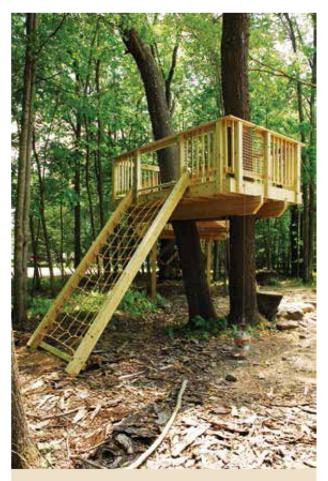
This cargo net is attached to 6x6 side rails and a pipe at the top as a grab bar.
