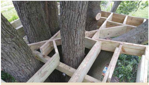
Joists are run at irregular angles to work around tree trunks in this spreading silver maple (Acer saccharinum).
