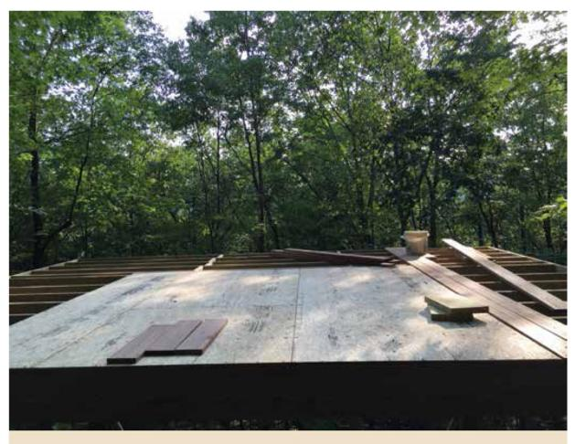
Start by installing the interior subfloor, leave a gap for drainage, and run exterior deck boards around the plywood.
