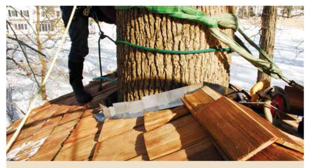
Rubber flashing, fashioned in place, is the best way to keep water out.
