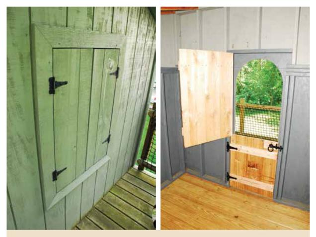
Left: Closed shutter windows in a homemade frame Right: Dutch door with separately hinged top and bottom
