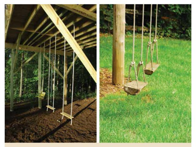
Left: These rustic plank swings use traditional swing-set hardware to attach to the treehouse. Right: These half-log swing seats are tied with a bowline knot.
