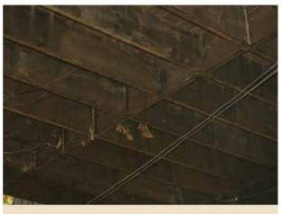
Scraps of joists can be installed perpendicular and tight to increase floor strength.
