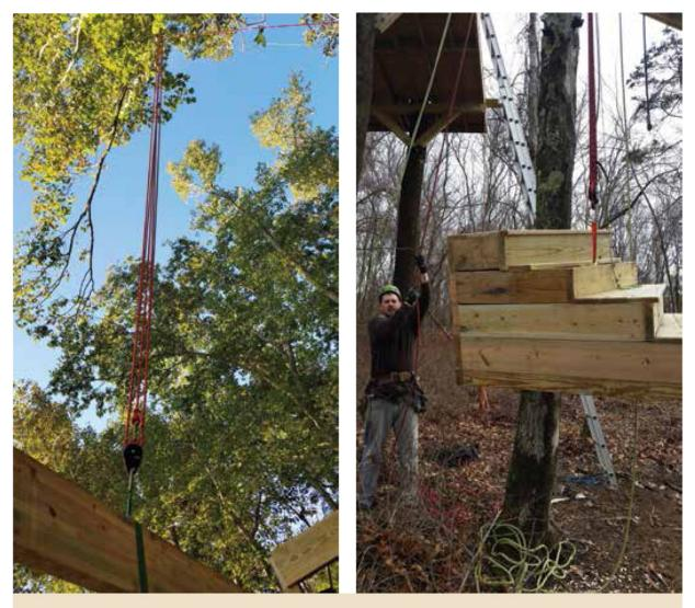
Left: Lifting large beams is done easily with the right equipment. Right: This section of turning stair tread was easier to build on the ground and then hoist into position.
