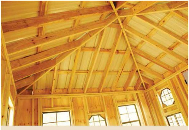
Metal roofing (white underside, color choices on top) over lath on hip roof frame
