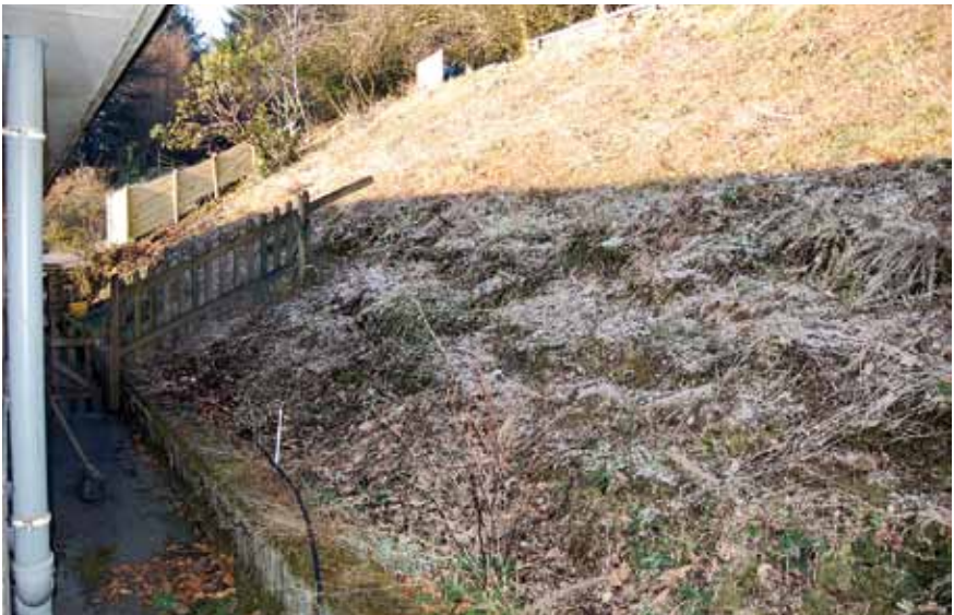
Frost pocket: The downhill flow of cold air off the moorland plateau is interrupted by the building, which is in turn chilled by the trapped air
