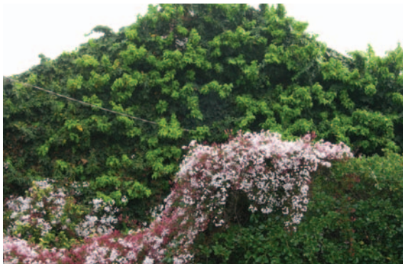
Figure 4.84 These climbers are well out of control and pose a threat to their support – in this case an entire house. Jasmine and ivy are a powerful mix.
