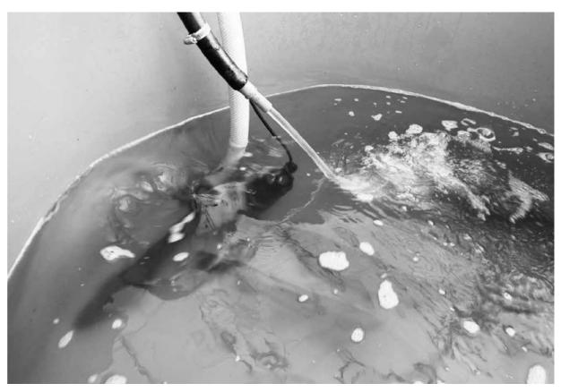
Purge tank with submersible pump for aeration and circulation.
