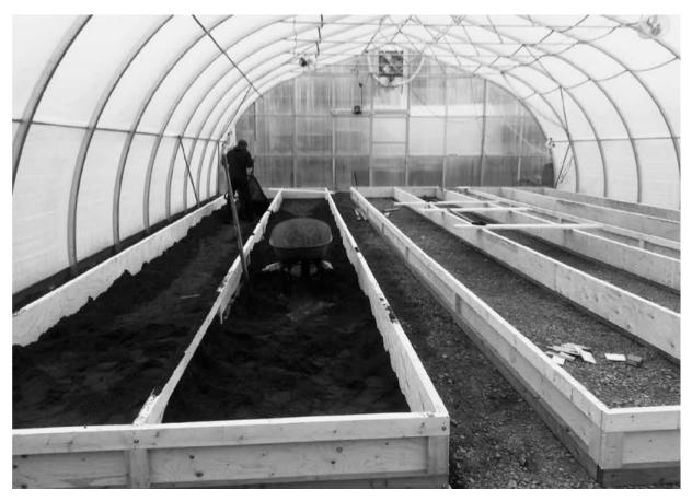
Laying the sand base in newly constructed troughs to protect the LDPE.
