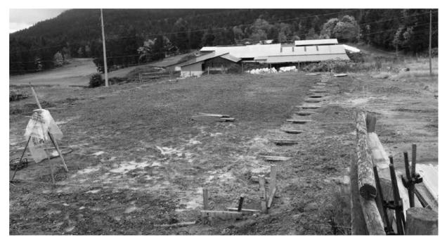
Foundation installation with string lines and batter boards, ready for concrete piers.
