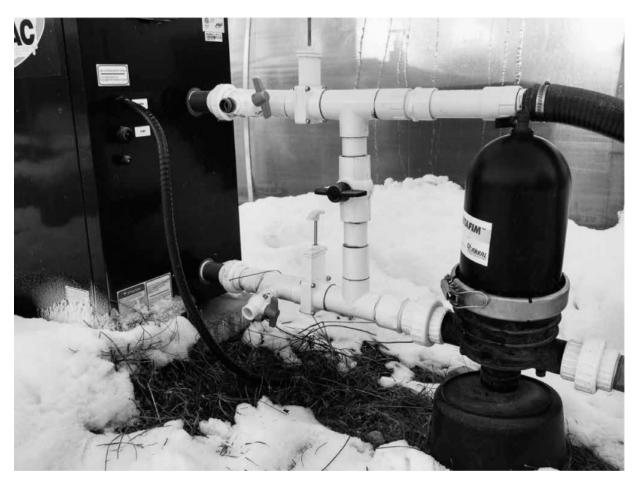
Heat pump bypass, inlet filter and flushing ports.
