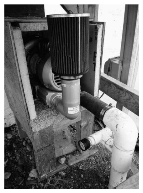
Aeration blower in sound-dampening box with front of box removed.
