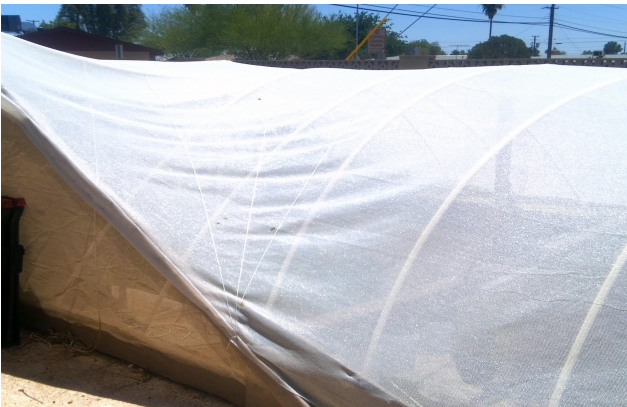
The loose shade-cloth has been secured with 1/8" braided nylon strings. This web prevents the looser areas of covering from moving too much in more extreme winds.
