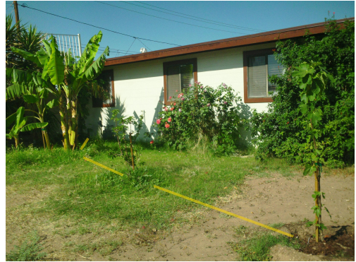
The yellow line shows where the 3/4" PVC is buried.
