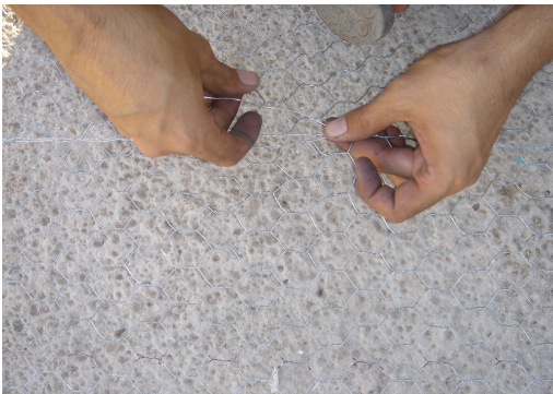
We braided the chicken wire together with 16 gauge wire.
