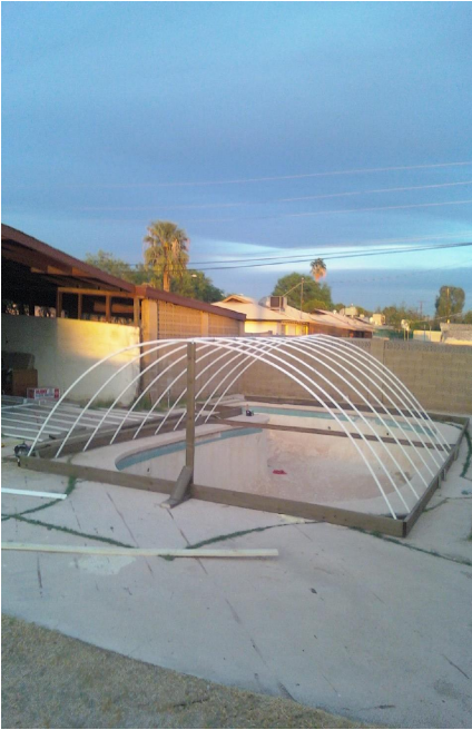
The first half has been installed.
