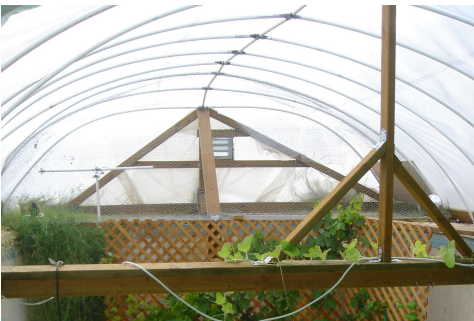
The GP has the reinforcement and lattice added.
