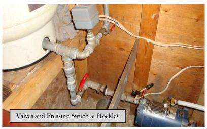
Now that my water line was connected from the pump to the lake, I had to finish plumbing the output side of the pump. Here's how I did that. On the output of the pump, I put another coupler. Then I installed a check valve (the check valve is another one-way valve), another Tee with a pressure gauge and then a shut off ball valve. The line out of the ball valve went to a pressure tank. Anywhere in the line to the pressure
