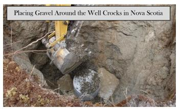
stone is to act as a course buffer and reservoir to allow water to easily collect and thereby fill the crock column. If we were to back fill with the material taken out of the hole we would be sealing off our well from the majority of the water source which defeats the purpose. Instead let that water infiltrate and become a reservoir around all that loose stone.
