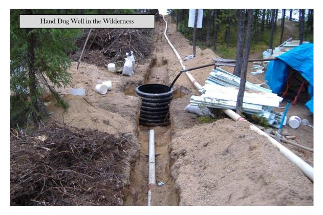
That dug well was in pure sand. If you've ever been to the beach and dug a hole in the sand, you know it's not long before the hole fills with water and the sides collapse. I came up with a way to deal with that problem though.
