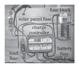
Example solar-power wiring configuration
