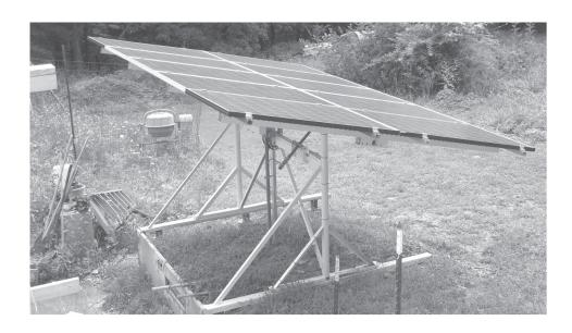
Metal racking with monthly repositioning
