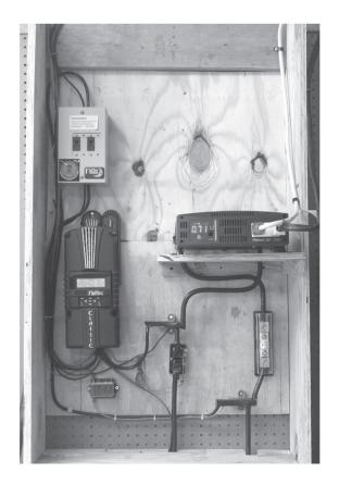
A friend's basic setup containing a solar breaker panel, charge controller, busbars, battery fuse, Whiz Bang Jr., and inverter
