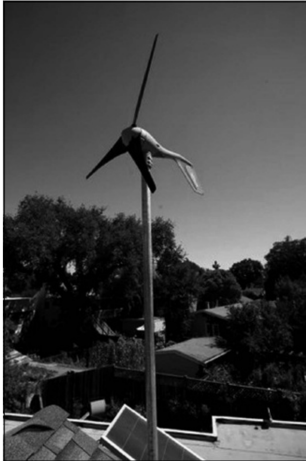
Small wind turbine powers computer and other small appliances. Photo by Ben Macri.
