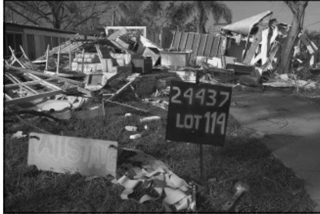
Hurricane Charley (2004) damage in Florida; this handmade sign identifies the house for the insurance adjuster. FEMA photo by Andrea Booher.
