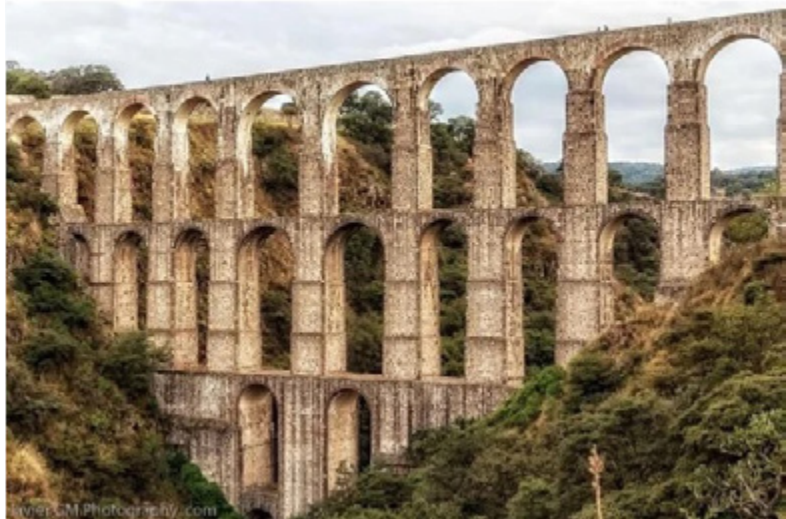
Aqueduct of Xalpa, Xalpa, Mexico; "Built by Jesuits in 1767"
