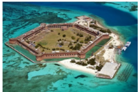
Fort Jefferson, Florida Keys, largest brick masonry structure in the Americas and is composed of over 16 million bricks. Star Fort
