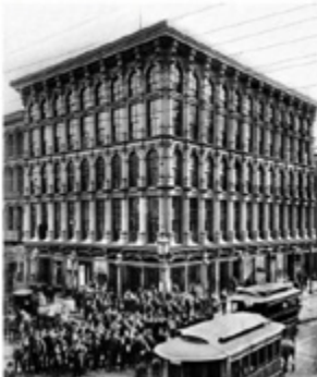
Sun Iron Building, Baltimore, Maryland (c. 1880-1890): Completed 1853, this was the first iron building finished in the U.S. It was destroyed in the Great Fire of 1904.
