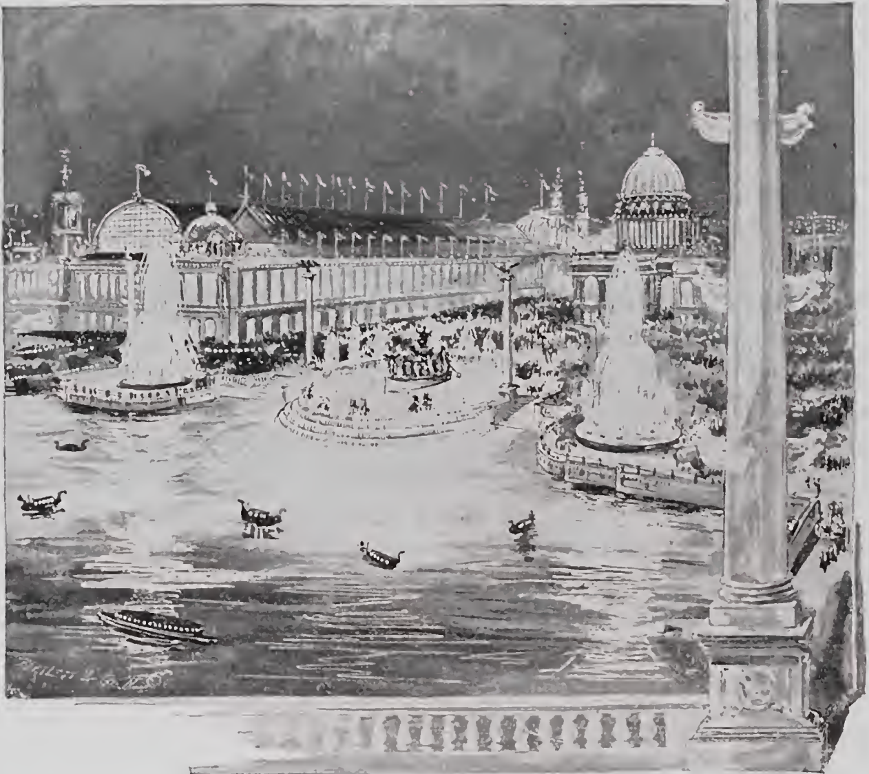
ELECTRIC FOUNTAINS AND ILLUMINATION
