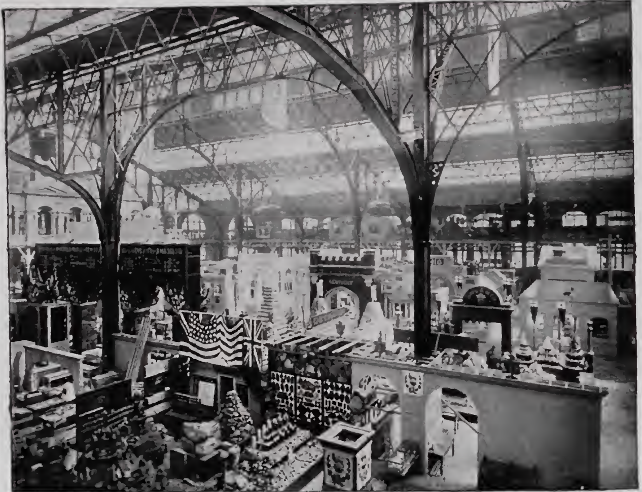
VIEW IN NORTH END OF BUILDING.
