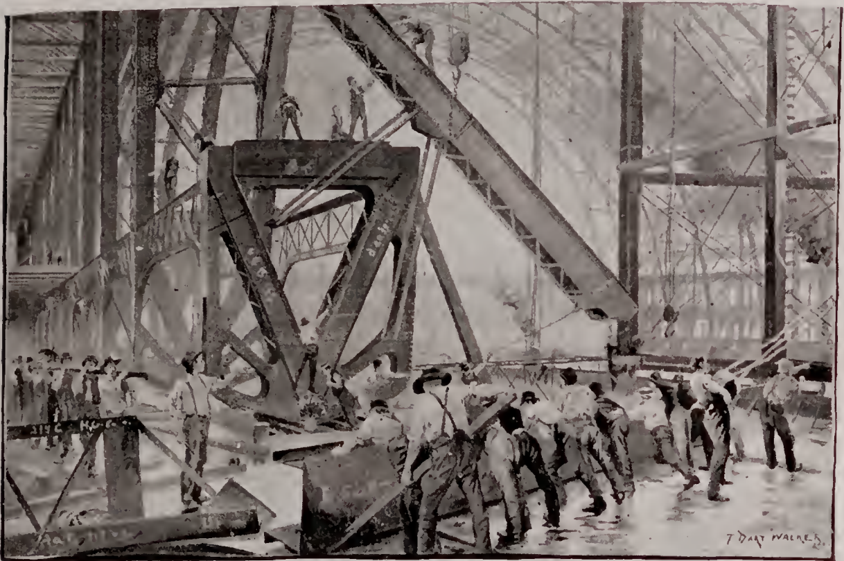
ERECTION OF MANUFACTURES BUILDING.
