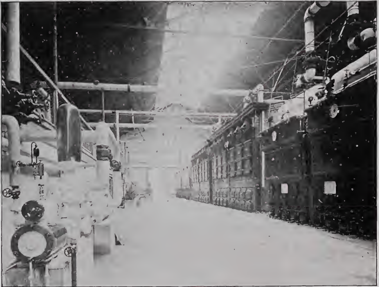
THE BOILERS IN MACHINERY HALL.
