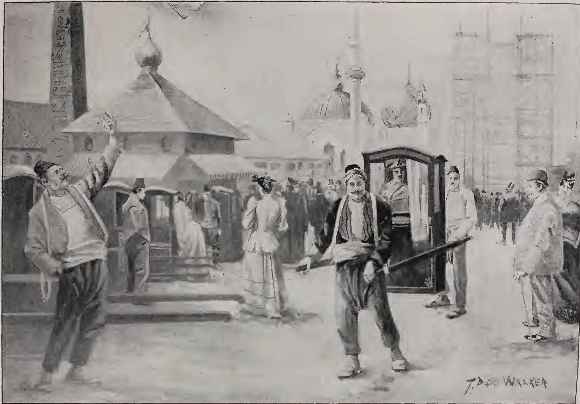
560 TYPICAL SCENE IN THE PLAISANCE.—FERRIS WHEEL IN THE DISTANCE, DURING CONSTRUCTION.
