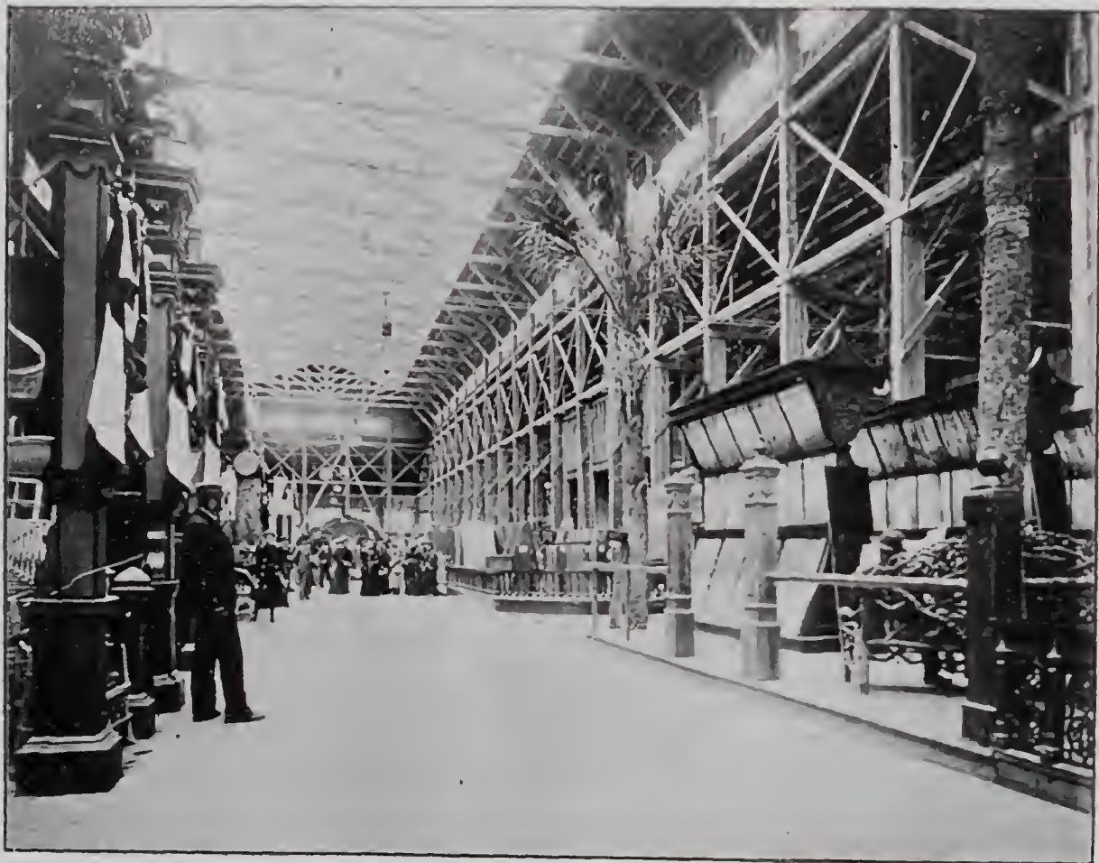
INTERIOR OF FORESTRY BUILDING.
