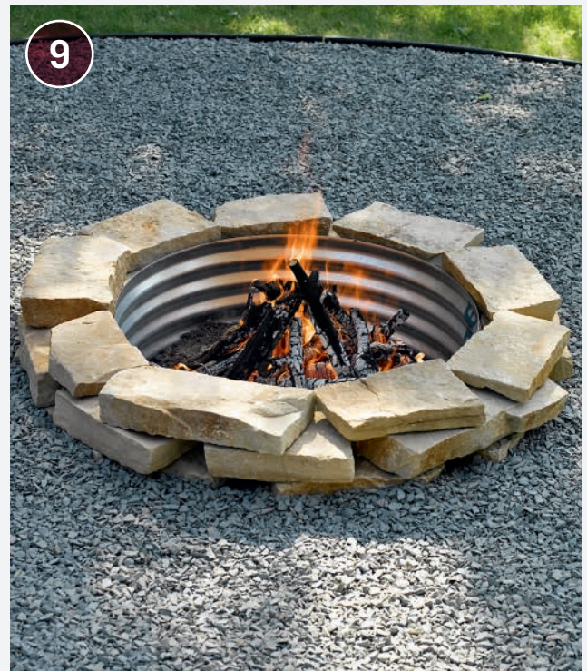
9 Place and compact a later of top-dressing rock in the seating/safety area to complete the fire pit.
