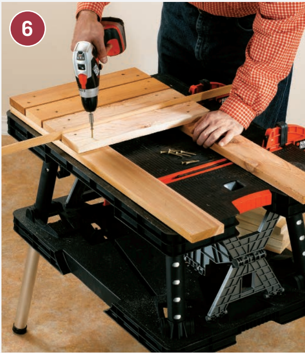
Attach the door siding boards to the door stiles. The top door siding board is attached with only one screw in each end.
