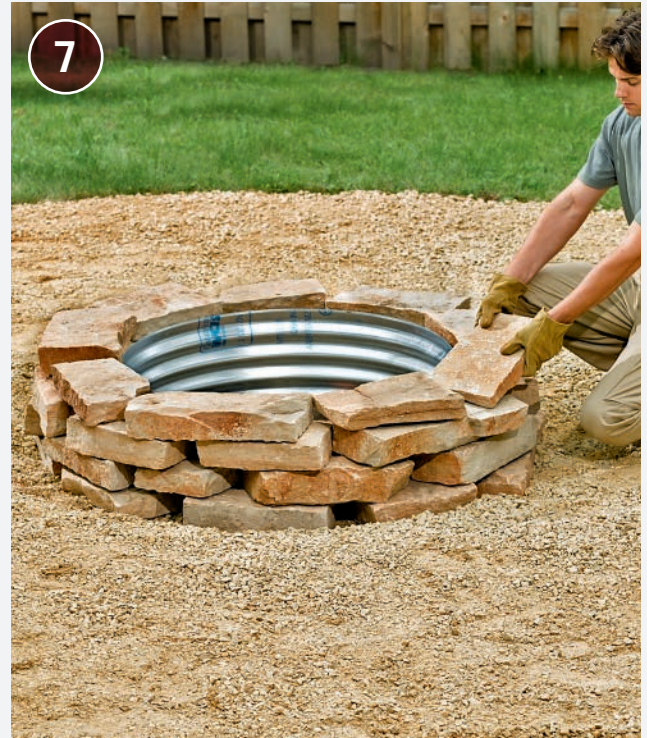
7 Install the second course of wall block , taking care to evenly stagger the vertical joints on the first and second courses. Add the remaining courses to the desired height.
