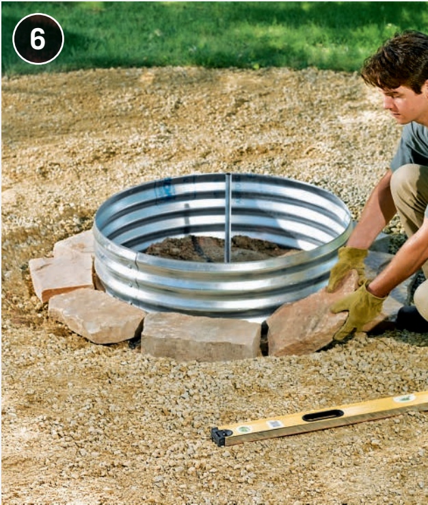
6 Arrange the first course of wall blocks around the fire ring. Keep gaps even and check with a level, adding or removing gravel as needed.
