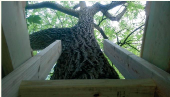
There's more than one way to build a treehouse in a single tree. If your tree isn't big enough or the right shape to enclose a house, you can supplement the tree trunk using other supports: either braces attached to the tree trunk, or posts that allow you to build a more substantial overhanging deck.
