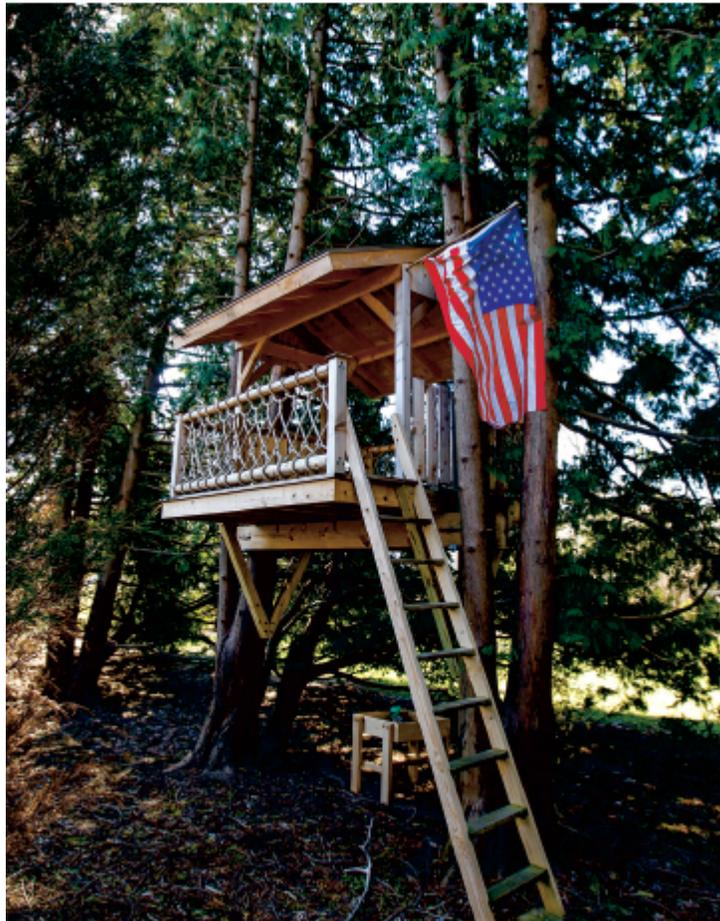
Supports for the treehouse are another consideration. Posts are the easiest, and allow usable space underneath the tree to sit, walk or play. On the other hand, braces blend in more with the tree trunk and are less noticeable. You can even make braces from branches sawn off the tree itself, disguising the fact that you needed braces at all.
