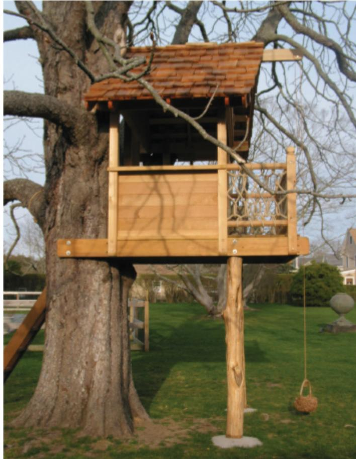
It's usually better to keep the floor about six or seven feet from the ground: it's easier and safer to build the platform of a treehouse from the ground; the supporting tree will be much stronger at this height than at the crown, and less likely to be affected by the wind; and treehouses are less conspicuous closer to the ground, and a bit easier for young children to navigate.
