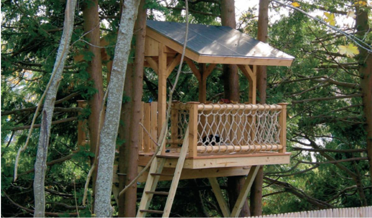
The treehouse is supported by girders under the floor joists, and by “V” braces under the side headers.
