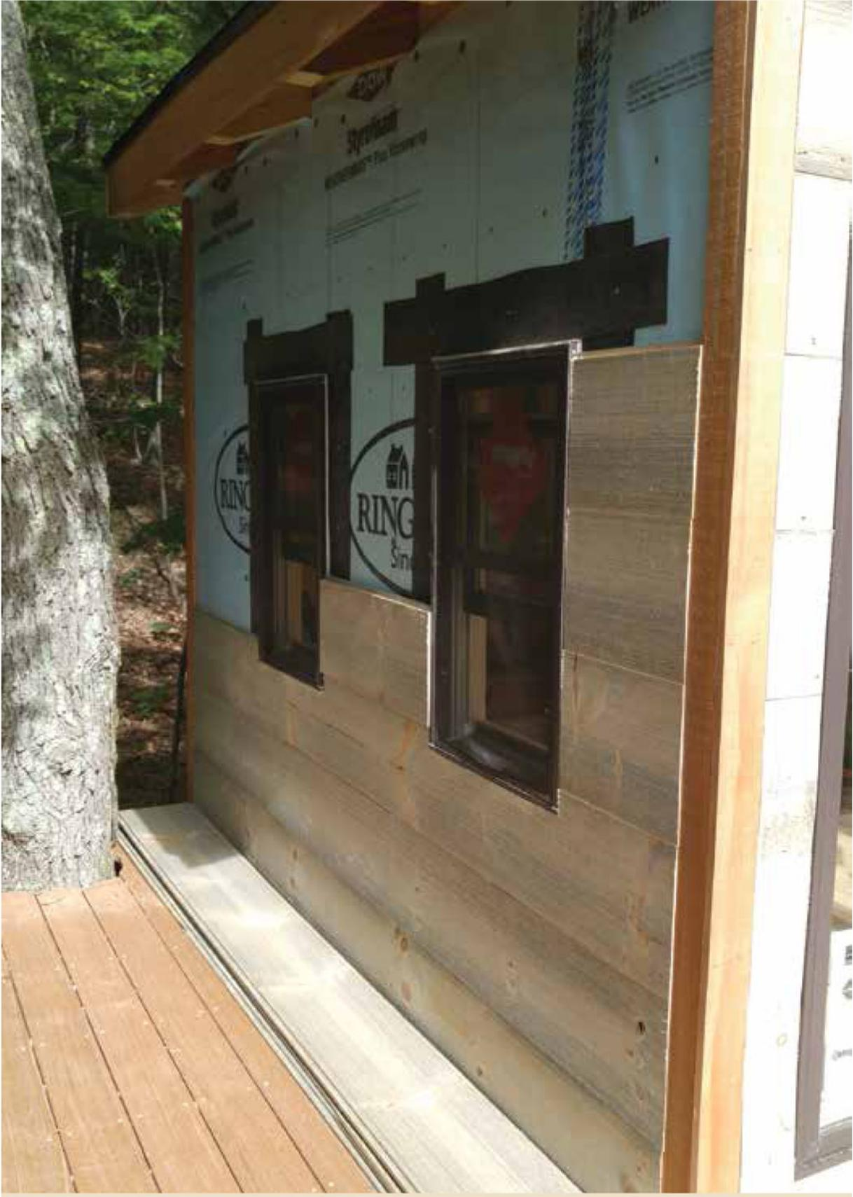
Four-season climate-controlled treehouses need insulation and weatherproofing layers.
