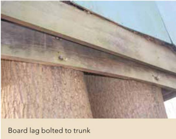
A pin attachment is where a wooden beam or joist is set flat against the tree bark and bolted or screwed directly into the tree. When an object touches a tree, one of two things will happen: The tree will envelop the object or push it away as the tree grows. When a structural beam is pinned to the tree, either option eventually leads to an
