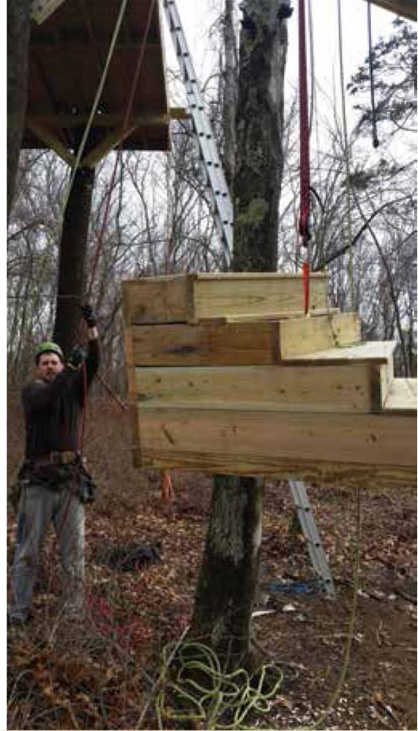
Left: Lifting large beams is done easily with the right equipment. Right: This section of turning stair tread was easier to build on the ground and then hoist into position.
