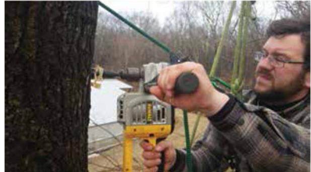
Start the hole with a 3-inch timber bit.
