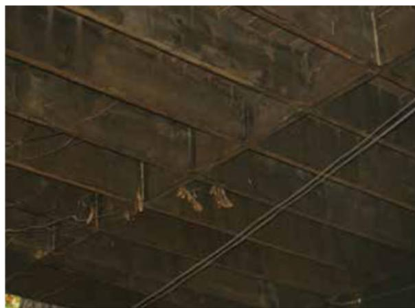
Scraps of joists can be installed perpendicular and tight to increase floor strength.
