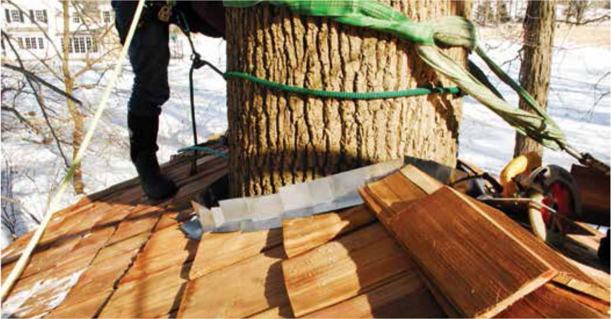
Rubber flashing, fashioned in place, is the best way to keep water out.
