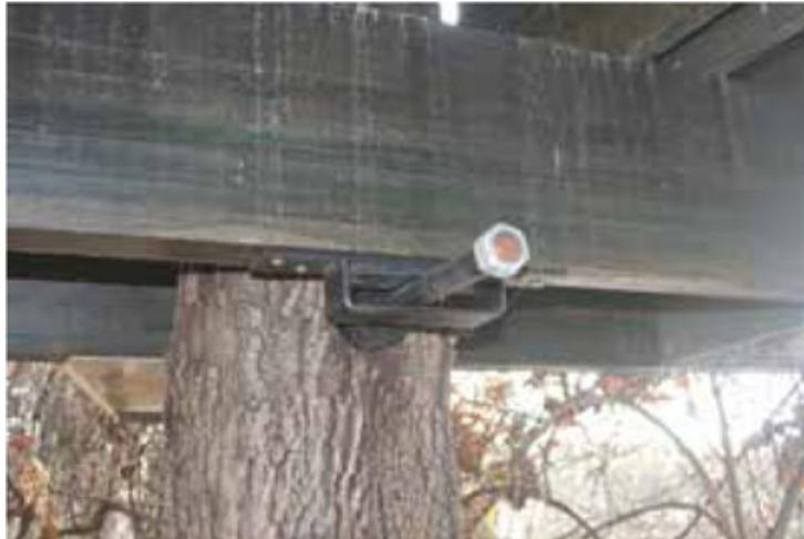
A slotted bracket allows trees to sway in any direction.
