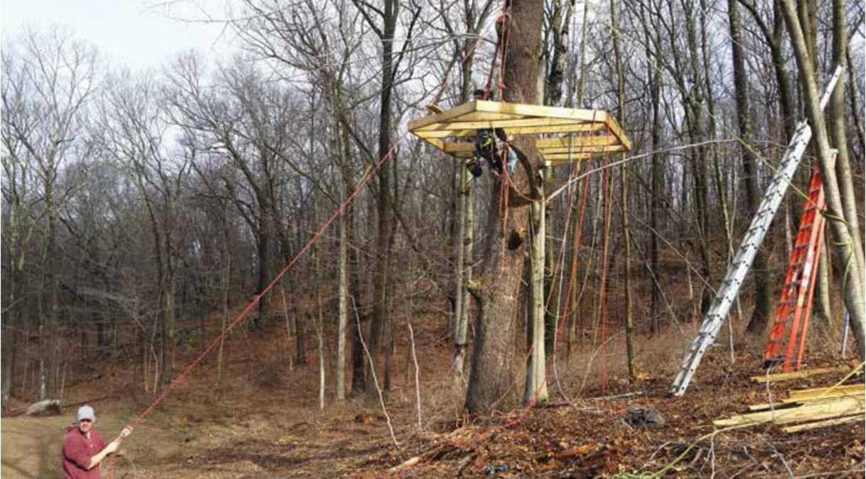
Lifting platform joists as one, using a 5:1 system and 1:1 balancing line
