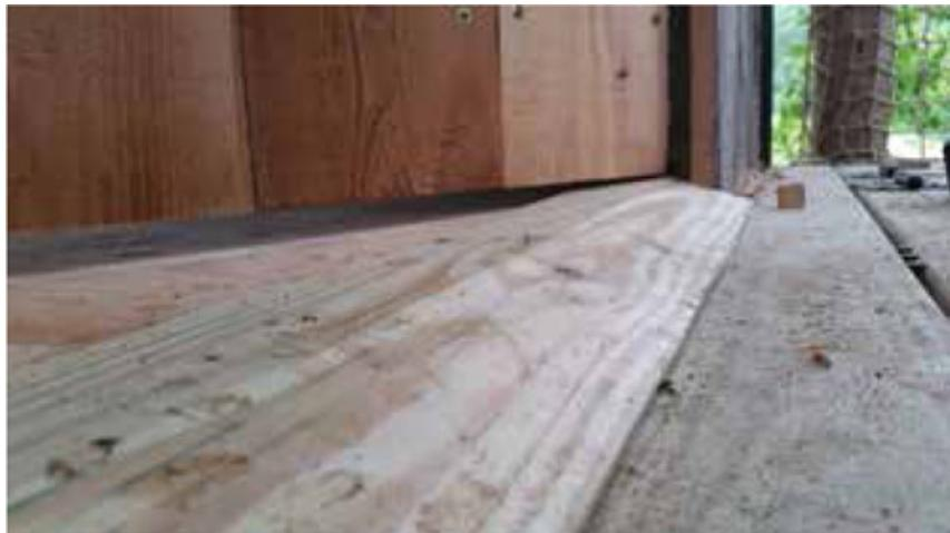
Homemade threshold beveled at 10 degrees to shed water outward
