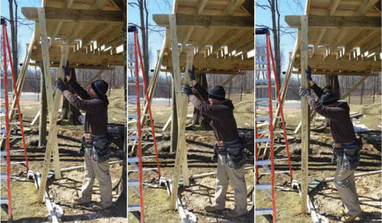
Left to right: Attach 2x4s together with RSS screw or single bolt. Push 2x4s to line them up, which lifts the beam or joist. Tack a second screw through both 2x4s to keep them from springing back while you work.
