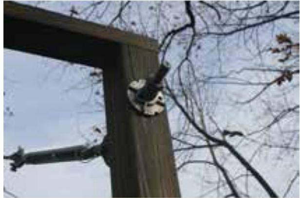
Extra washer and nut added to allow inspection after tree growth
