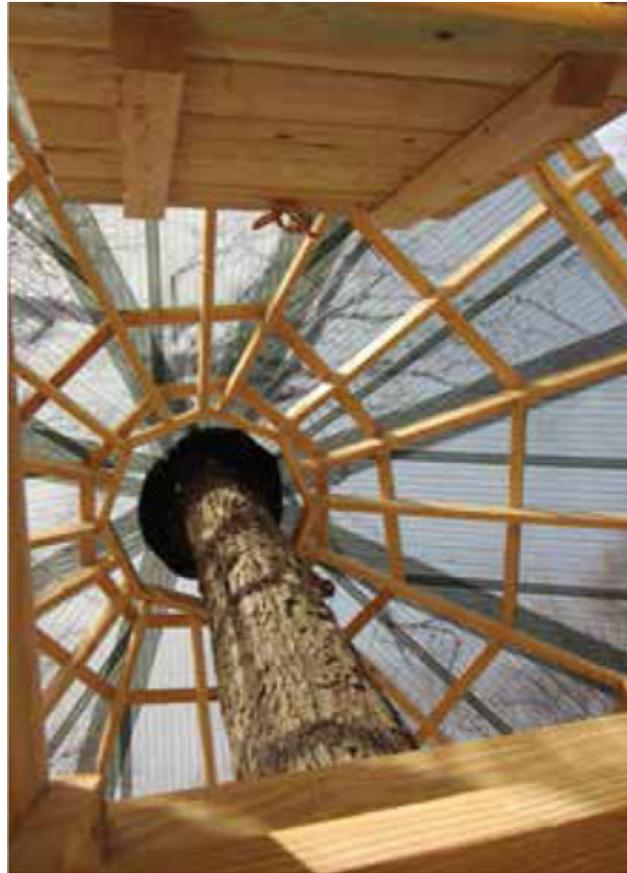
Smoke-tinted polycarbonate roofing over lath on gazebo roof frame
