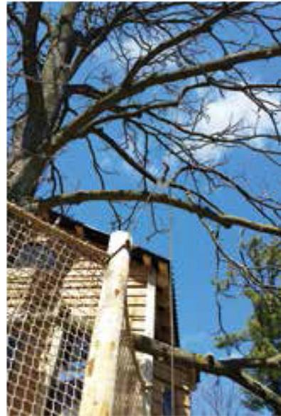
The pulley is attached to an overhead branch so that the rising bucket clears the edge of the railing.
