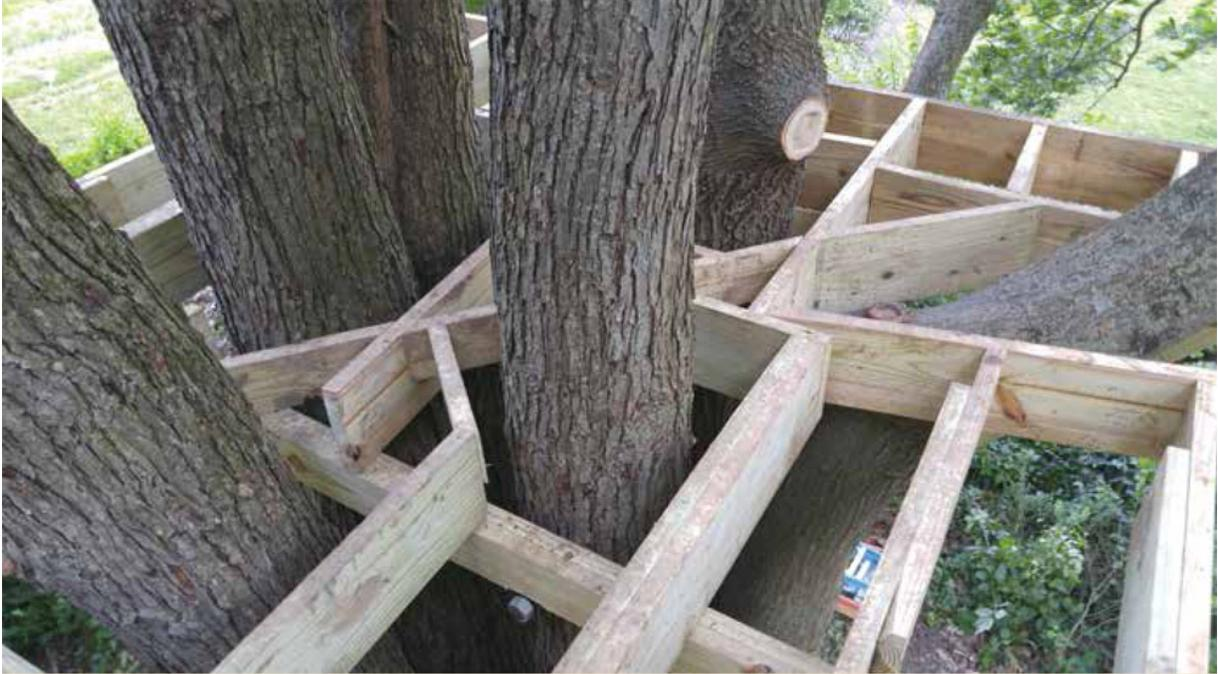
Joists are run at irregular angles to work around tree trunks in this spreading silver maple (*Acer saccharinum*).
