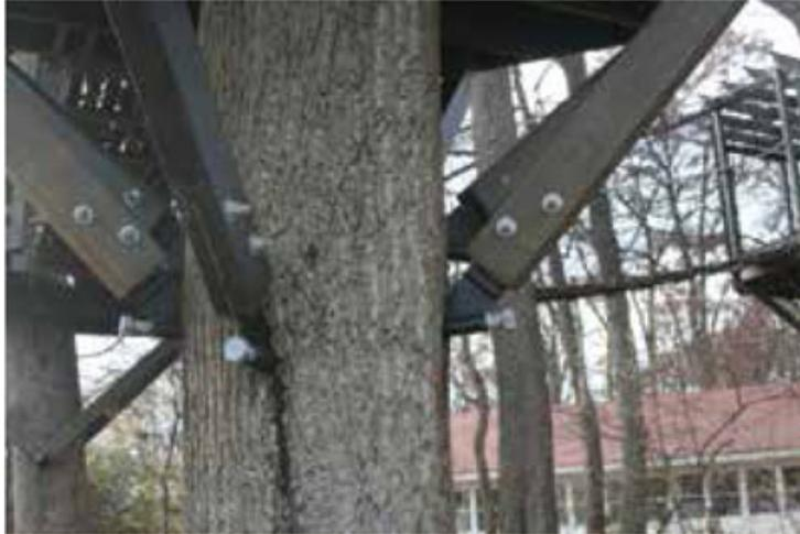
Single knee brace brackets support the perimeter of a platform.
