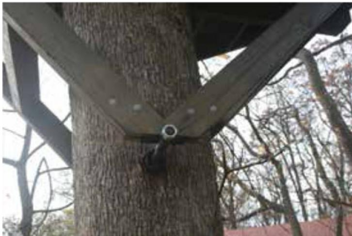
Double knee brace bracket secures two braces to a single TAB.
