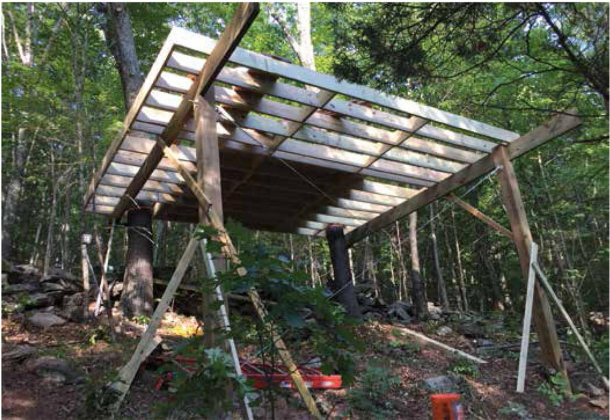
Wires forming an X shape add stability to the posts.
