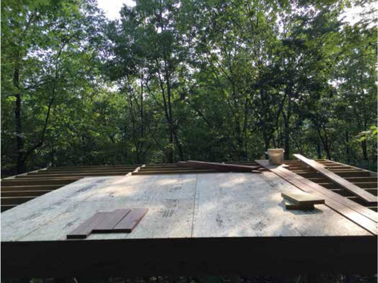
Start by installing the interior subfloor, leave a gap for drainage, and run exterior deck boards around the plywood.
