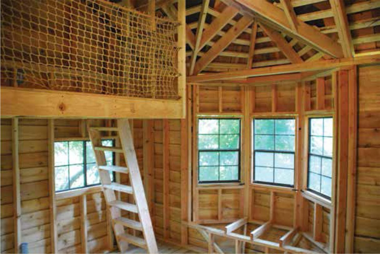
Siding and roofing applied directly to framing in one layer
