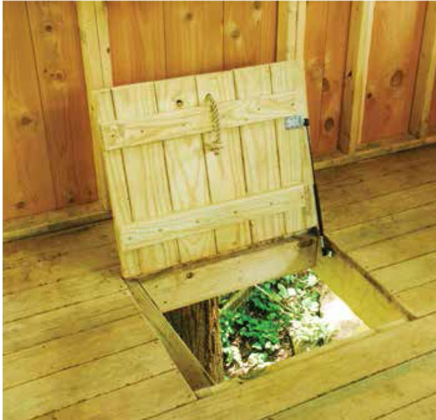
The piston hinge slows the closing of the trapdoor and makes it easier to open.
