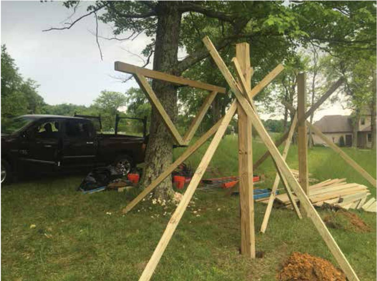
Holding a post plumb with temporary braces while stone or concrete is added
