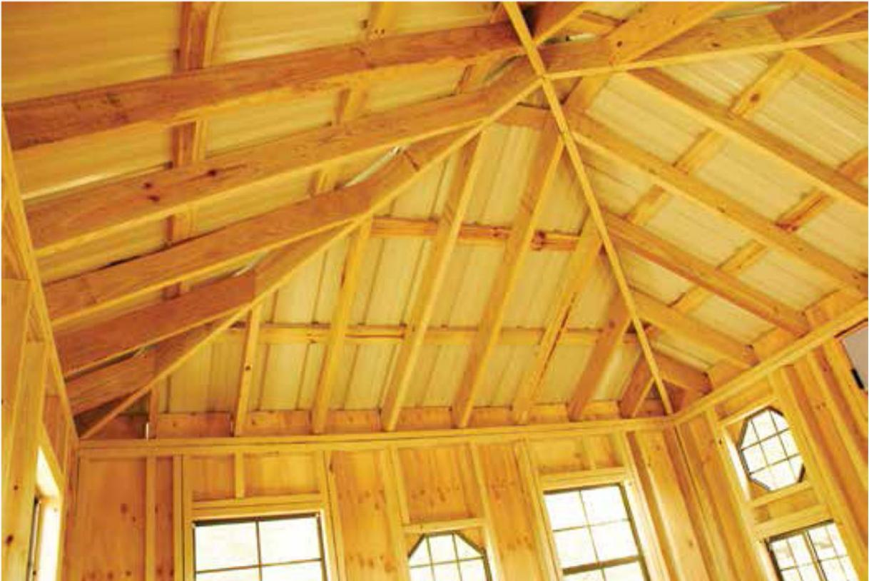
Metal roofing (white underside, color choices on top) over lath on hip roof frame
