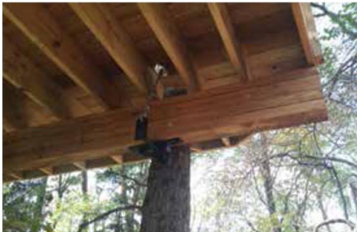
Suspension plates allow reinforcement of the TAB under high loads.
