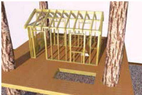
Normally I suggest framing all the walls on the ground and lifting them into position with the help of a friend or hoist system. However, with the size of this platform, the best place to frame the walls is right on the platform. Frame the window and door rough openings per the
