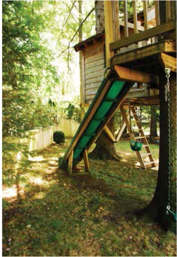
Back of sectional slide shows side rails and supports.
