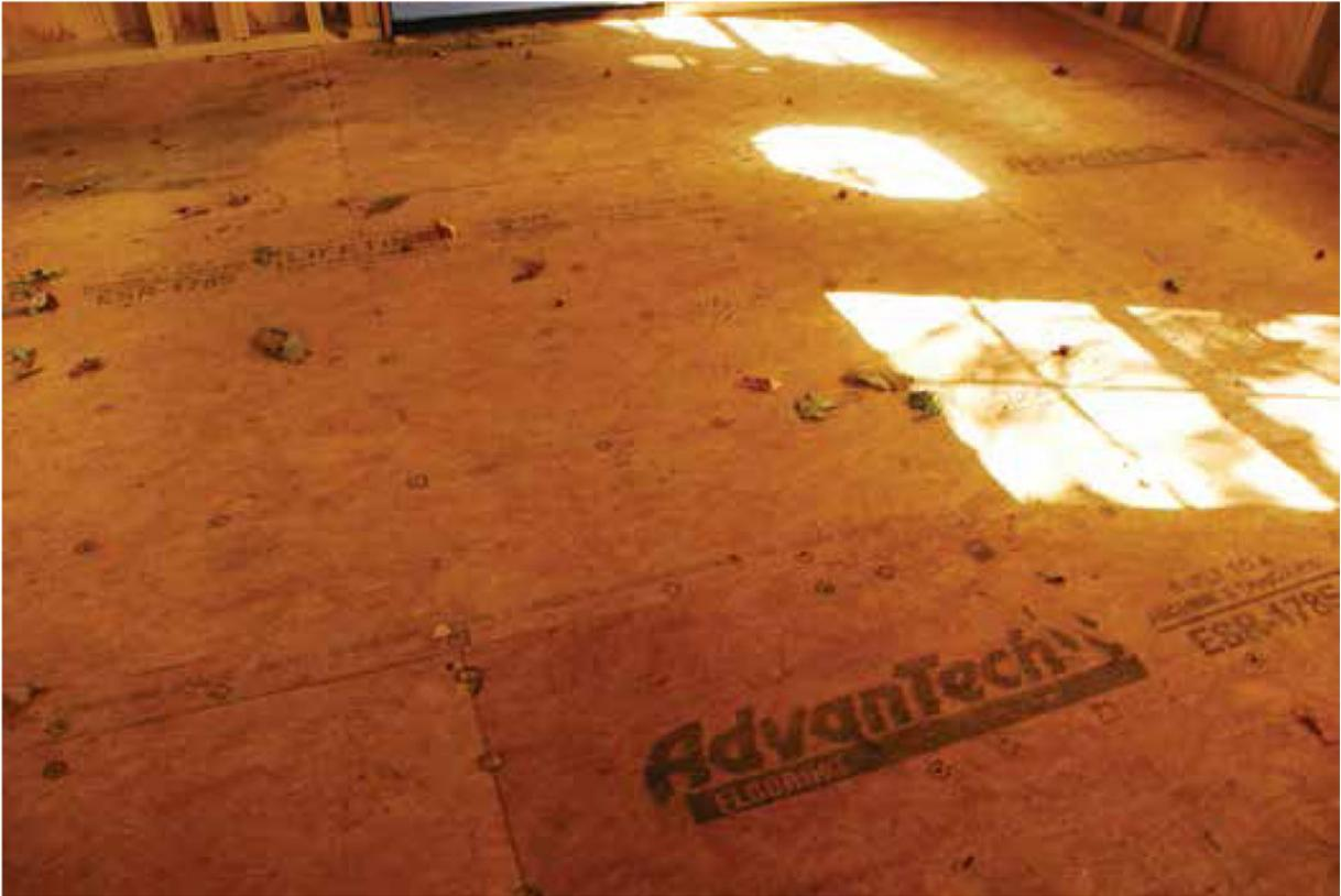
A solid interior subfloor is  $\frac{3}{4}$  inch thick and moisture resistant.
