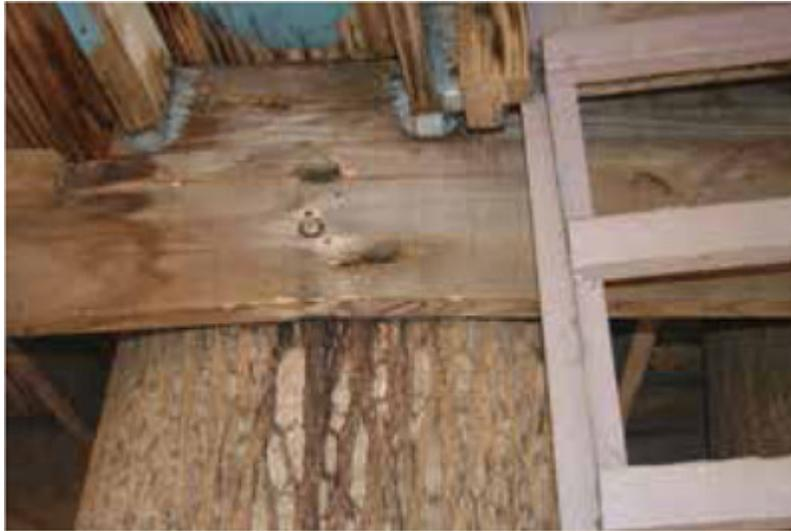
Tree pushing board over bolt head. New bolt was installed afterward.
