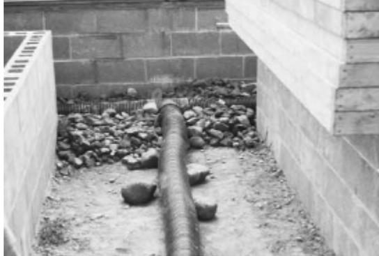
*The ventilation pipes in the deep beds delivery warm air to the soil at Three Sisters Bioshelter.*
