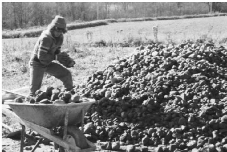
*Thirty tons of stones provide thermal mass in Three Sisters Bioshelter.*
