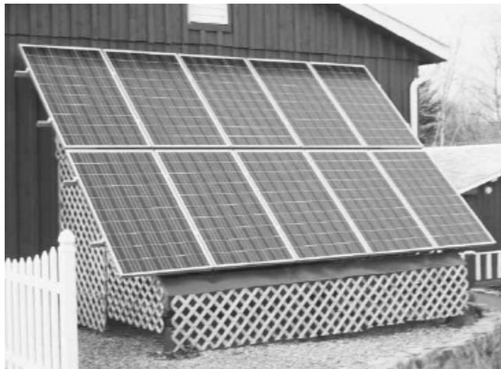
*Grid tied solar array at Sally's Cider Press offsets electricity used in cider sterilization.*
