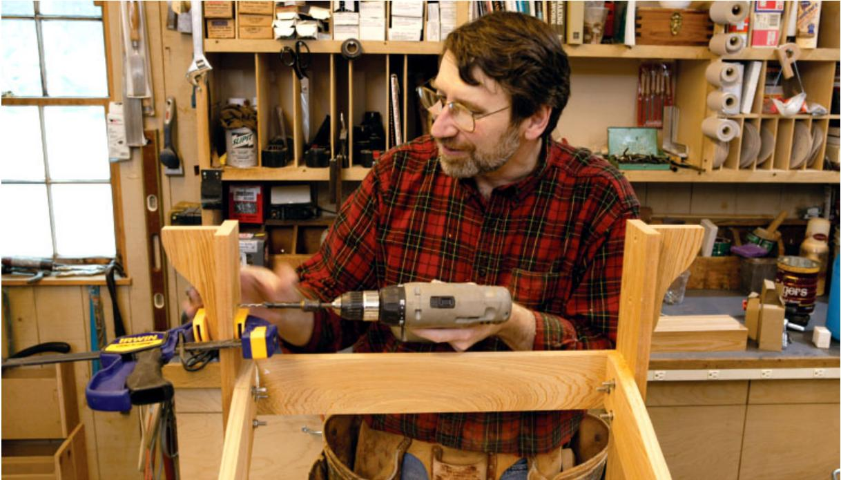
*Position and clamp the arm bracket then drill and countersink for two screws. The top edge of the support should be flush with the top of the leg and centered in the width dimension of the leg.*
