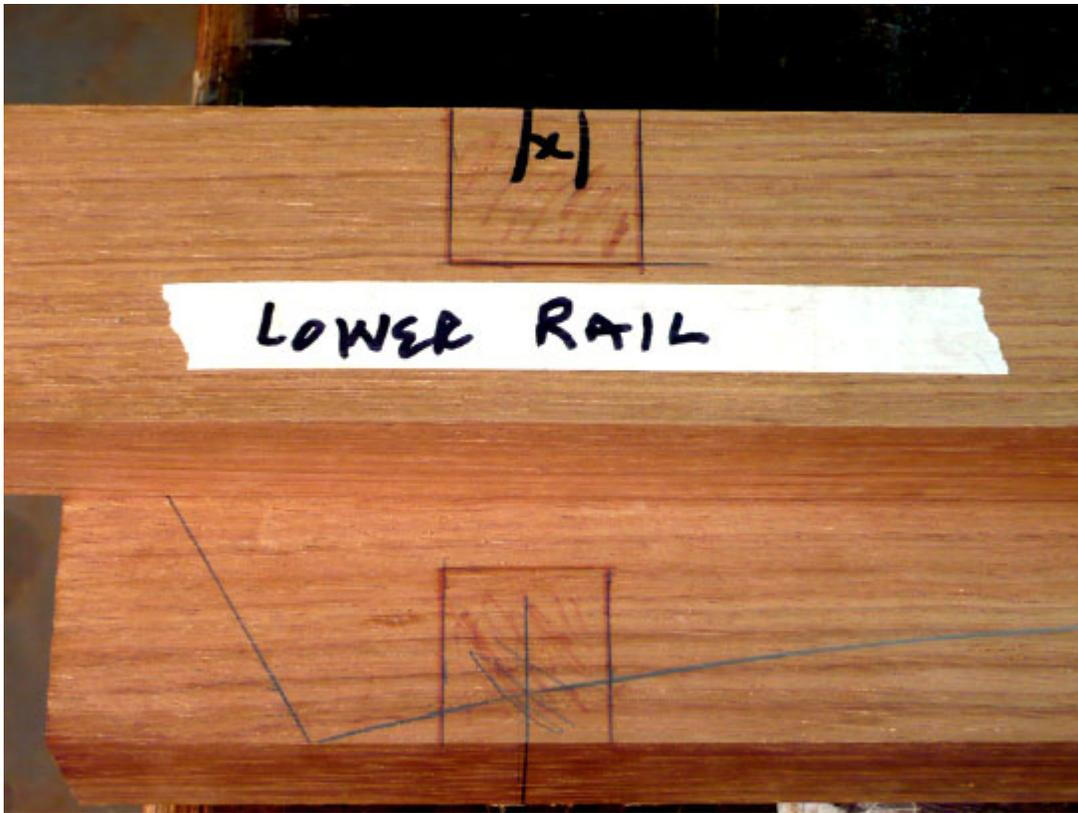
**Mark The Notches.** Carefully mark the notches for the rails. Here, a lower rail blank is lying on top of the stretcher blank.
