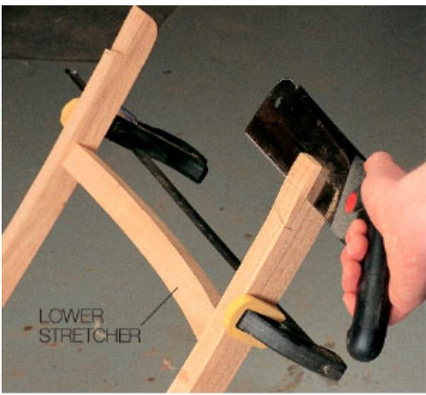
**Step Three** *Using the lower stretcher to maintain the proper spacing, the crest rail is held in place and the notches are marked on the legs then cut and hand fit.*
