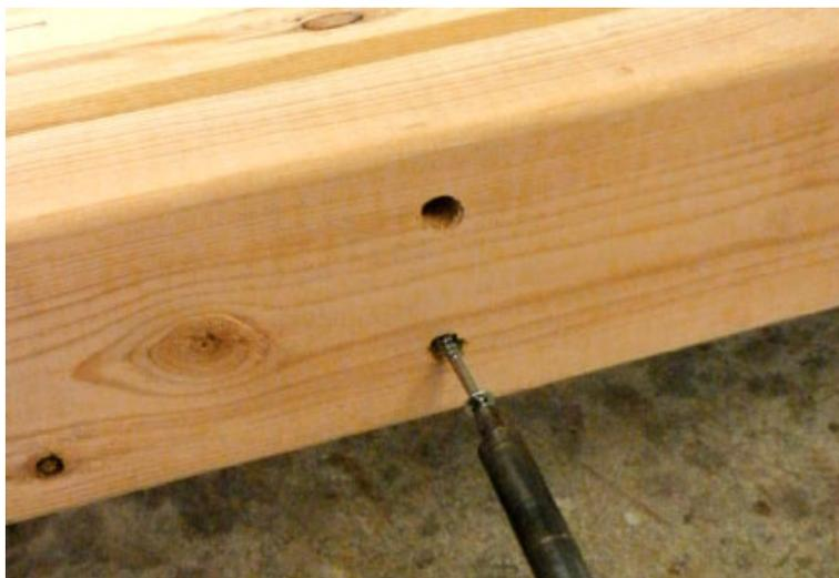
**Step 18** *The brace can be secured through the stretchers on the front and rear of the bench. I also recommend screwing and nailing down through the top of the slats into the brace.*
