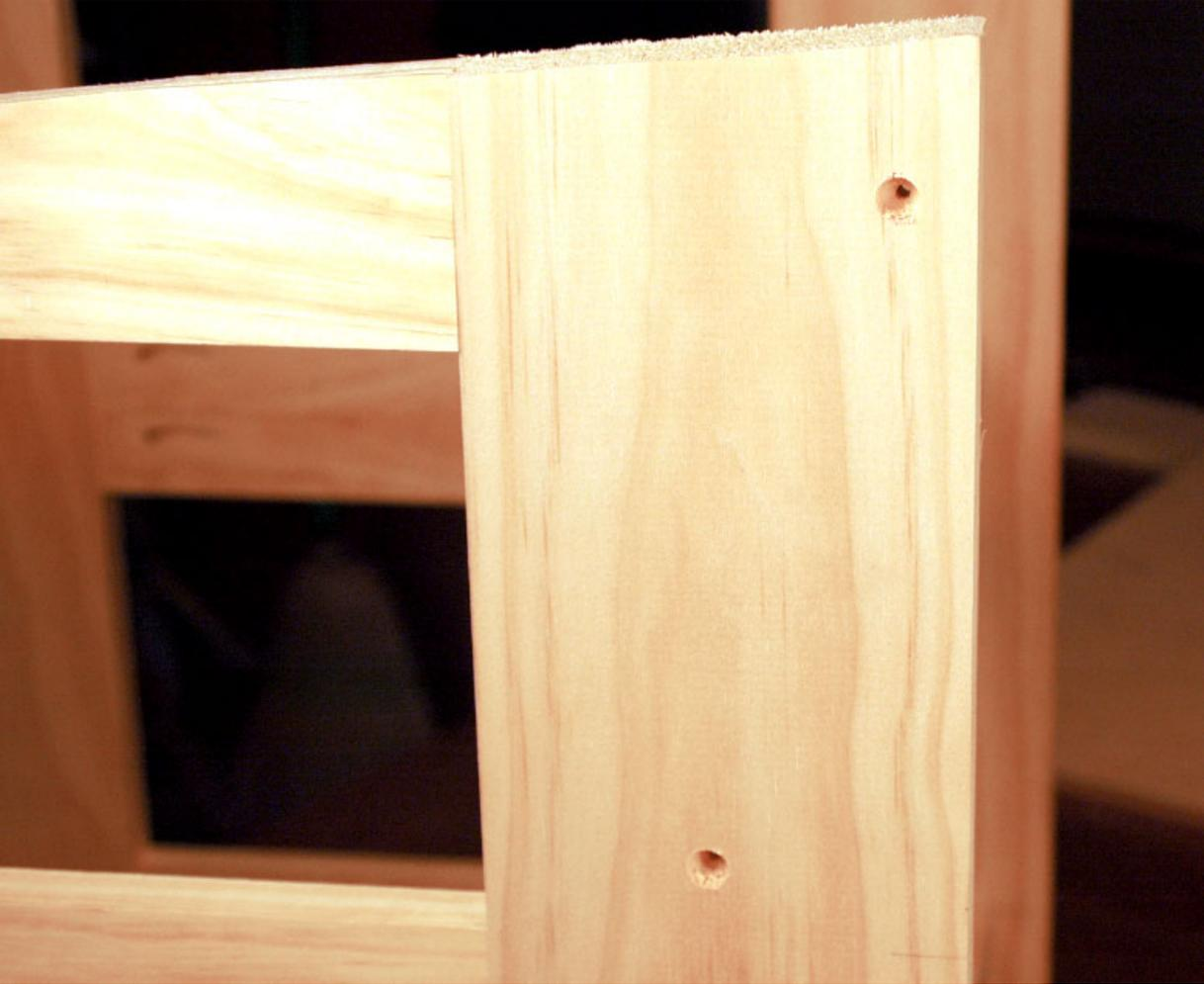
**Step 11** *I then came from the outside surface of the sides, drilling deeper to countersink the holes for plugs.*
