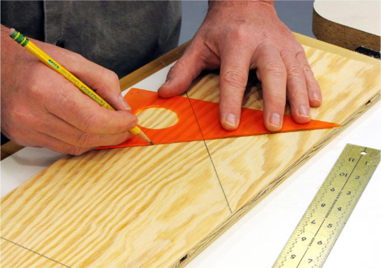
**Figure 1** Lay out the cutlines for the front/back parts
