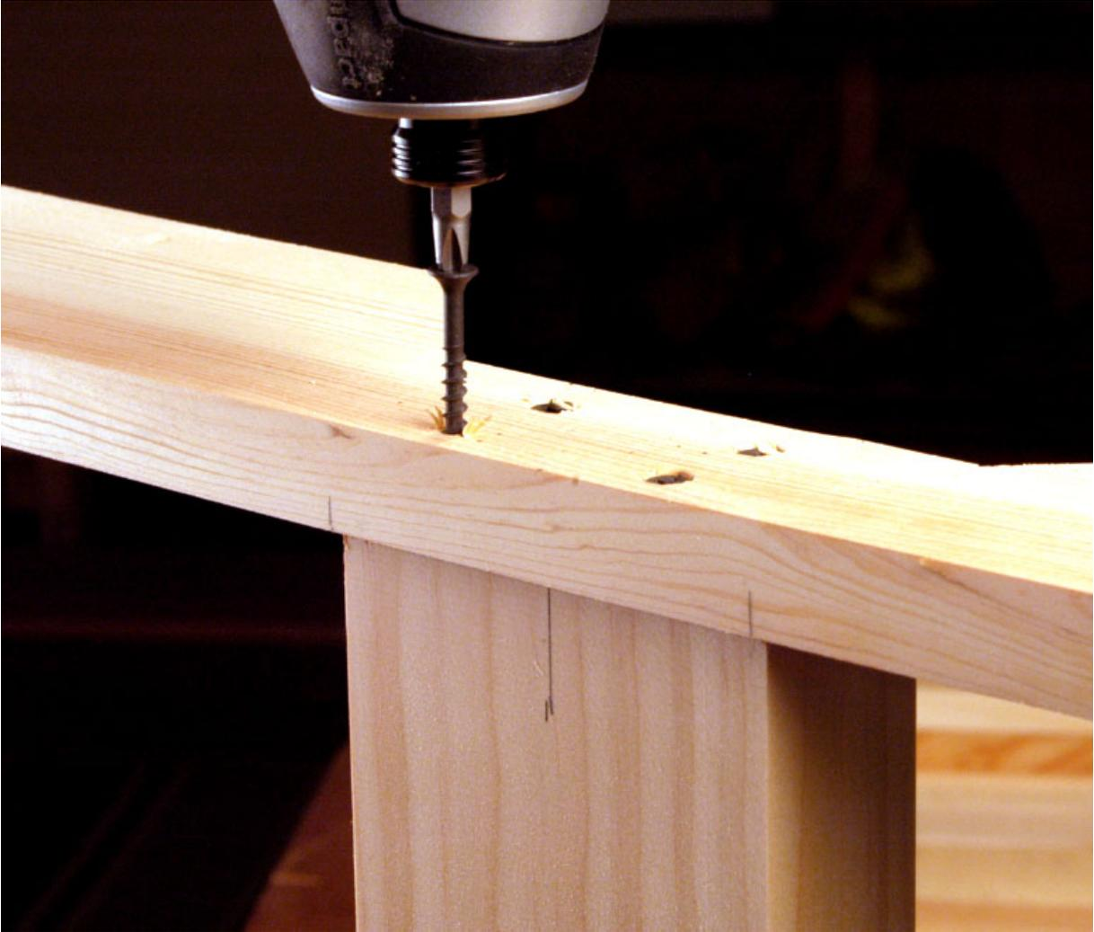
**Step Seven** I used 2 ½"-long screws to attach the inner bracket feet. I didn't countersink or plug these holes on my table, but were I to do it over, I think I'd take that step the second time around, as these were the only visible (but fairly well hidden) screws when the table was complete.
