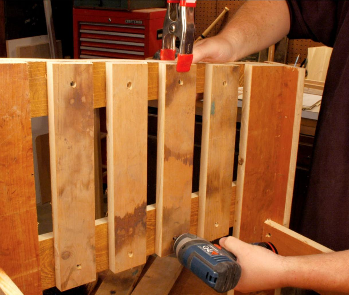
**Step 15** *A single screw in the center of each slat (top and bottom) holds things comfortably in place.*
