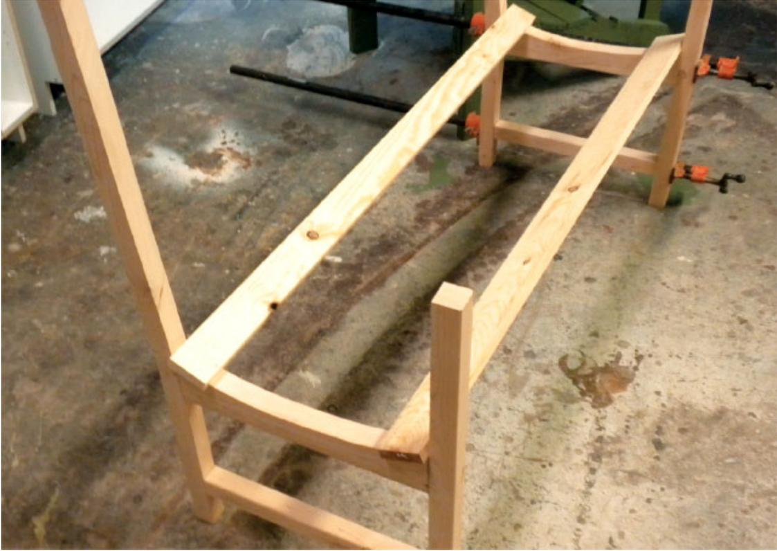
**Step Eight** *Two clamps are sufficient to ensure good, even clamping pressure. Joining the sides with the seat boards helps the project really start to look good. I tack them in place with a brad nailer and then reinforce the joint with weather-resistant screws. Spacing the slats is easy since I'd already ripped them to the width indicated in the cutting list.*
