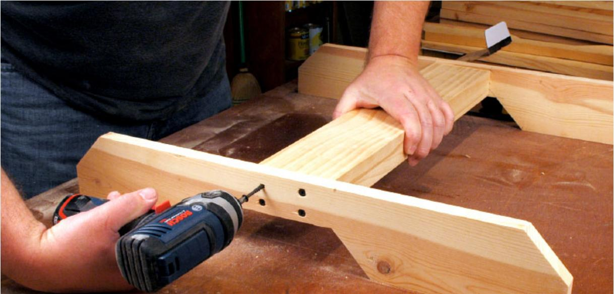
**Step Eight** I then set the base frame on my work surface and made sure it was sitting flat before screwing the second inner bracket foot in place.
