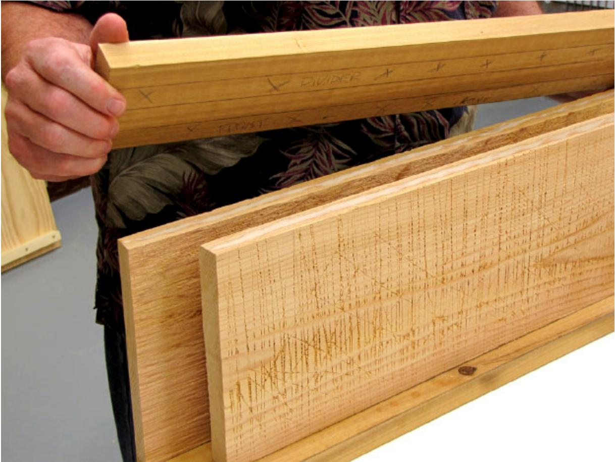
**Figure 4** *Glue and nail the sides in place.*
