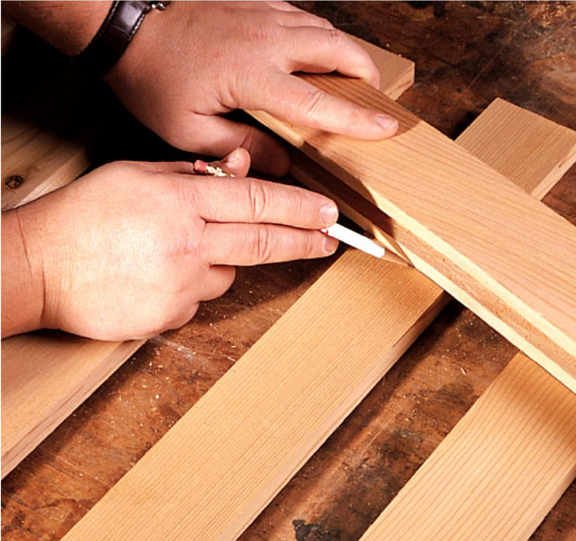
*With the miters cut on the top rail and back stiles, space the slats and use the top rail to mark the angle and length of each slat, (adding 1").*
