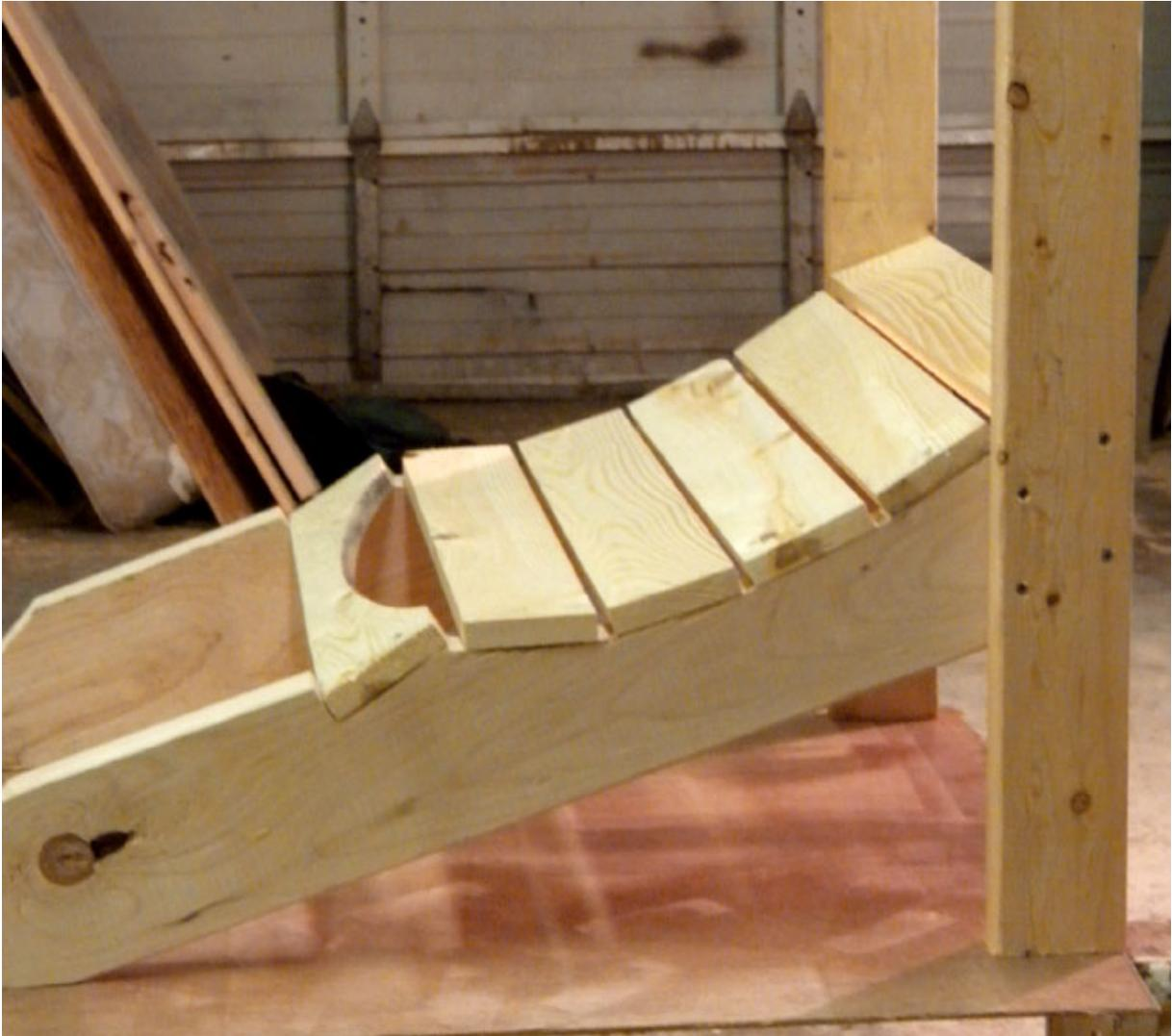
**Step Nine** *Once the lower part of the seat assembly is complete, the front legs can be attached. I left them longer than necessary at this point. I figured I could easily trim them down to a comfortable height when the time came. The legs should be bolted to the seat supports (flush to the front edge) with carriage bolts, but long screws will provide a fine temporary method of attachment.*
