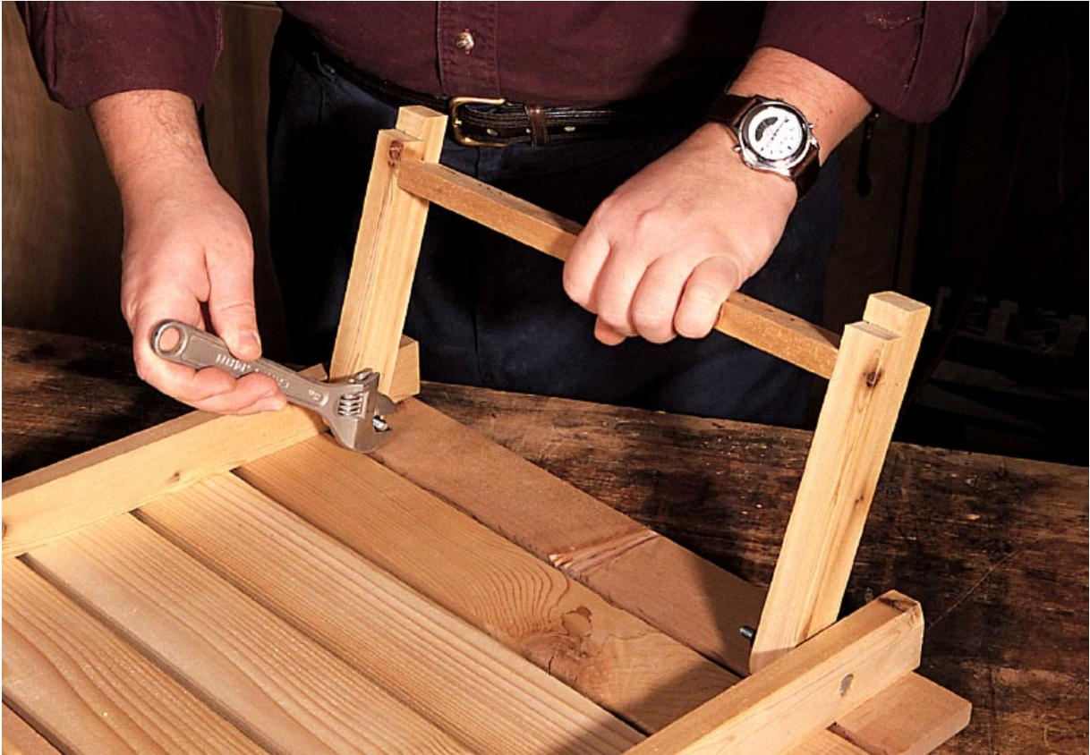
*Last, but not least, bolt the table legs in place to the table battens. Note the notches on the ends of the legs which drop into the previously cut notches to stabilize the table.*
