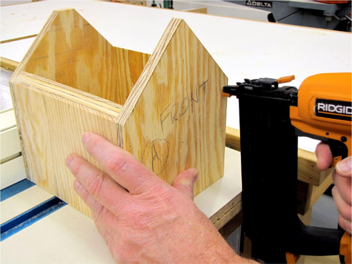
**Figure 2** Start assembly by attaching the front and back of the house to the two sides with waterproof glue and nails.
