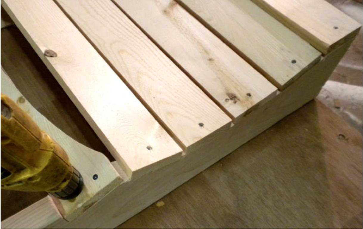
**Step Eight** Here's a helpful view of the screws into the seat slats. I suggest placing the screws as far from the outside edge as possible to prevent splitting.
