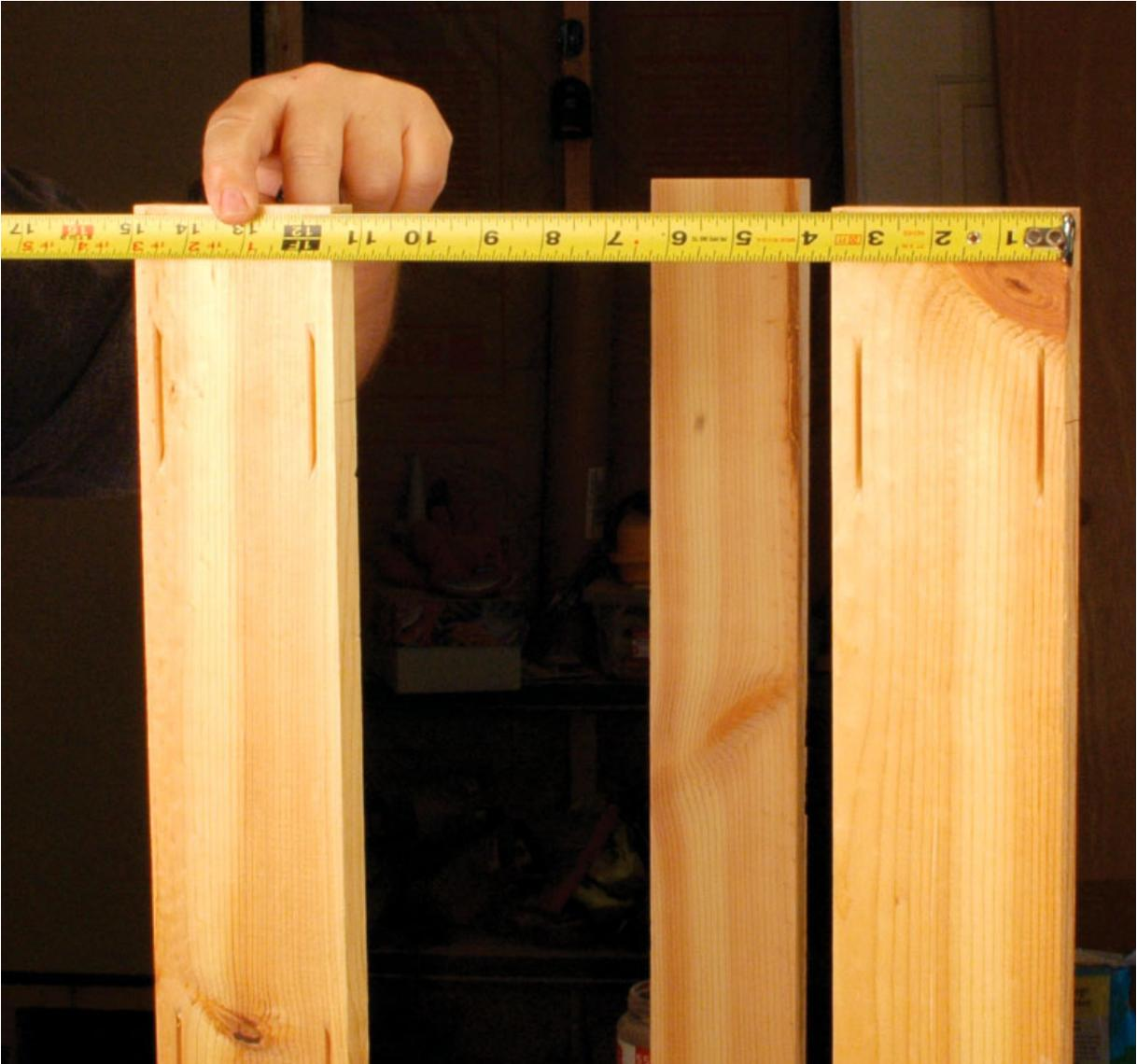
**Step 12** *I measured across the two posts down by the feet, and then made sure that the dimension was the same at the top of the posts, then put the last three screws in the bottom of that post.*
