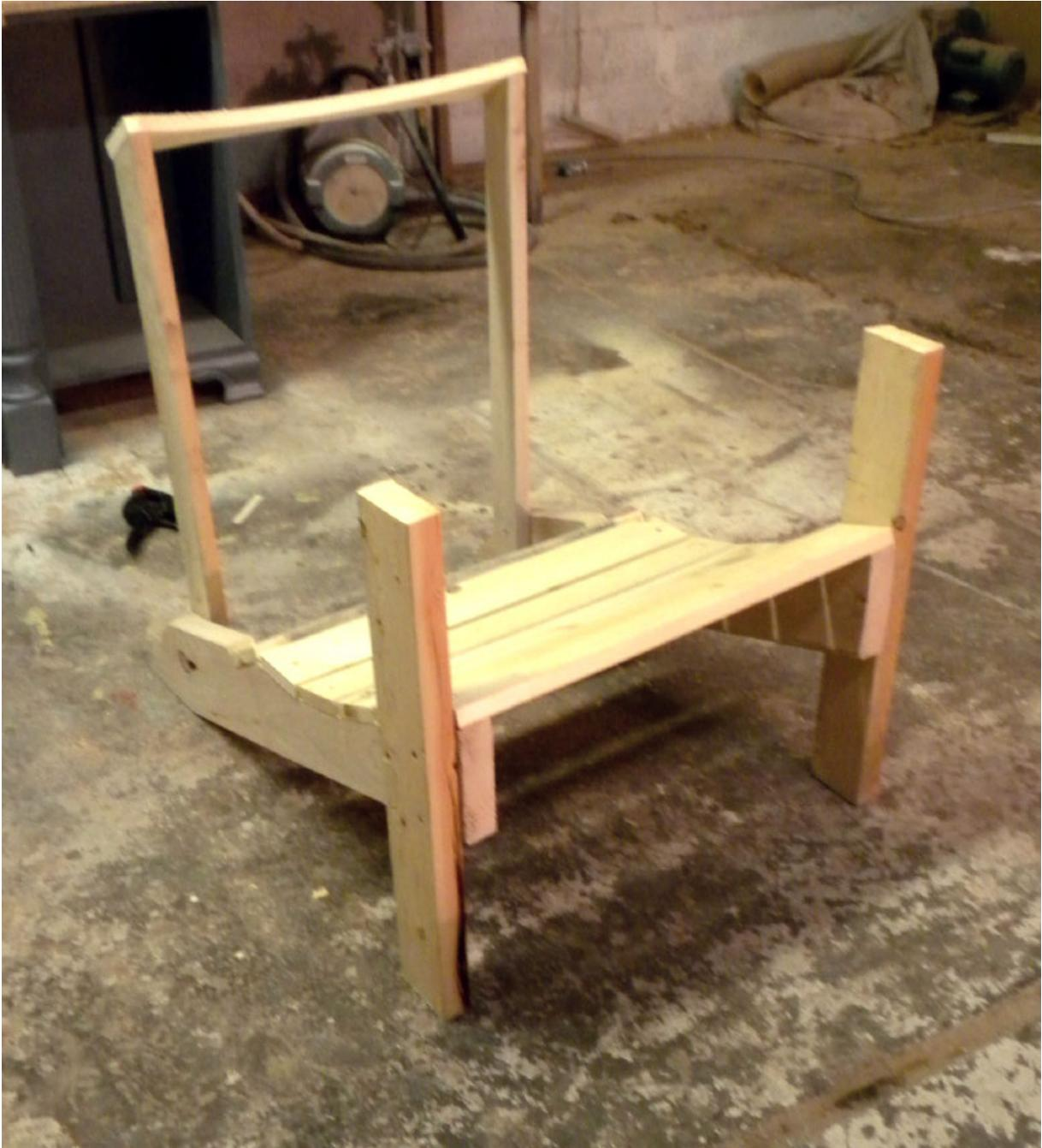
**Step 11** *I screwed the upper back support rail to the tops of the rear legs, and this set the stage for me to begin laying out the fanned back slats.*
