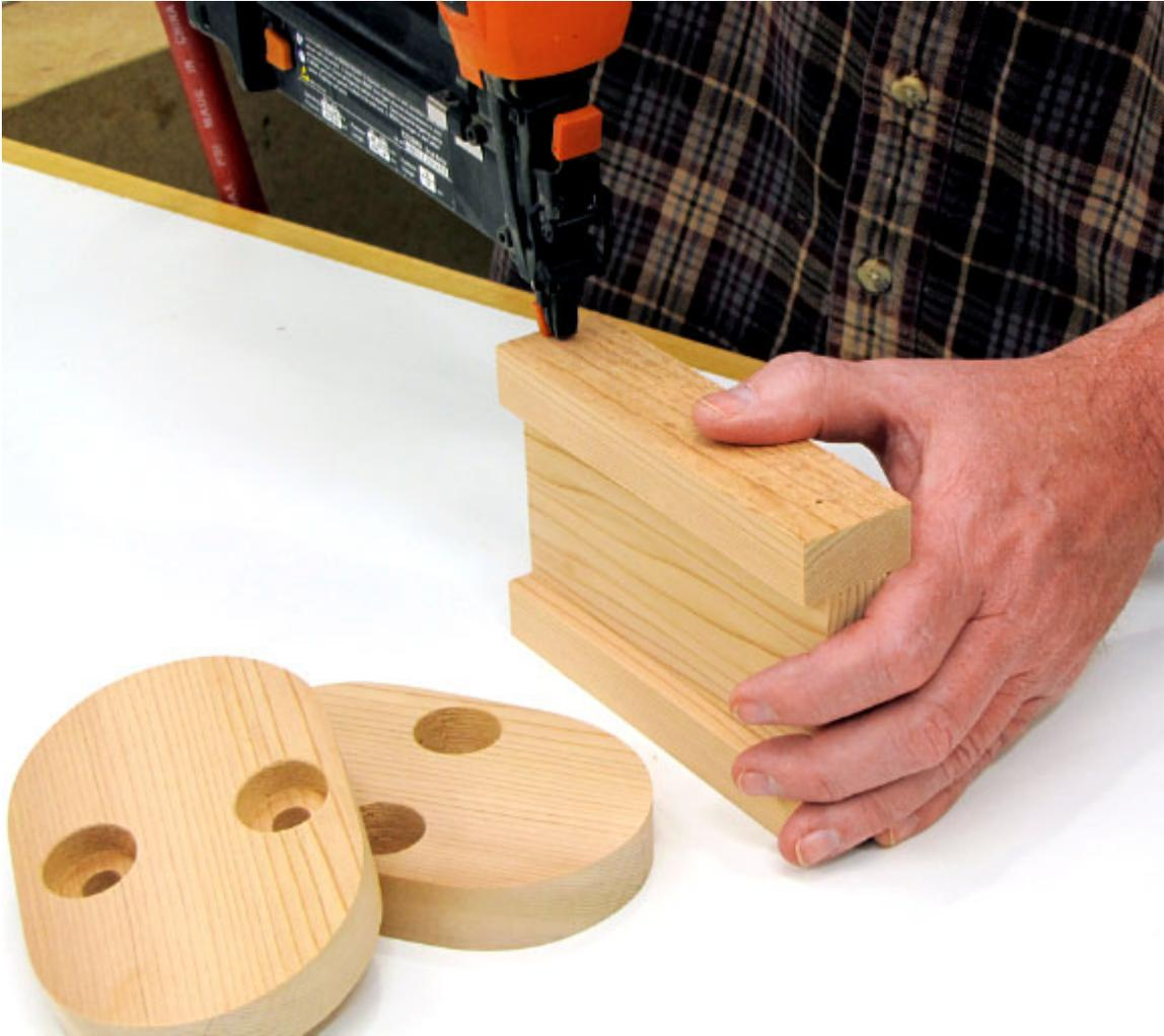
**Figure 3** *With glue and nails, attach the 1 ½" sides to the center piece.*
