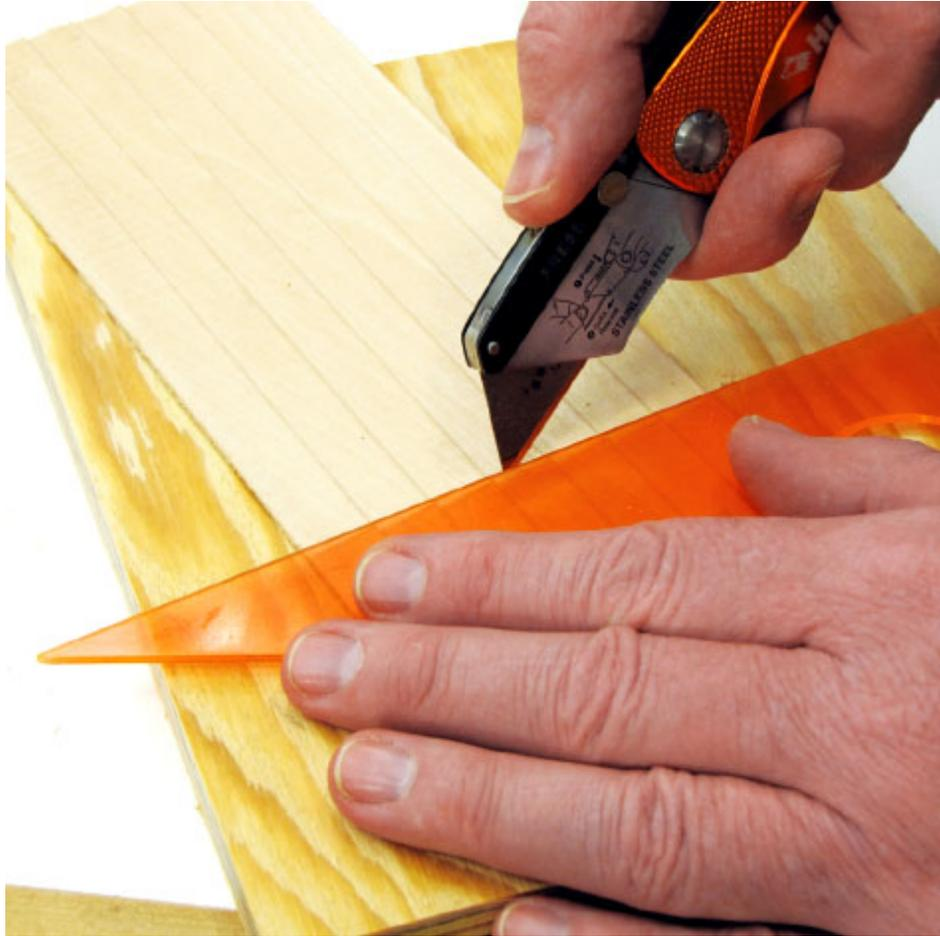
**Figure 4** *With a piece of scrap underneath, use a sharp utility knife (or a fine-cut saw) to cut your siding to size.*
