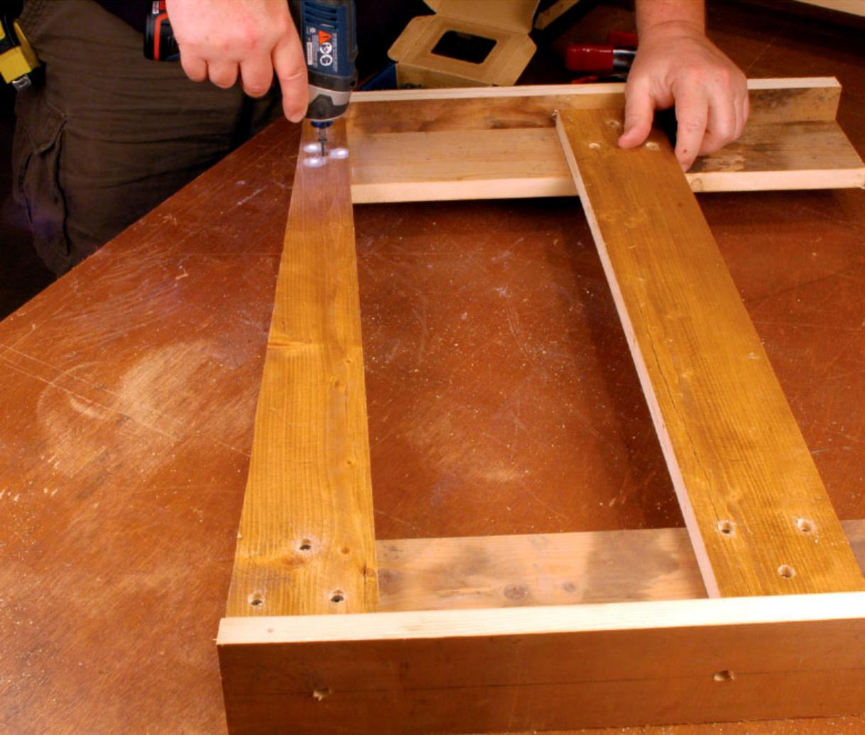
**Step 12** *Screw the upper stretchers in place to complete the leg sides.*
