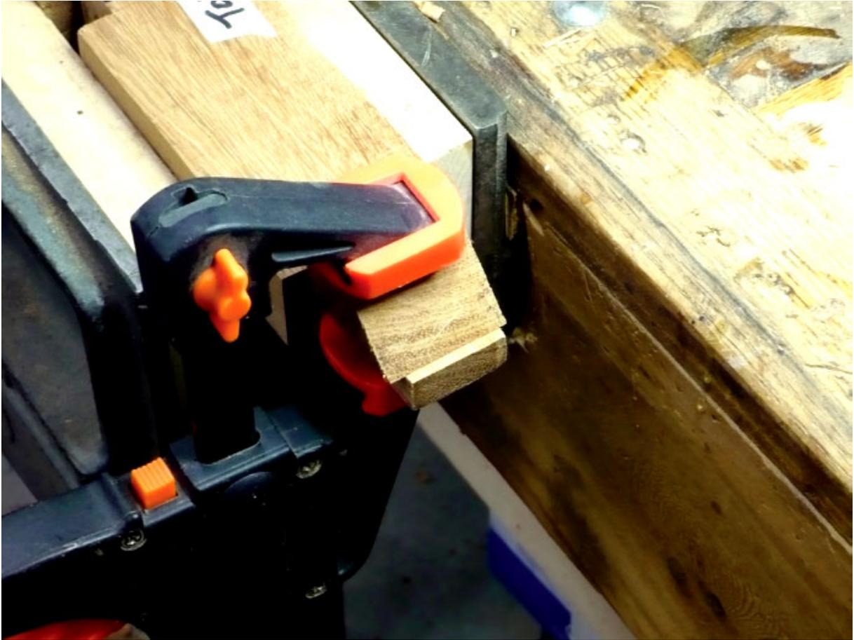
***Chamfer.*** I finished the end of each through-tenon by clamping the workpiece into my bench vise, then clamped on a jig to hand-cut the chamfers.
