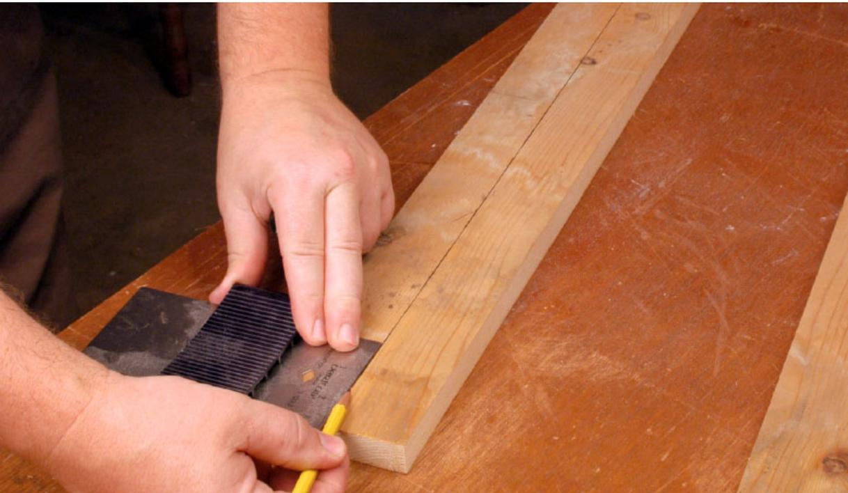
**Step Four** All four legs have the leg of the T centered on the flat of the T. Mark the center line for screws.
