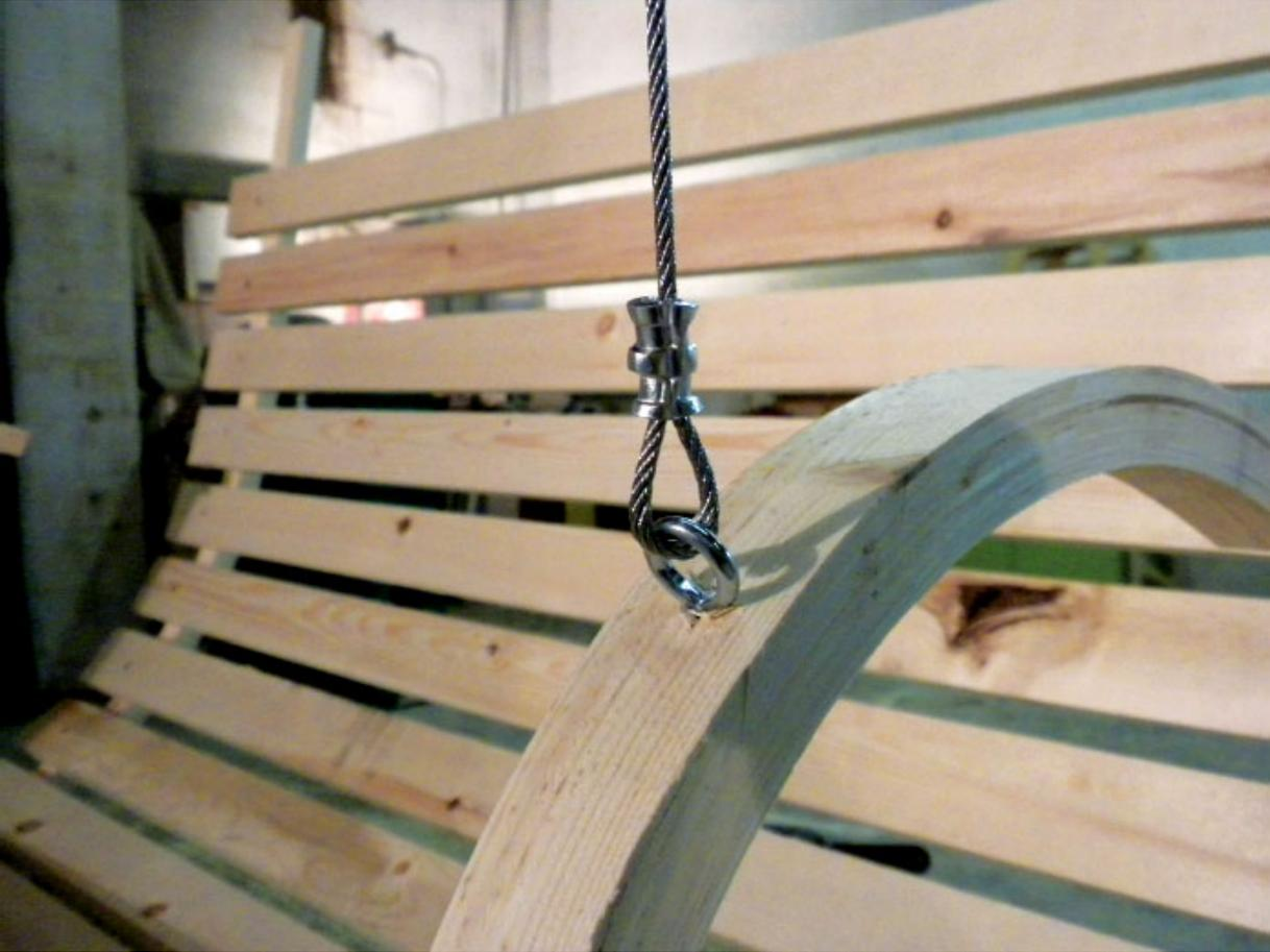
**Step 24** *I thought a cable might be a nice complement to the clean, modern design of this swing, but you could use chain or rope, too. Either way, a pair of eye hooks will need to be installed. Cable swages can be crimped using an inexpensive tool designed for the purpose. Just squeezing them in a vise is tempting, but it may not result in a strong and durable connection.*
