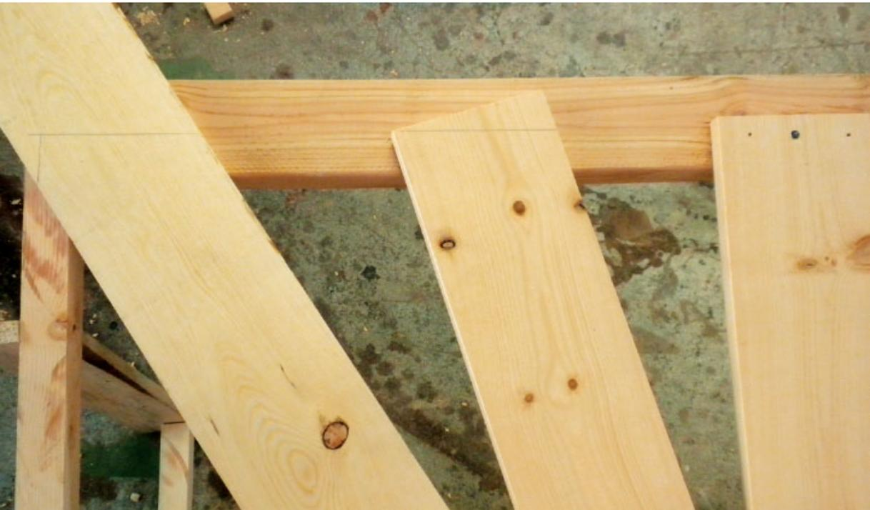
**Step 21** I also drew a line across the top. The top corner of the slat on the end needed to be trimmed to a point.
