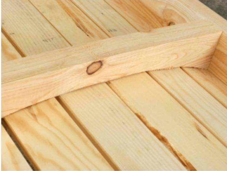
**Step 16** *When I added the remaining three strips to complete the first lamination, I found that I could set the whole thing on the floor. This freed up the form for me to begin laying out the second side.*
