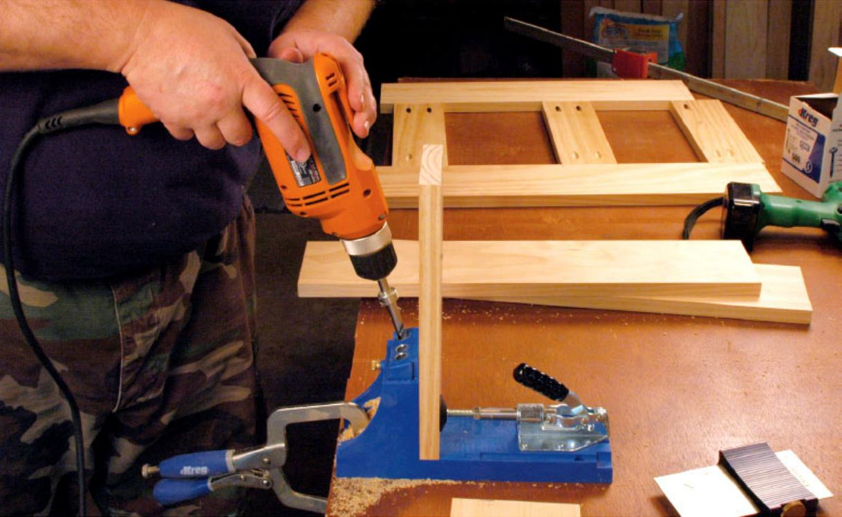
**Step Two** My pocket screw jig makes quick work of the holes drilled in only the horizontal parts.
