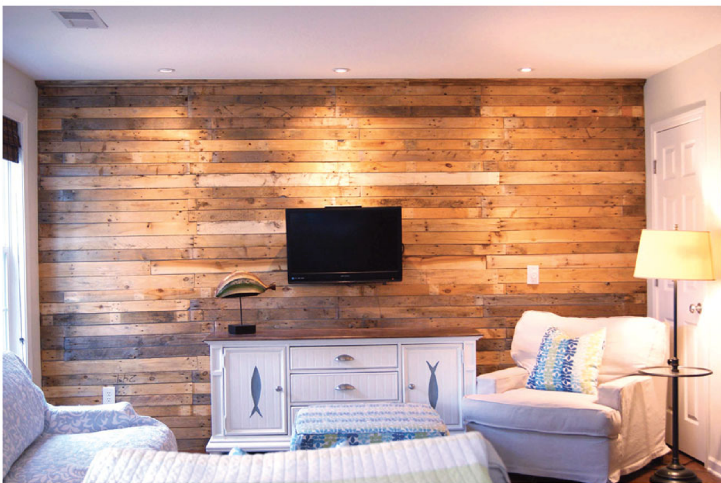
For an accent wall like this one, you may need up to 25 pallets. Construction adhesive and a nail gun attached the pallets, and the TV is anchored to a wall stud.
