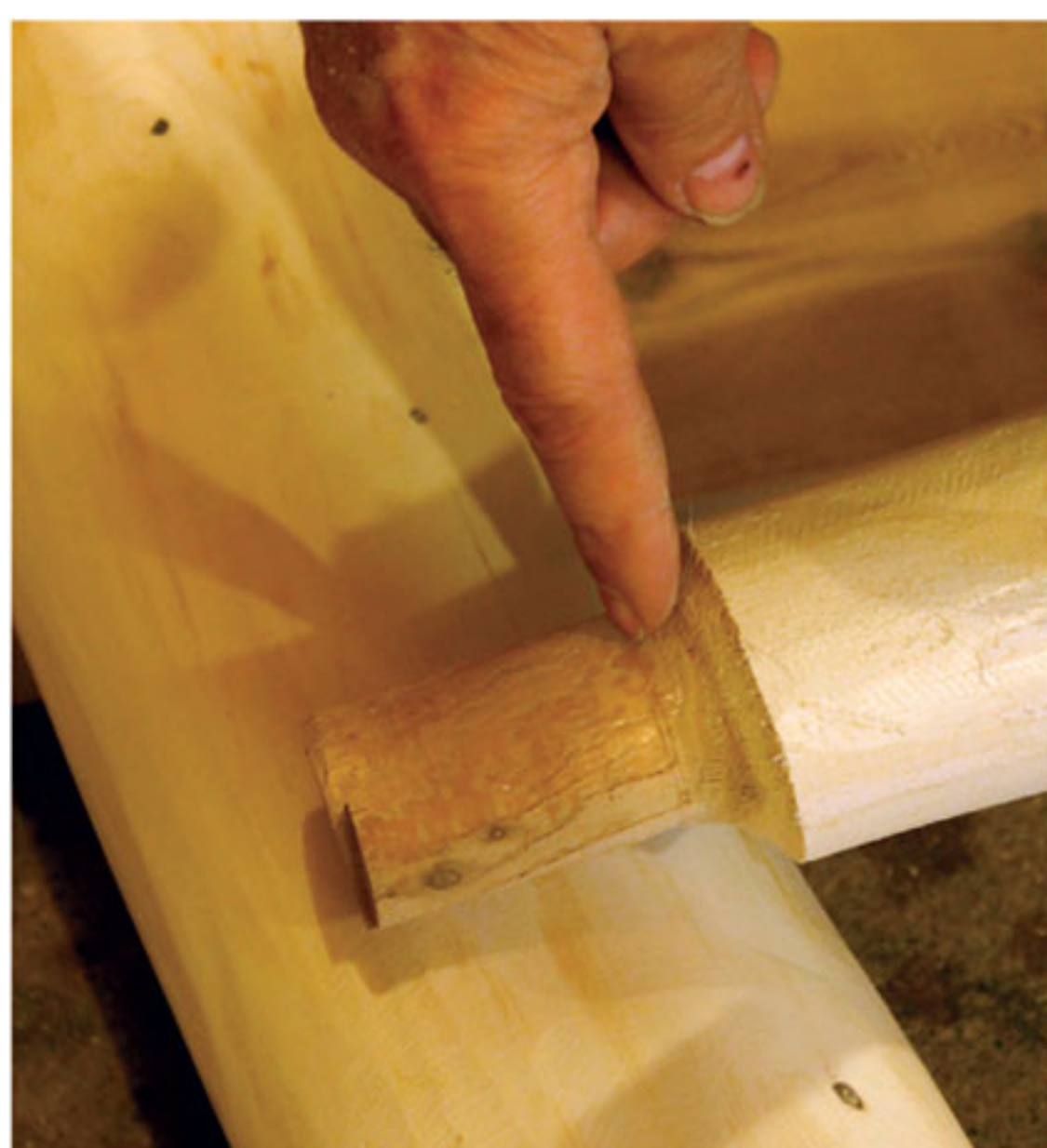
All tenons are 1½ inches around and 2 inches long.
