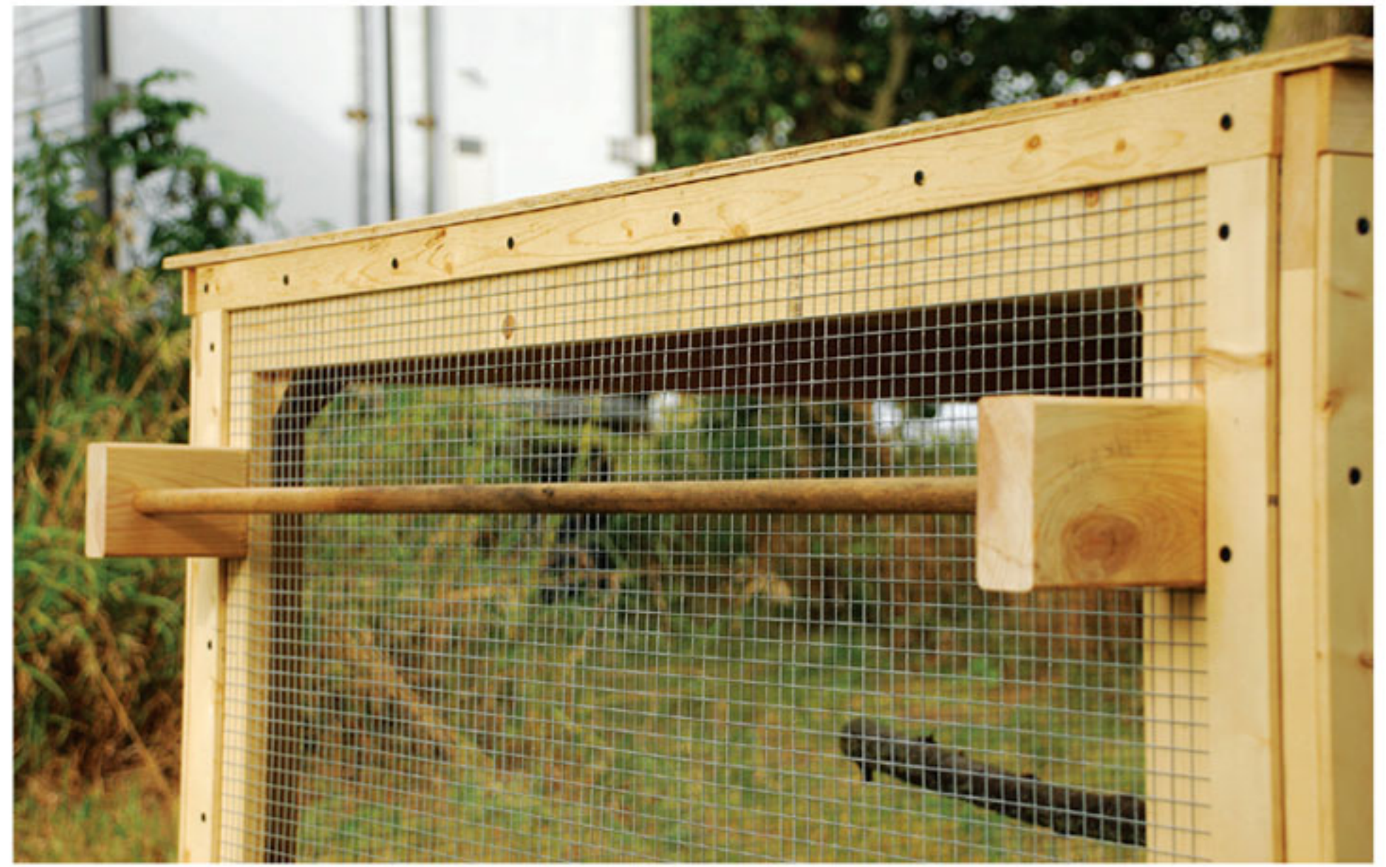
The end blocks of the dowel handle will be attached from the inside with 3-inch screws, and you can position the handle to accommodate varying heights, whatever is most comfortable.
