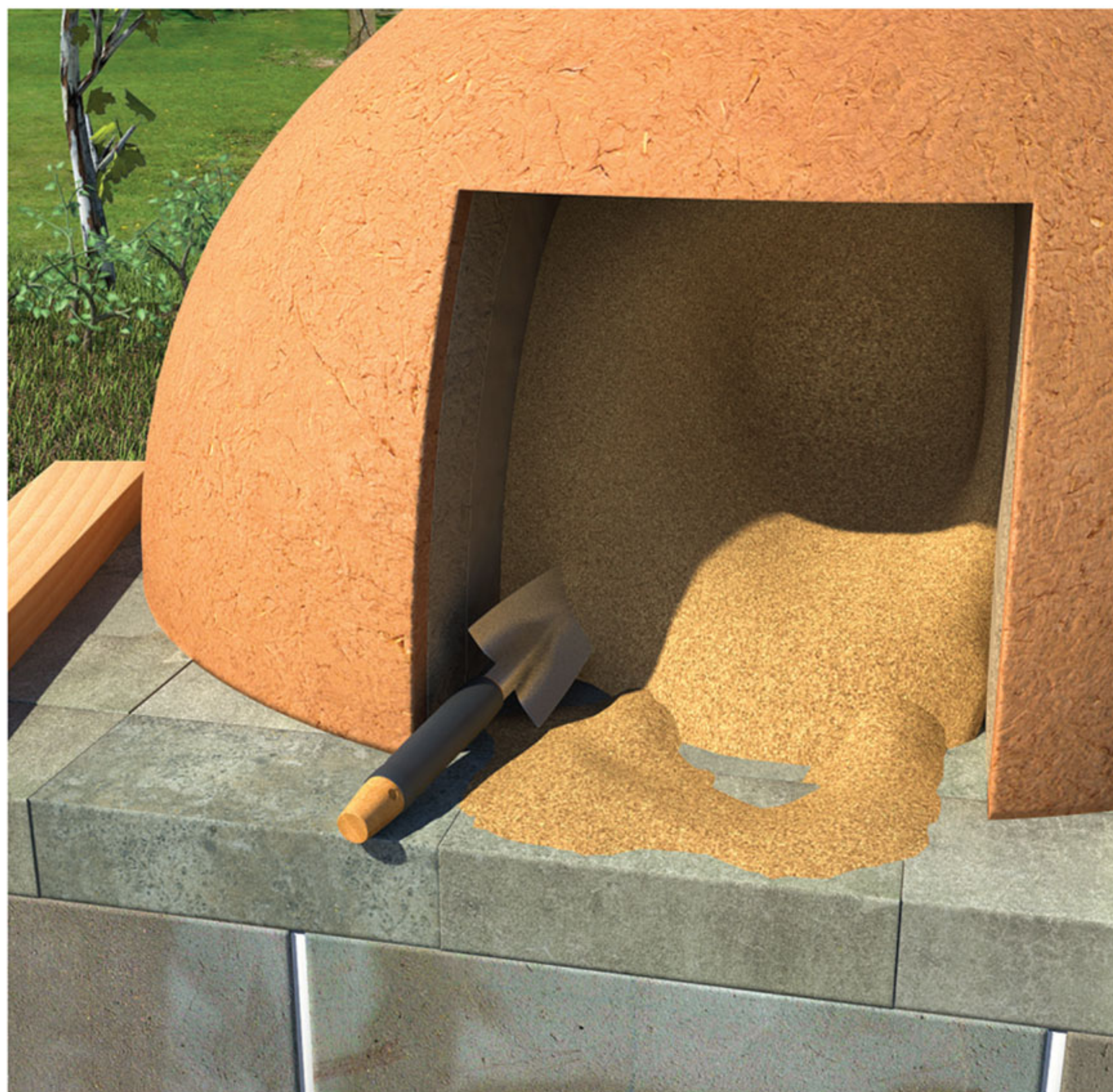
FIGURE 4. After the door is cut, carefully remove the sand, and gently scrape or brush it from the interior.
