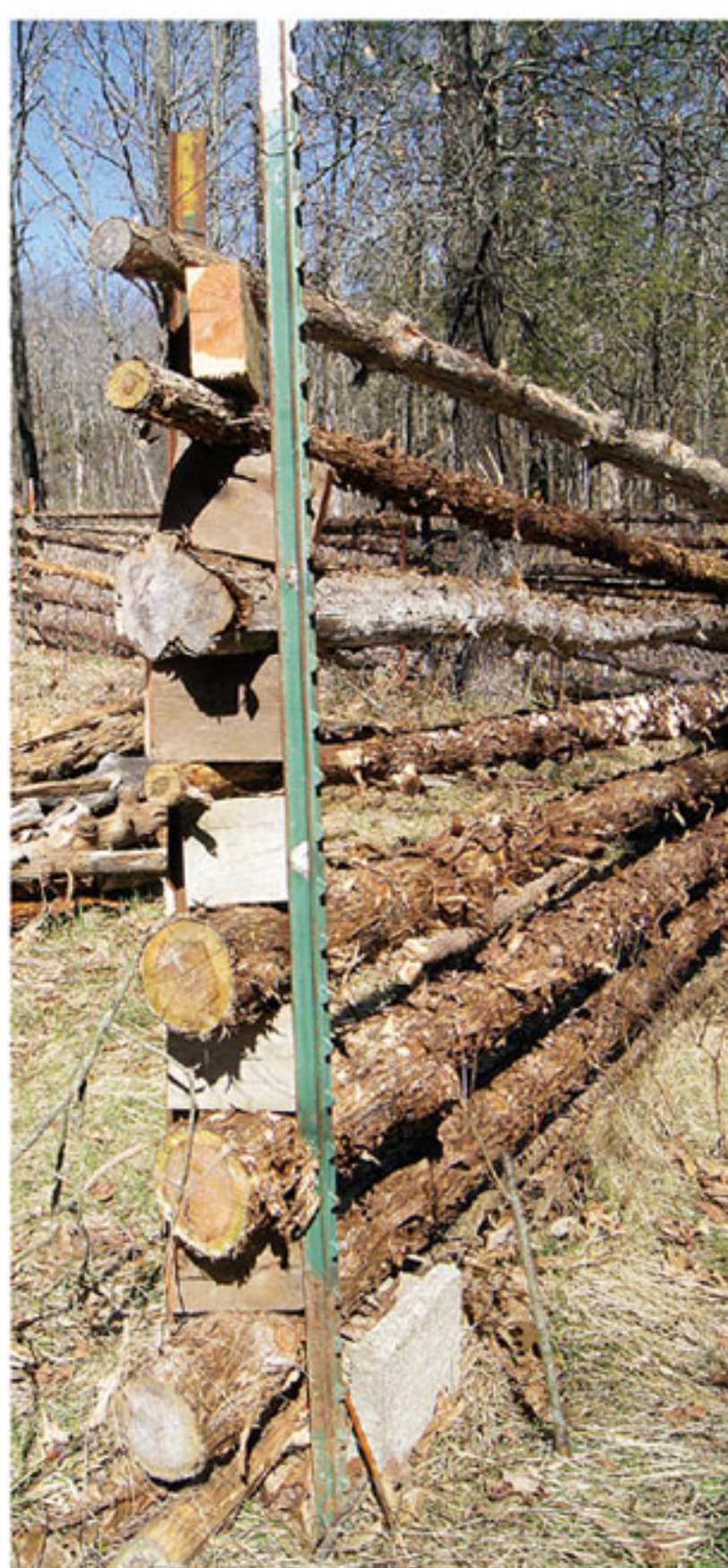
Two T-posts keep this homestead rail fence straight and secure.
