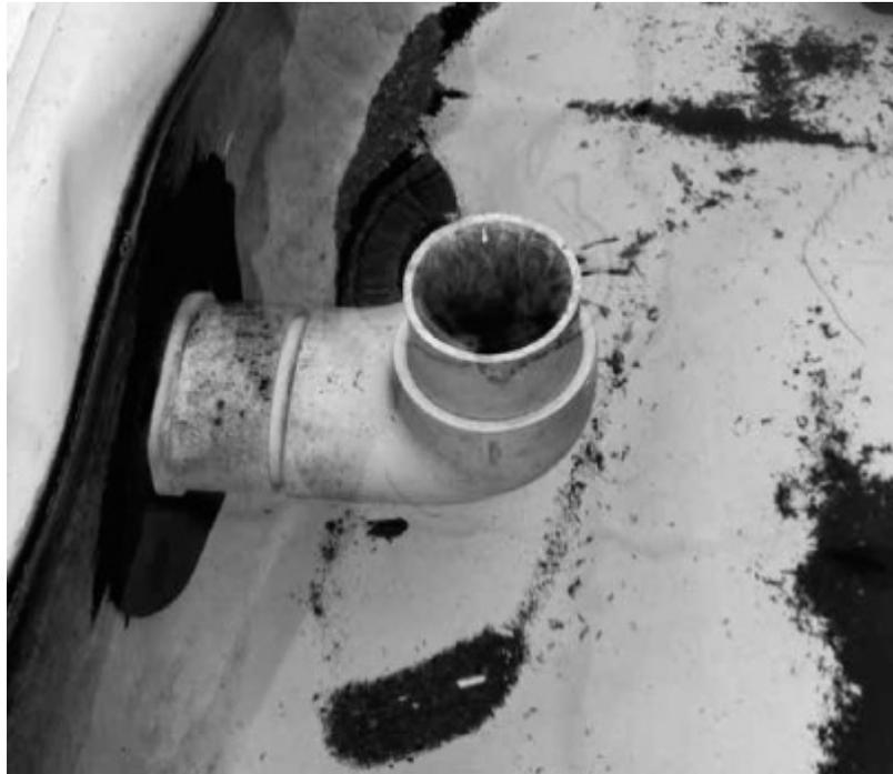
*Trough drain standpipe.*
