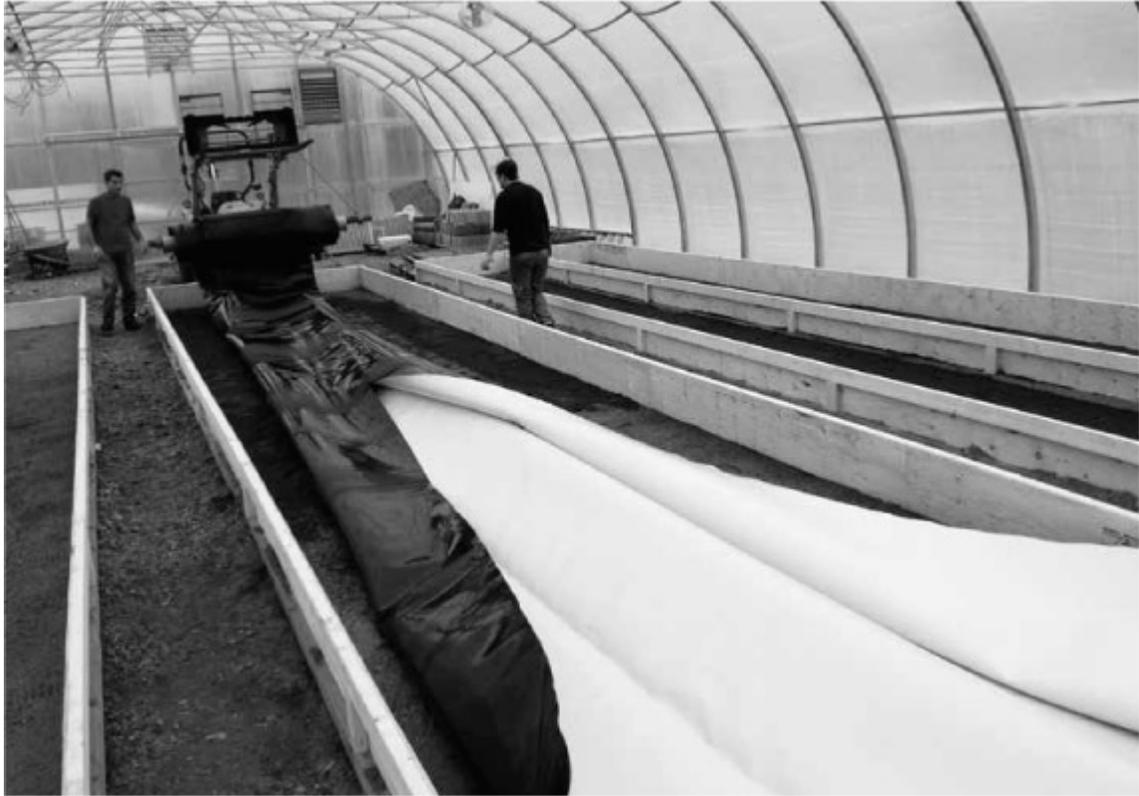
*Rolling out the LDPE for liner installation.*
