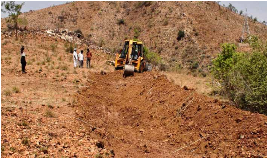
FIGURE 7.3. A backhoe making the initial excavation for the swales.
