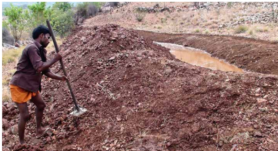
FIGURE 7.5. A worker compacting a swale's spillway.
