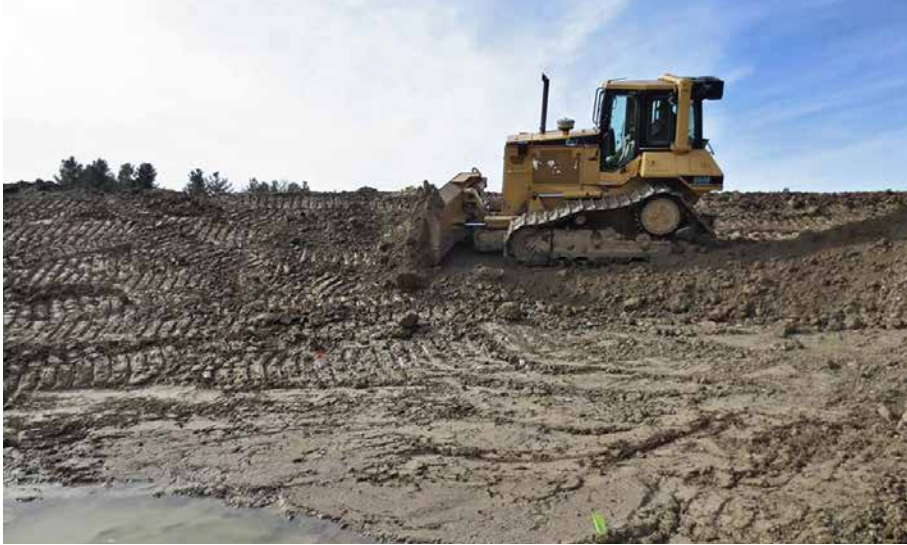
FIGURE 8.9. Good clay being spread across the inside of the dam wall.
