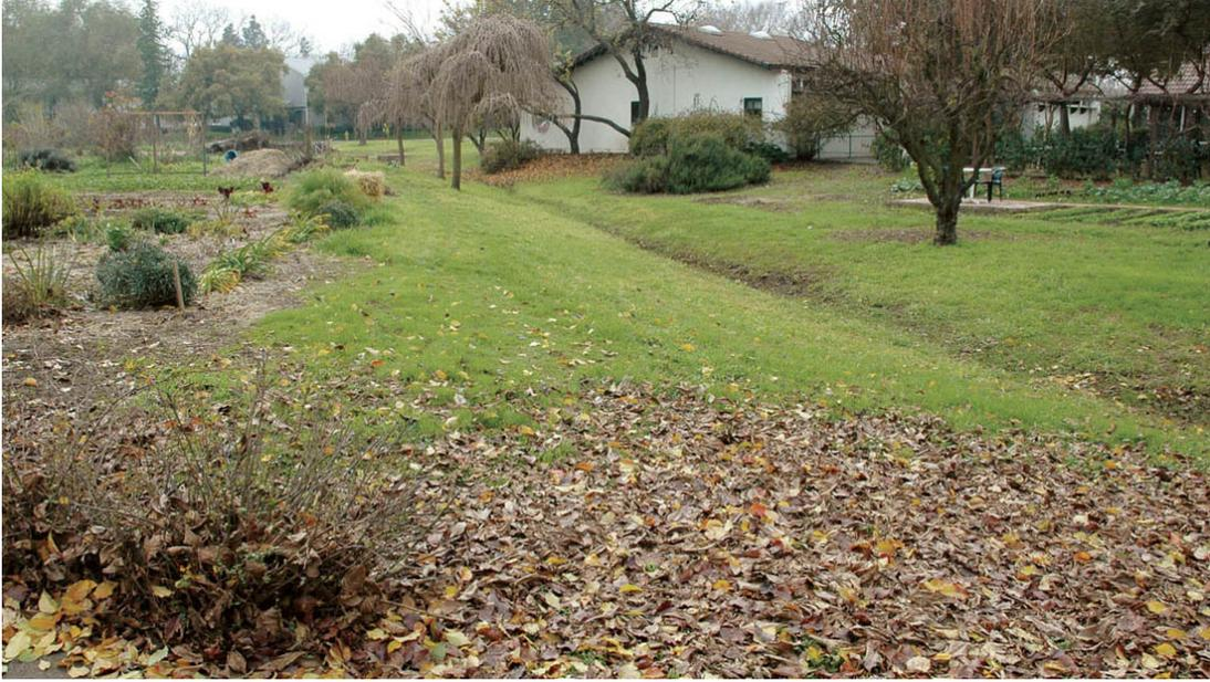
*ABOVE: At a time when most housing developments funneled stormwater into the town sewer system, the Village Homes community was designed with a network of drainage channels to keep stormwater on-site and allow it to infiltrate back into the soil.*
