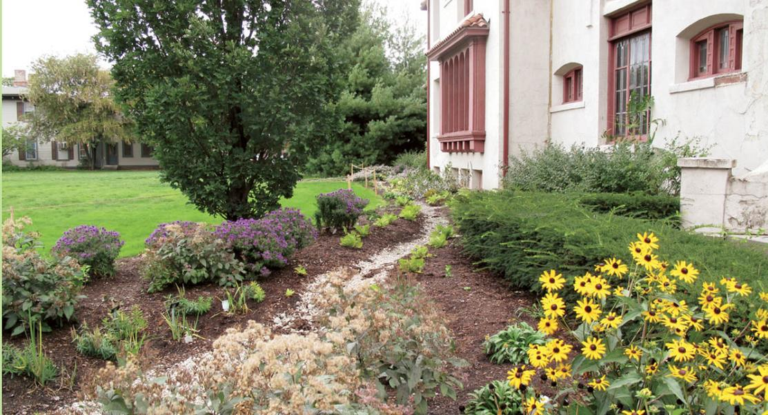
*ABOVE: At the core of this rain garden — which my firm designed and installed for the Springfield Museums in Springfield, Massachusetts — is a conveyance swale, which catches rainwater from the roof, directs it away from the building, and allows it to infiltrate into the surrounding soil.*
