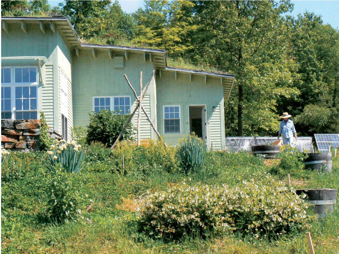
*ABOVE: The green roof cottage at Wildside is positioned on a south-facing slope — perfect for active and passive solar. The green roof insulates the roof and lengthens its life span. Gardens wrap around the cottage to the south for easy harvesting access and the solar hot water and electric systems are positioned out of the way to the north of the cottage.*
