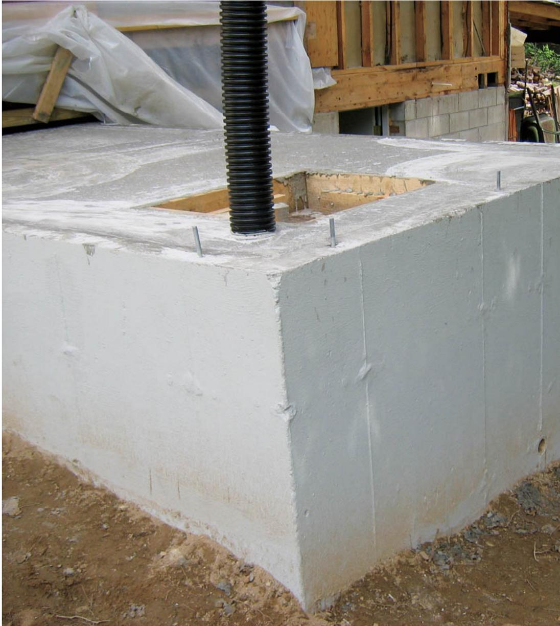
*ABOVE: When we built an addition onto our house, we incorporated a cistern into the poured foundation to capture and store rainwater.*
