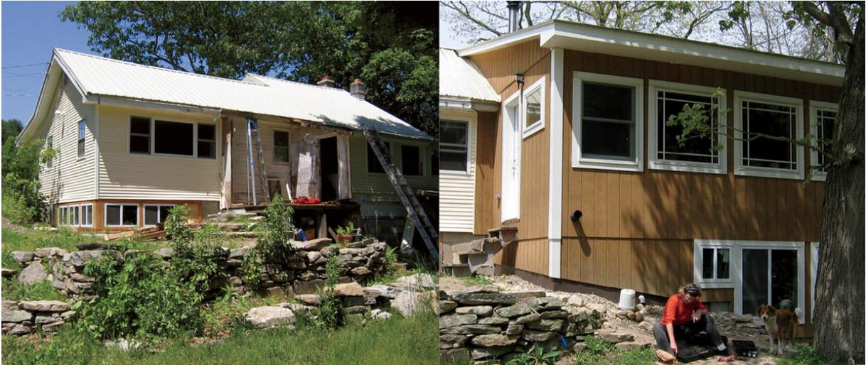
*ABOVE: Removing the uninsulated, south-facing enclosed porch and replacing it with an insulated, window-filled space allowed sunlight to enter our living space and made the whole house warmer.*
