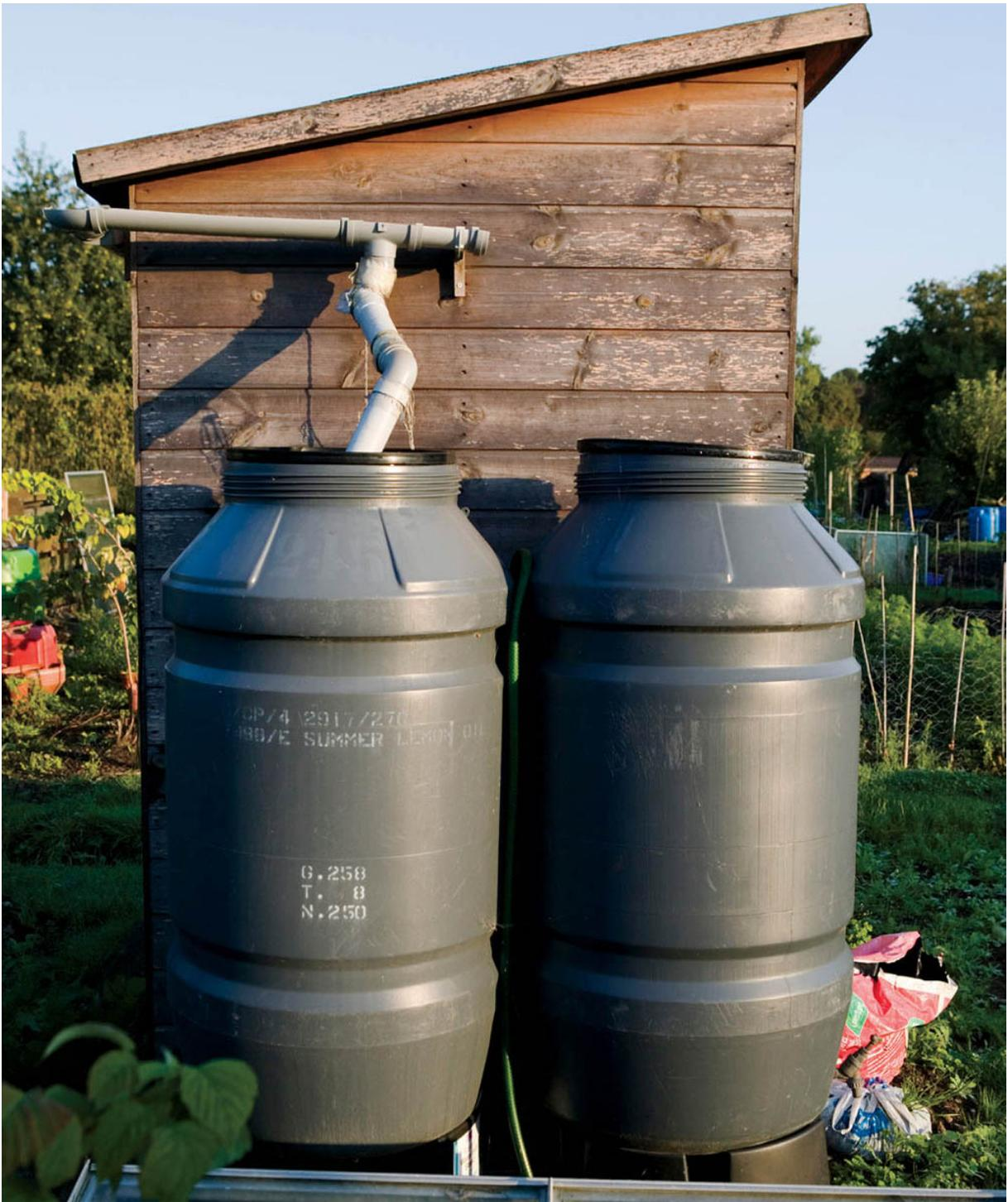
*ABOVE: Using rain barrels to capture water for irrigation is a simple way to cut down on groundwater usage.*
