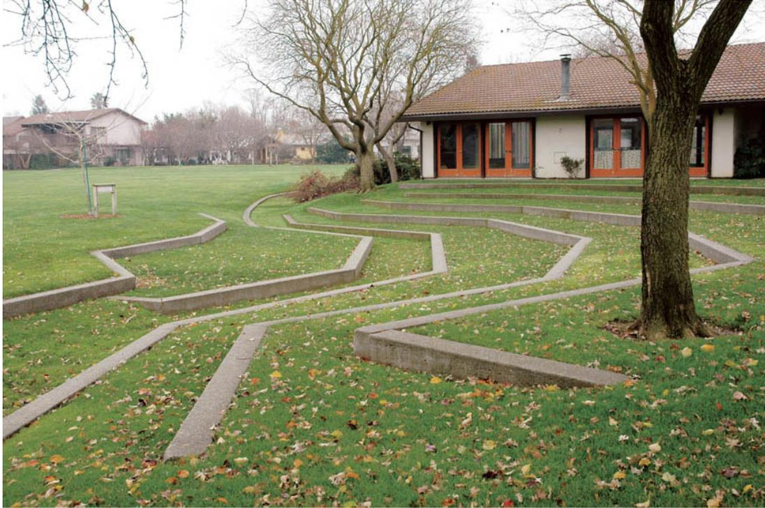
*ABOVE: A stormwater retention basin becomes an outdoor amphitheater during dry times.*
