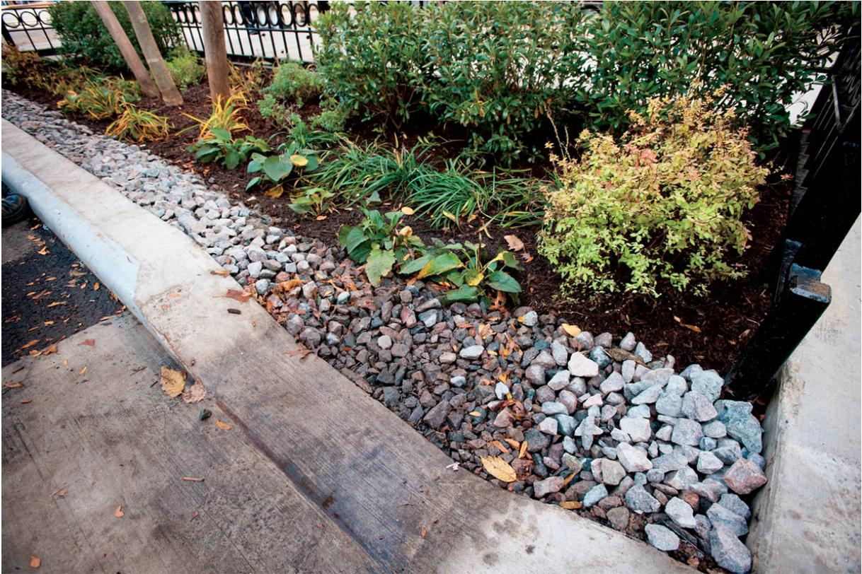
*ABOVE: Using strategically placed curb cuts and stormwater runoff basins helps keep rainwater on-site, where it can infiltrate back into the ground instead of flowing into streams and rivers (often carrying pollutants with it).*
