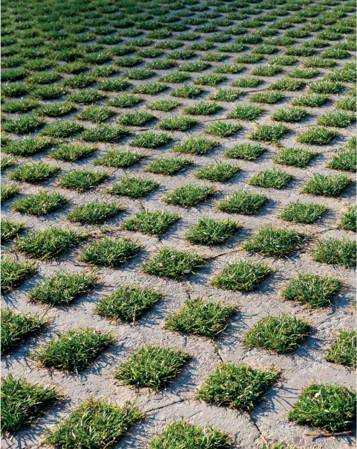
ABOVE: *Using permeable pavement instead of solid blacktop or cement is one way to make cities more livable. It allows rainwater to infiltrate into the soil, keeping it on-site instead of flowing into local waterways.*
