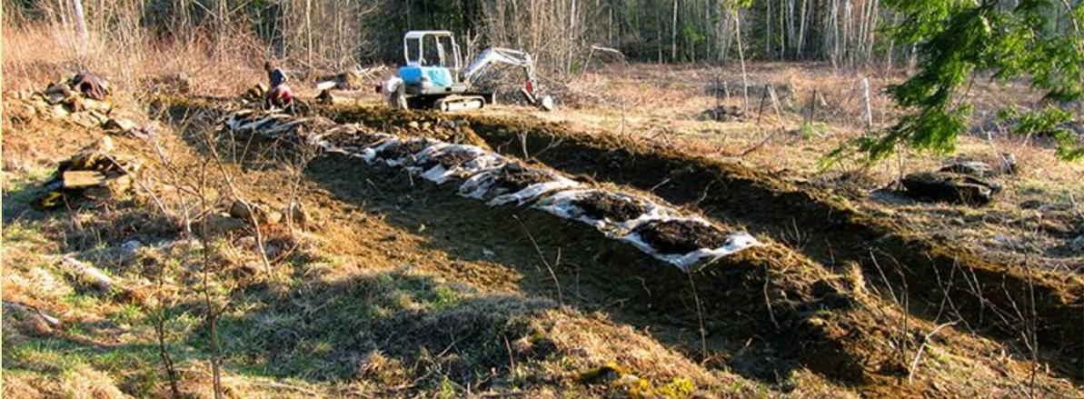
Swale construction on a relatively steep (approximately 35 percent) grade in early spring at the WSRF. Note that swales are seeded and planted immediately.
