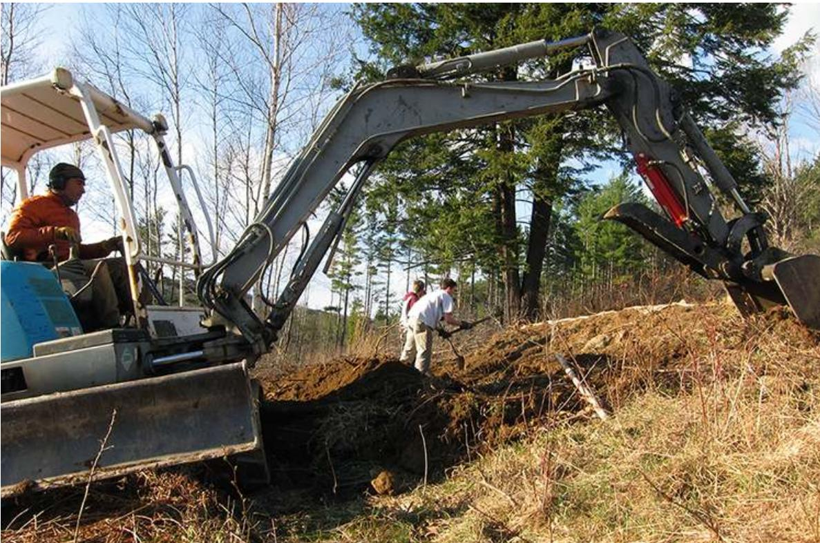
The author constructing swales with an 8,500-pound compact excavator—the most useful small earthworking tool for swales and paddies at this scale
