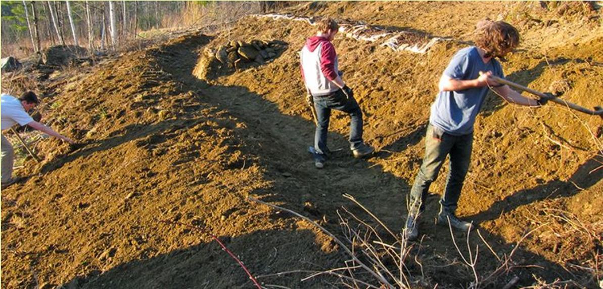
Hand-working swales to smooth the grade out after machine forming them
