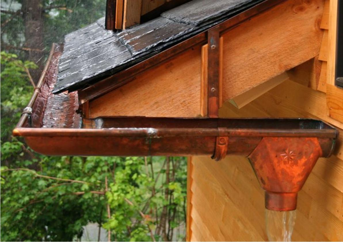
This copper-gutter “drop” connects to a copper downspout that feeds a pond and can be connected to drinking-water storage. Slate and copper combine to offer completely potable water from our roof and also last a century or two.
