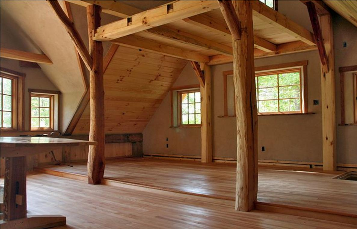
The Whole Systems Design studio before move-in, with roughly 95 percent of the materials by volume used in construction sourced within seventy-five miles of the site and more than 75 percent of the wood sourced on-site.
