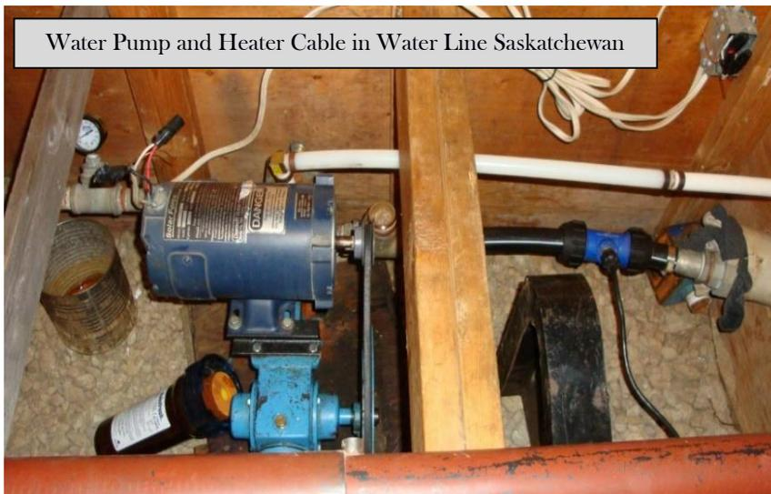
Water Pump and Heater Cable in Water Line Saskatchewan
