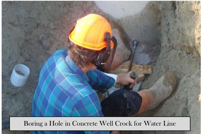
Boring a Hole in Concrete Well Crock for Water Line
