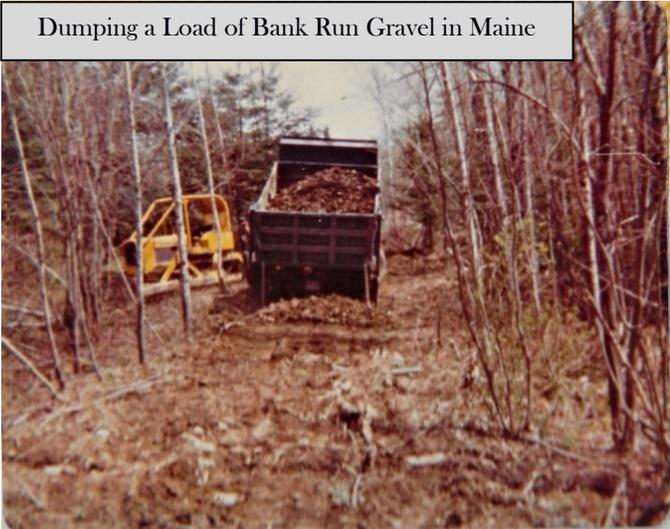
I bought “bank run gravel” from the local contractor. Bank run gravel is unprocessed, right out of the ground material containing small boulders, gravel and sand. In wet ground, you want some big material (boulders and rock) to form a good solid base. Then gravel on top to create a relatively smooth, drivable surface.
