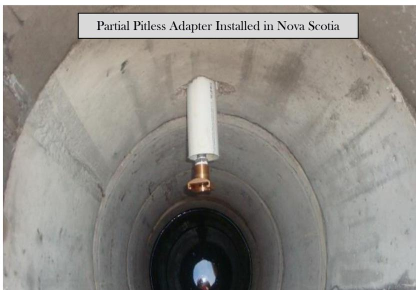
Partial Pitless Adapter Installed in Nova Scotia
