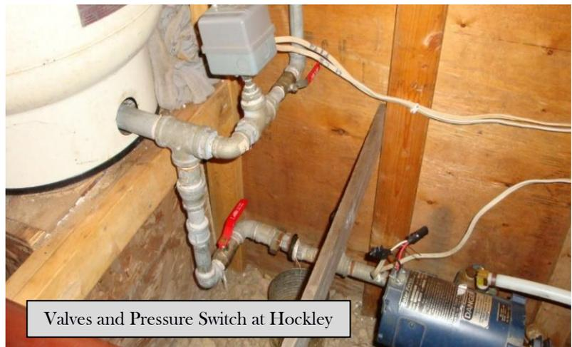
Valves and Pressure Switch at Hockley
