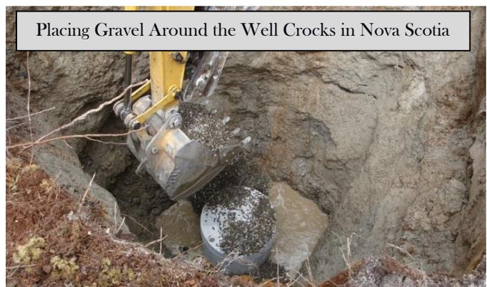
Placing Gravel Around the Well Cocks in Nova Scotia
