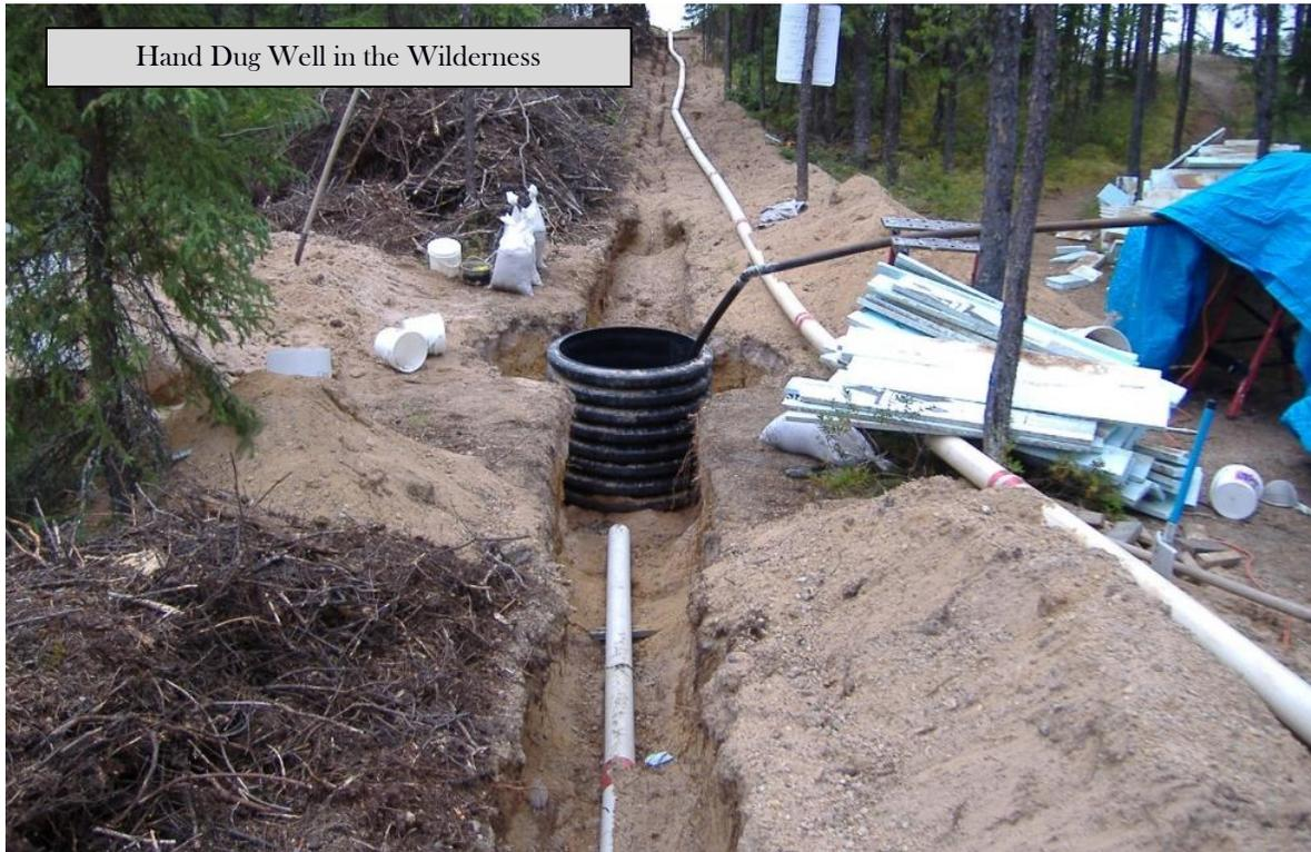
That dug well was in pure sand. If you've ever been to the beach and dug a hole in the sand, you know it's not long before the hole fills with water and the sides collapse. I came up with a way to deal with that problem though.
