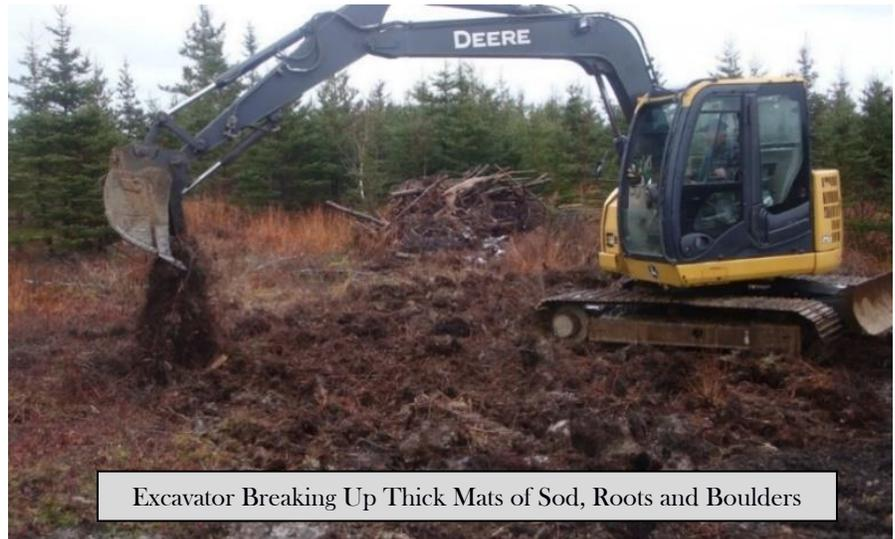
Excavator Breaking Up Thick Mats of Sod, Roots and Boulders
