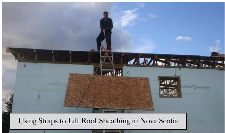
Using Straps to Lift Roof Sheathing in Nova Scotia
