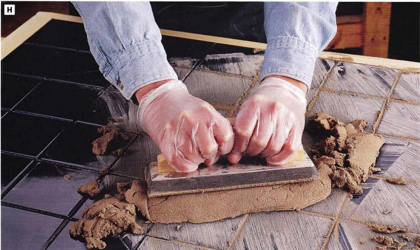
**PHOTO H:** Press grout into the gaps between the tiles using a grout float. Work diagonally across the surface, pulling the float toward you as you go. Working diagonally helps to minimize the chances of accidentally pulling grout out of the gaps you've already filled.
