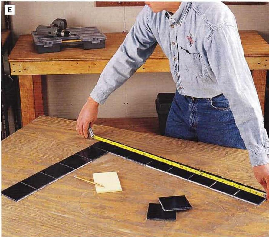
**PHOTO E:** Arrange rows of tiles to determine the length and width of the tile top. *Note: You may need to space the tiles to allow for grout lines if your tiles don't have self-spacing nubs on the edges.* The overall dimensions will establish the size of the plywood subtop.
