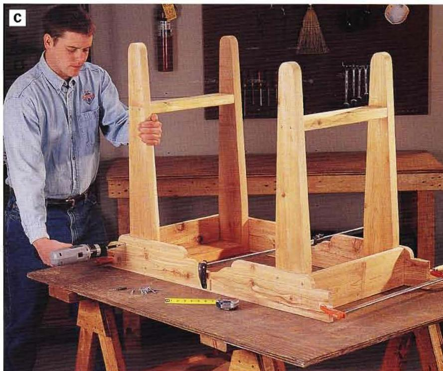
PHOTO C: Attach the end aprons to the legs, then turn the leg assemblies upside down and fasten the side aprons in place. Hold the parts in position with clamps while you drive the screws.
