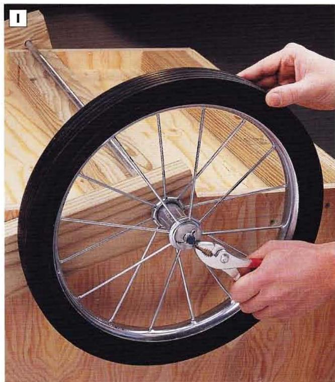
**PHOTO I:** Install the axle, washers and wheels on the cart. Slip cotter pins through the holes on each end of the axle, and secure the wheels by bending the ends of the cotter pins around the axle.
