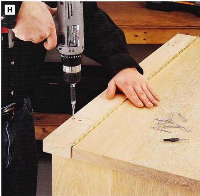
**PHOTO H:** Fasten the seat assembly to the bench, driving countersunk wood screws in the areas on the fixed seat slat that will be covered by the back supports. Screw into the upper long cleats and back slats.
