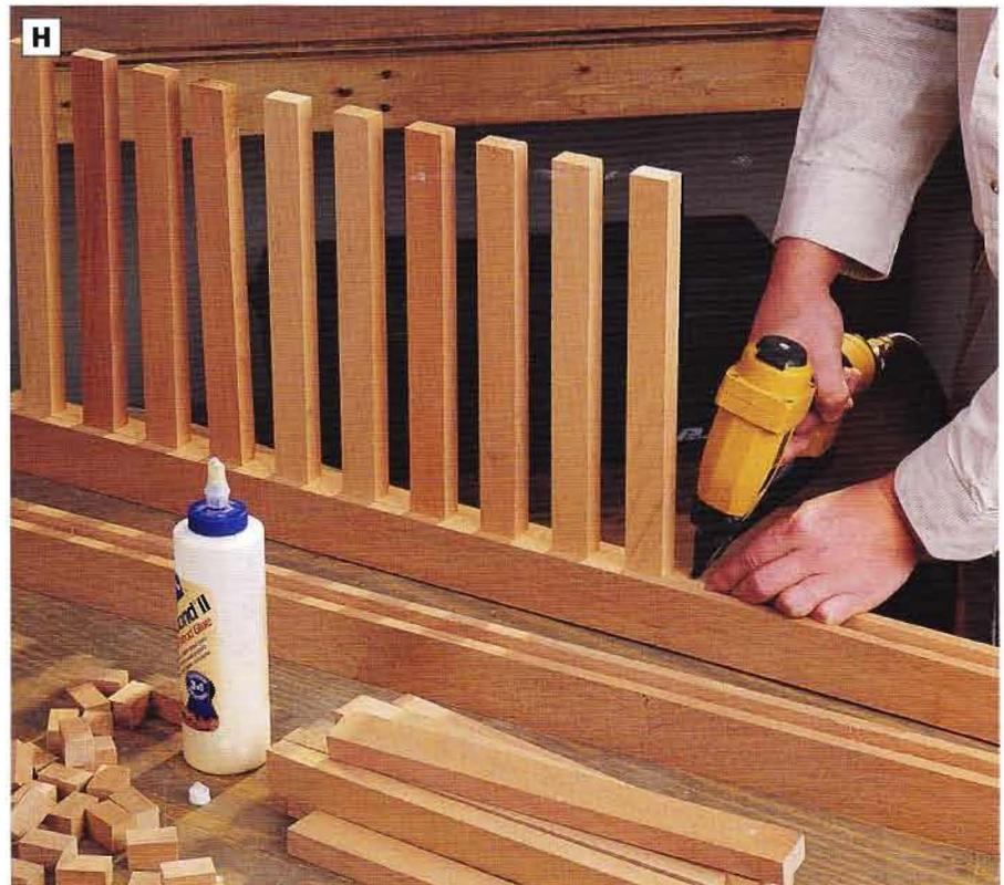
**PHOTO H:** Locate the position of the center seat slat in the bottom rail. Working from the middle toward each end, secure the slats and short spacers in the bottom rail with glue. Nail the spacers in place. We used a pneumatic nail gun and pin nails.
