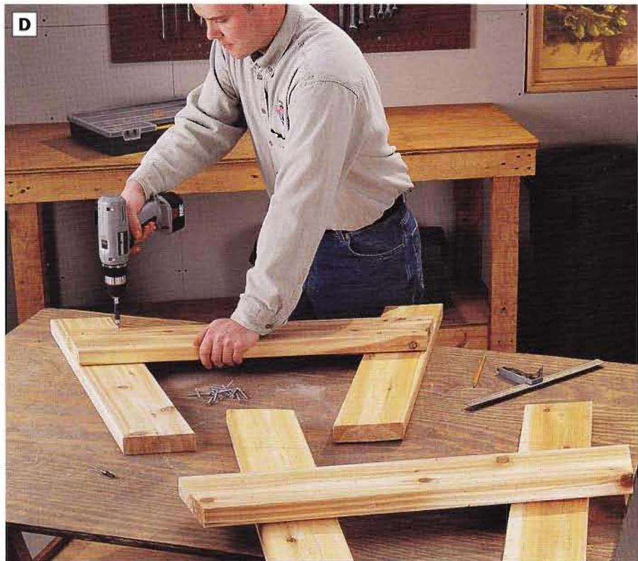
**PHOTO D:** Cut the legs and leg braces to size, and cut the ends of the parts at 75° angles. Use the *Table End View* drawing, page 57, as a reference for cutting the parts. Then construct the two table leg assemblies by fastening each leg brace to a pair of legs with deck screws.
