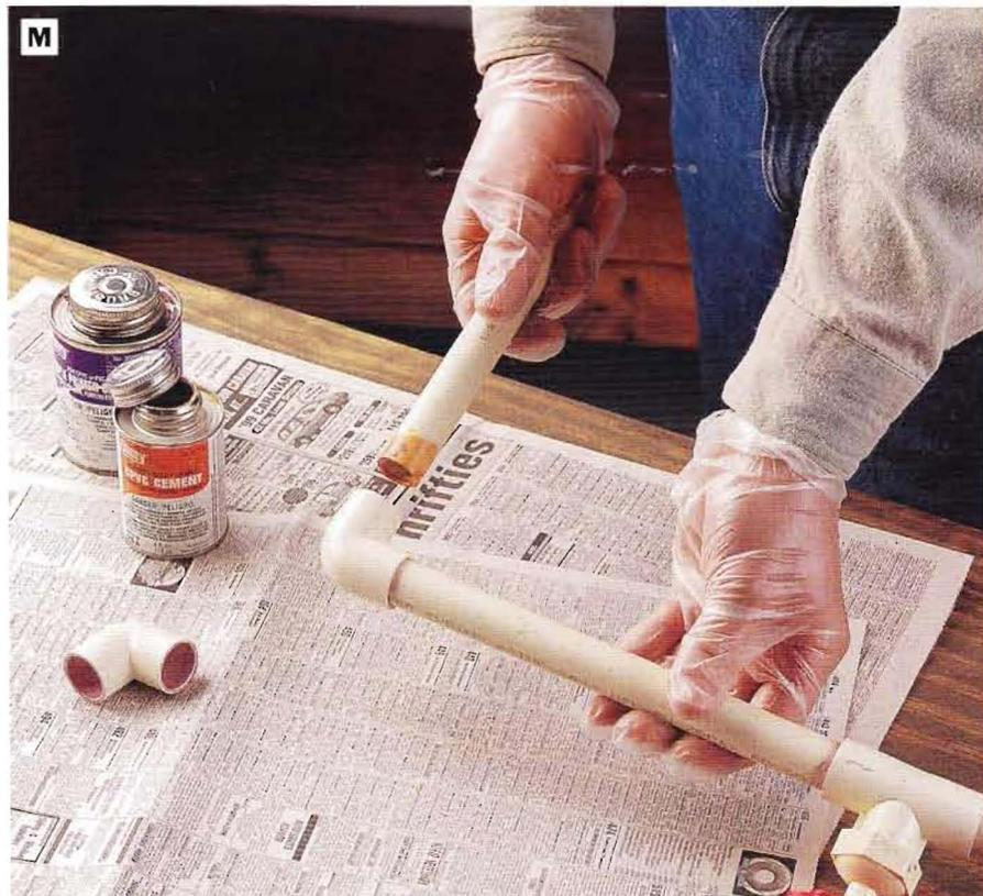
**PHOTO M:** Cut the straight pipe sections to length and dry-assemble the entire plumbing unit to check its fit on the potting bench. Then disassemble the PVC, prime the mating parts of each joint, and bond the PVC together with CPVC cement. Wear gloves when bonding the parts.
