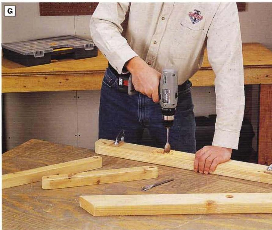
**PHOTO G:** Bore a 1-in.-dia. hole through each back rail for the back rest dowel and a  $\frac{3}{8}$ -in.-deep counterbore for the heads and washers of the adjustment brace pivot bolts.
