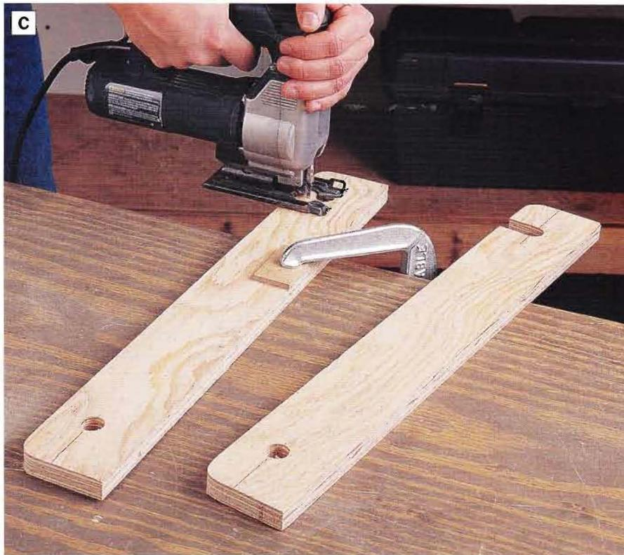
**PHOTO C:** Connect the lock dowel hole with straight lines to the edge of each stretcher, forming the lock dowel slots. Clamp the legs to your work surface and cut along these lines. The width of the slots should be  $1\frac{3}{16}$  in., to provide a loose fit for the  $\frac{3}{4}$ -in.-dia. lock dowel.
