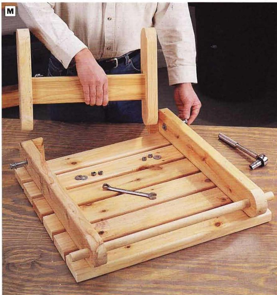
**PHOTO M:** Attach the foot rest stretcher to the legs with 2½-in. deck screws, then join the leg assembly to the foot rest with bolts, washers and double nuts.
