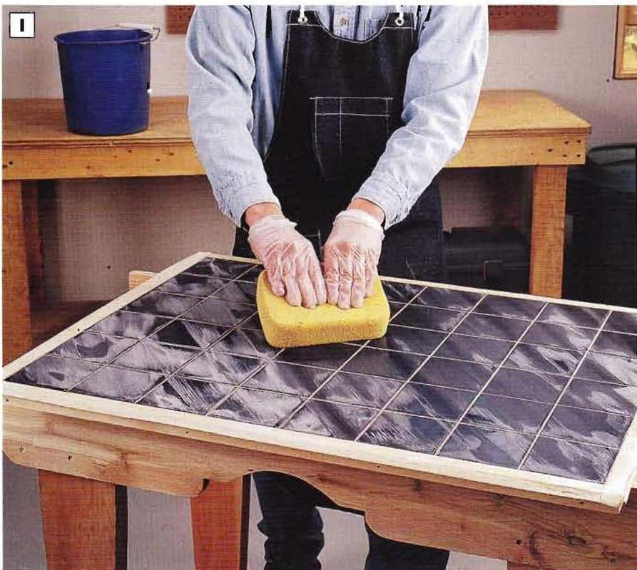
**PHOTO I:** Remove excess grout and smooth the grout lines with a water-dampened sponge. Again, work diagonally. Continue wiping the tiles, rinsing the sponge and wringing it out until the tiles are clean. Wipe away haze left by the grout with a soft cloth.
