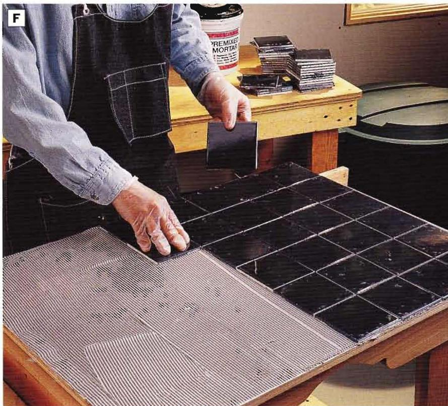
**PHOTO F:** Spread a layer of thinset mortar over the subtop using a 1/4-in. notched trowel. Press the tiles into the mortar in a systematic fashion, working out from one corner both lengthwise and widthwise. Keep watch on your tile spacing to ensure that all the tiles will fit on the subtop.
