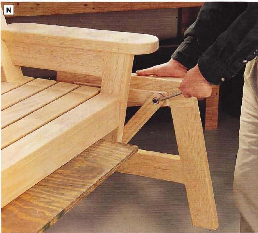
**PHOTO N:** Set the bench on your work surface so the glider arms hang freely. Attach the glider arms to the blocking pieces on the glider stand end assemblies with pivot hinges.
