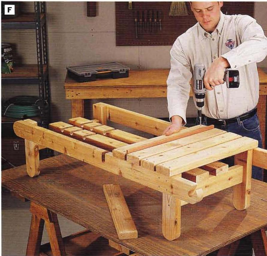
**PHOTO F:** Screw the five seat slats to the seat rails. Determine and mark the positions of the end slats first, then space the remaining three slats evenly between the end slats. If the slat space is consistent on your chair, use a scrap spacer to make spacing easy when fastening the parts.
