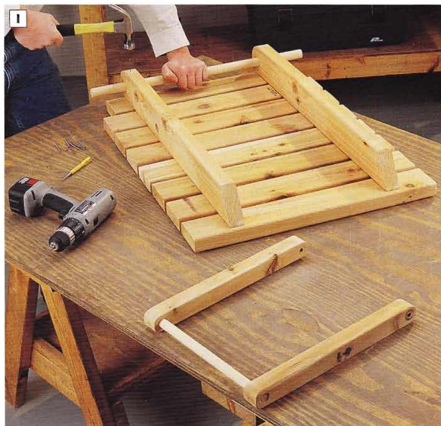
**PHOTO I:** Tack the back rest dowel in place on the back rest rails with #6d galvanized finish nails. Drive the nails through the rails and into the dowels. To keep the dowels from splitting, drill a pilot hole for the nails first.
