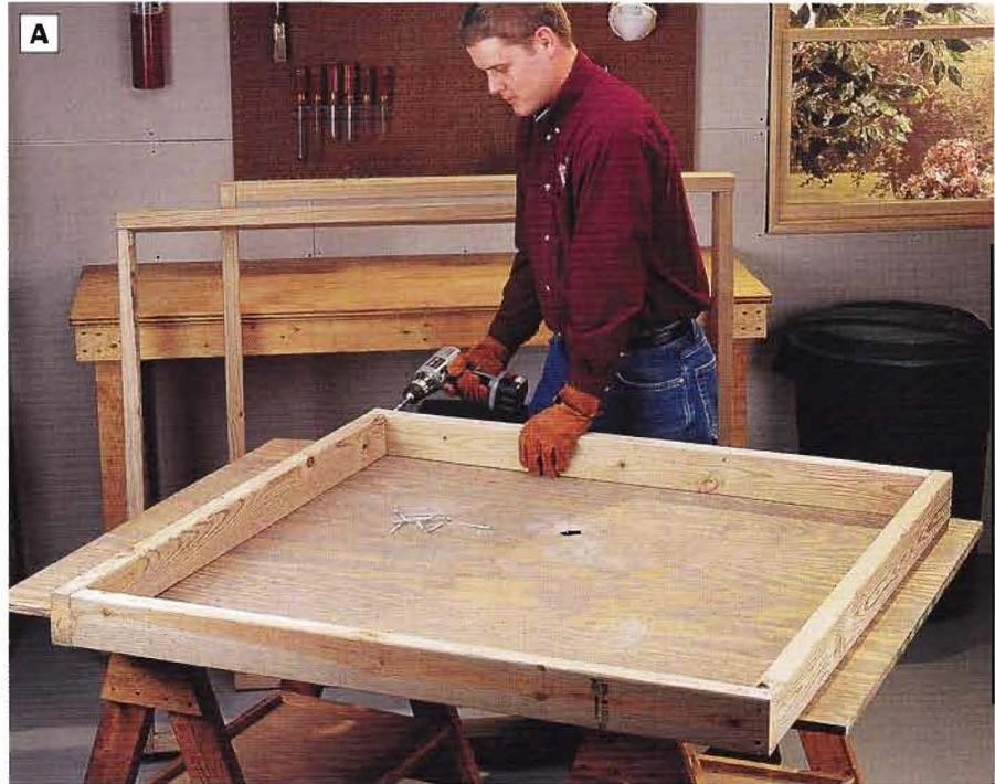
PHOTO A: Place the parts that compose each tier in position on your worksurface, alternating the orientation of the butt joints around the tier. Attach the parts with countersunk 3-in. galvanized deck screws. It's a good idea to wear gloves when working with treated lumber.
