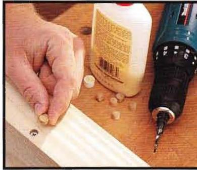
**STEP 2:** Drive the screw into the hole until it stops at the bottom of the counterbore. Glue and insert a wood plug cut from the same wood species or from a piece of dowel.
