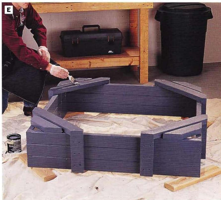
PHOTO E: Apply latex primer to all exposed surfaces of the sandbox, then follow up with two coats of exterior latex paint. We covered the whole box in a single color, but you could also create a multi-colored paint scheme instead.
