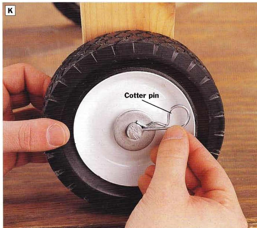
**PHOTO K:** Insert the axle through the holes in the front legs, then install washers, wheels and cotter pins to secure the wheels. The washers next to the cotter pins keep the wheels from rubbing against the cotter pins as the wheels turn.
