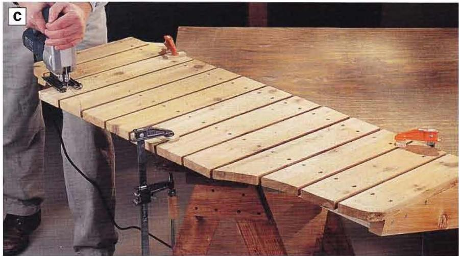
**PHOTO C:** Once you've marked the profile (either your own design or the one we've provided in the drawings) on the back slat assembly, trim along the profile lines and smooth the cut edges.
