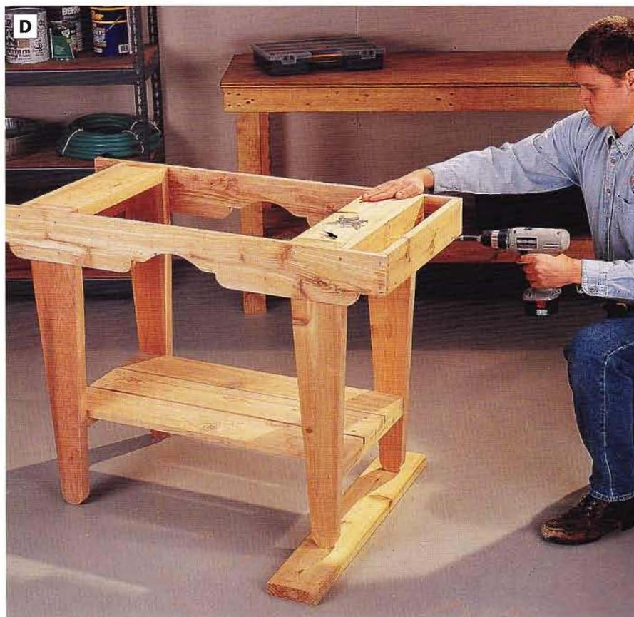
PHOTO D: Fasten the shelf slats in position, then attach the condiment shelf and front to the side aprons. Leave a 1/4-in. gap between the condiment shelf and the end apron (See *Side Aprons* drawing, page 33), to allow for water drainage. Use 2-in. galvanized deck screws on these parts.
