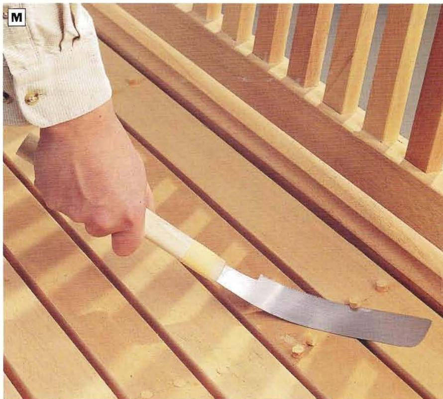
PHOTO M: After the glue dries, trim the plugs with a flush-cutting saw. Given the cup in the seat, use a flexible blade saw that can adjust to the contour of the slats. Be careful not to mar the seat slats as you trim against them.
