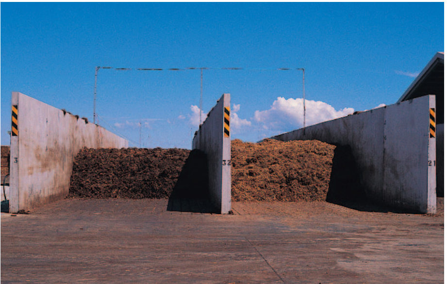
Air pumped through the concrete floor assists in the preparation of the compost. Meadow Mushrooms, New Zealand. (Buchanan)
