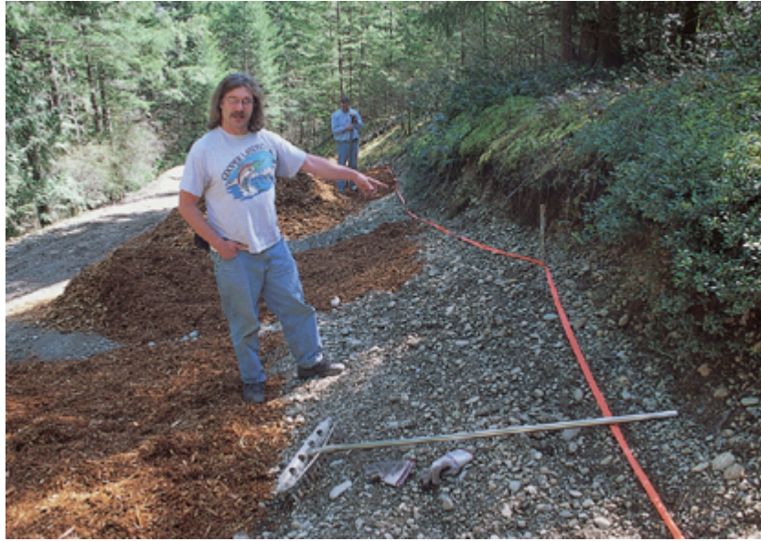
FIGURE 92 David Sumerlin points to location where wood chips should be placed—up against the bank of the scar face of the road cut, thus eliminating erosion from the silt-producing exposed surface.
