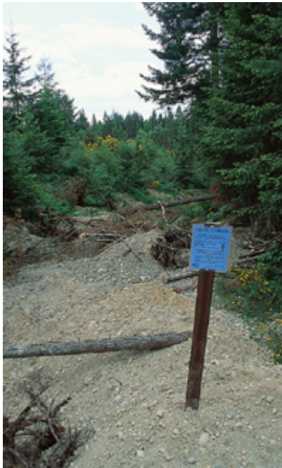
FIGURE 88 Depicted here is the conventional approach to reclaiming a road: digging deep ditches (called tank traps in military speak; I call them “terra interrupti”) that block vehicles so that, ostensibly, the land can recover from human activity by disturbing it further.
