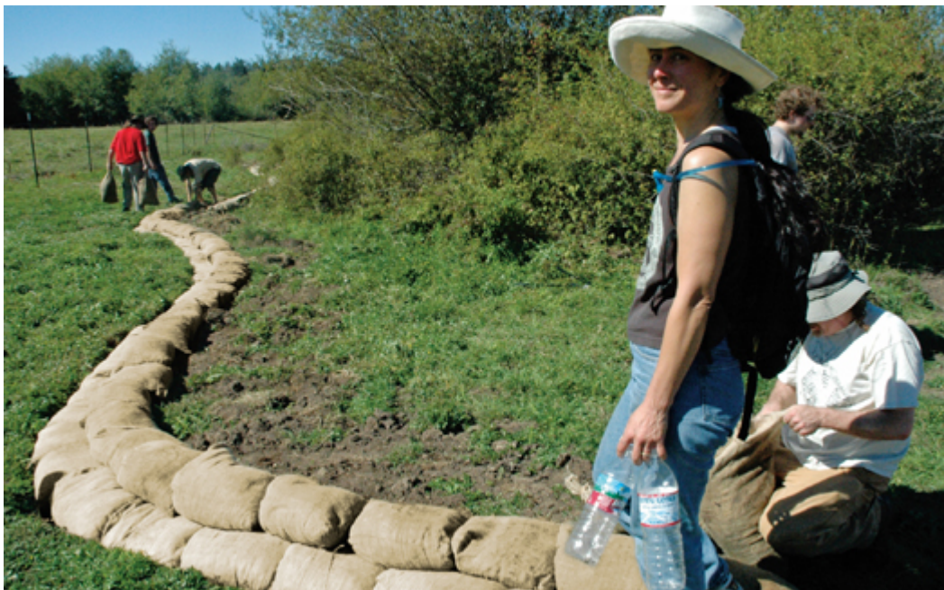
FIGURE I To reduce coliform bacteria from an upland farm, two rows of woodchip-filled burlap sacks, inoculated with oyster mushroom mycelium, catch surface water before entering a sensitive salt-water estuary in Mason County, Washington, USA. Rows of myceliated bags are added annually as a best management practice. I prefer using woodchips from storm-created debris and inoculating with a native mushroom with proven antimicrobial properties. Similarly, such an arrangement can be used to catch and destroy chemical effluents.
