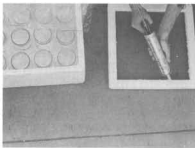
fig. 18: Applying silicone marine glue.
