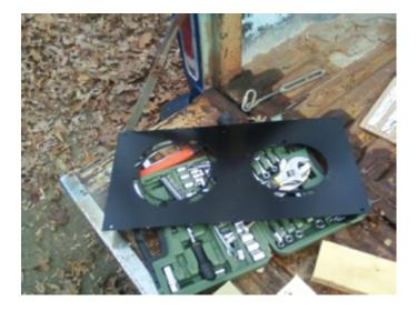
Once the plate arrived, I measured it and built a frame of scrap  $2\times4$ . The plate measured  $12\times24$  so I cut two 2-foot lengths of  $2\times4$  and 2 9-inch lengths. After screwing them together, it made a perfect frame.
