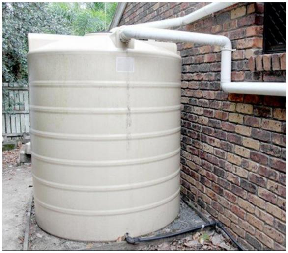
Collecting rainwater is one of the fastest ways to get access to fairly fresh and clean water. This is a great first project, as it's very simple to set-up and offers immediate benefits to the user. Rainwater harvesting can provide the user with their own water supply, independent of the city. This water can be used freely for any purpose and doesn't apply to water restrictions in counties that have them.
