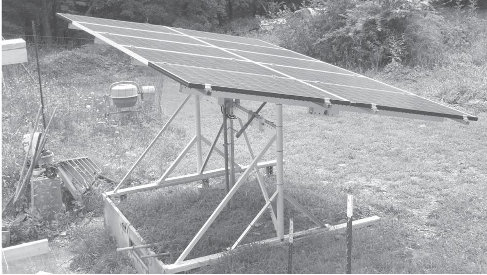
Metal racking with monthly repositioning
