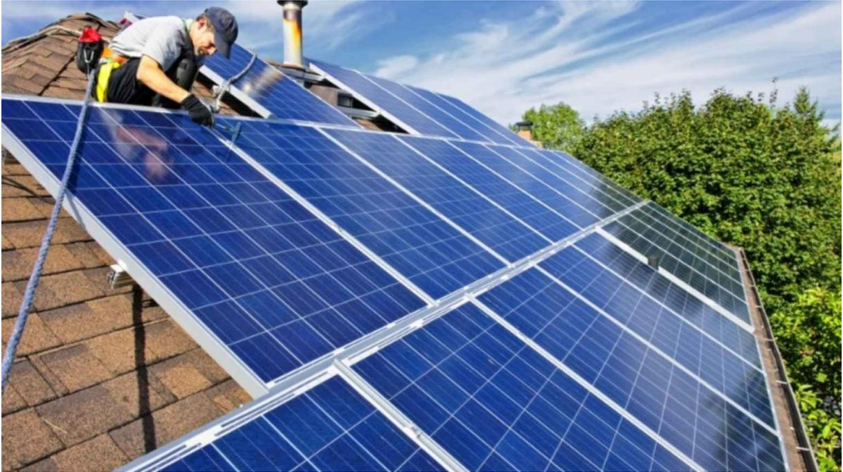
To install solar panels, you must necessarily be comfortable with working with heights, roofing, and waterproofing to avoid water leaks. This is done by installing hooks, rails, or battens. Depending on the solar panels and their method of attachment, you may need to install an under-roof screen or a waterproofing system. A good physical aptitude is also necessary to intervene on a roof and handle the voltaic panels.
