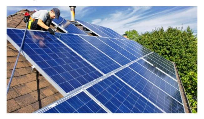
To install solar panels, you must necessarily be comfortable with working with heights, roofing, and waterproofing to avoid water leaks. This is done by installing hooks, rails, or battens. Depending on the solar panels and their method of attachment, you may need to install an under-roof screen or a waterproofing system. A good physical aptitude is also necessary to intervene on a roof and handle the voltaic panels.
