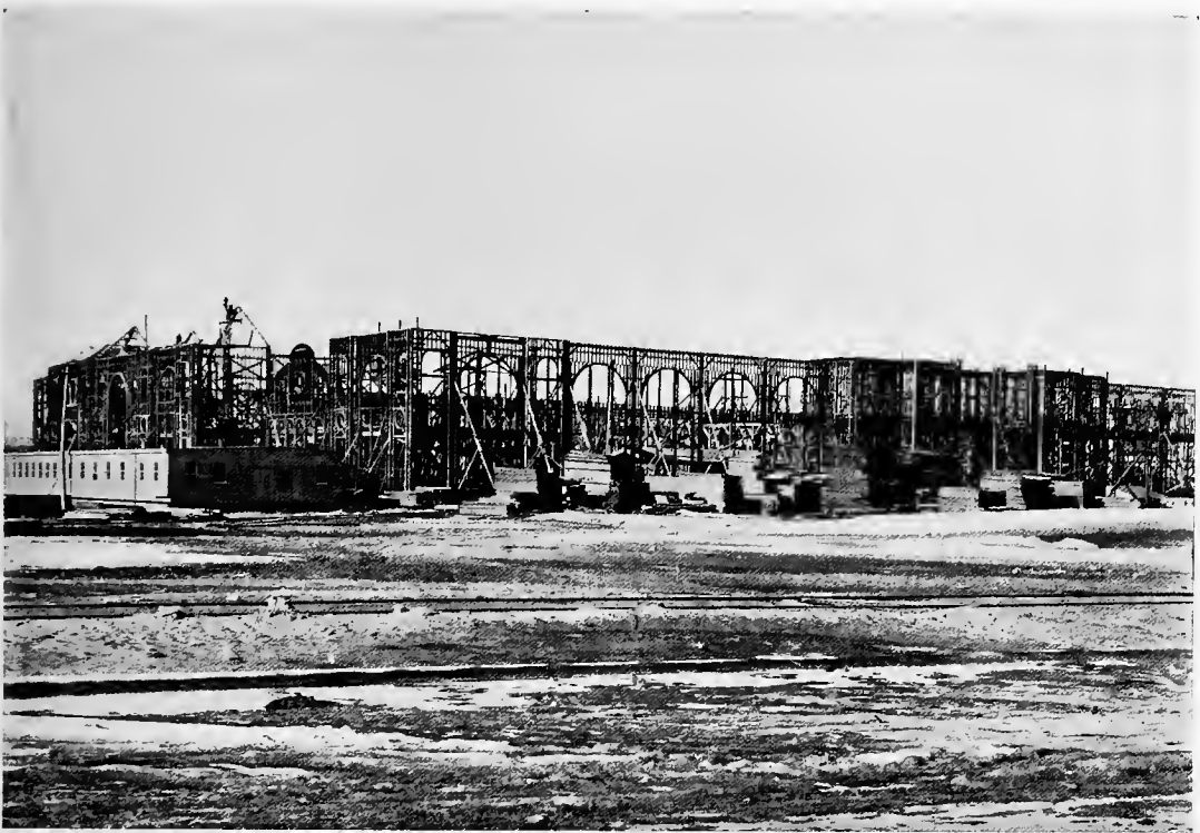
THE GOVERNMENT BUILDING, JANUARY 29, 1892.
