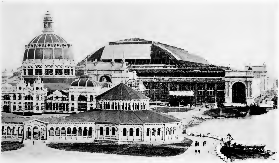
APPROACHING COMPLETION. LOOKING SOUTHEAST.
