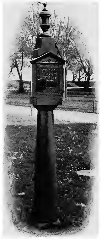
A FIRE SIGNAL BOX.
