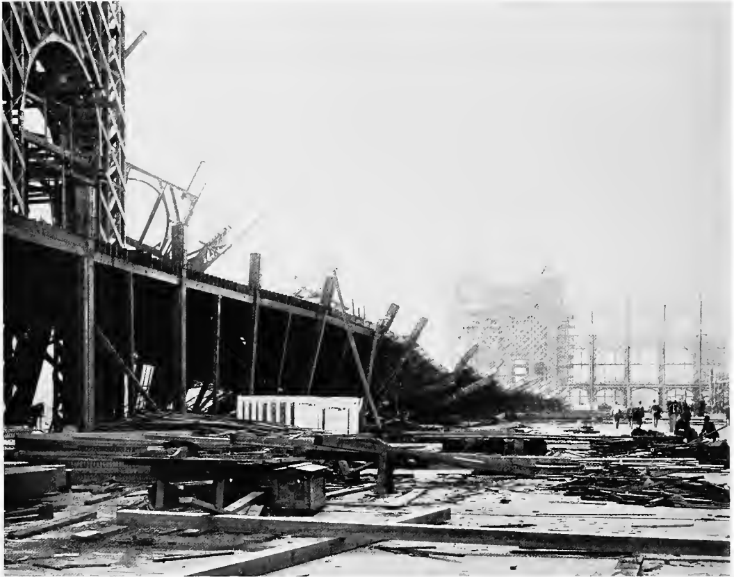
WEST SIDE OF THE MANUFACTURES BUILDING after the gale, April 27, 1892,
