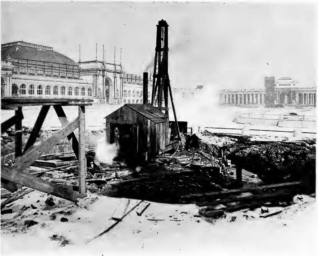
CONSTRUCTION OF THE SOUTH ELECTRIC FOUNTAIN.
