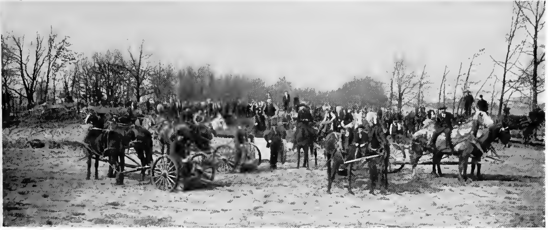
Working on the Midway Plaisance, March 24, 1892.
