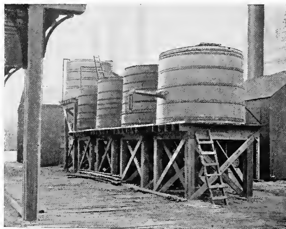
Tanks for purifying drinking-water.
