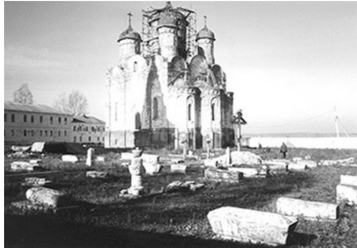
Fig. 14.28. The Louzhetskiy Monastery in Mozhaysk. We see the courtyard. In 1999, some two metres of the turf were removed. The former level of soil can be judged by the dark strip at the bottom of the monastery's cathedral. One can also see that the windows of the cathedral have been elevated except for one window, which had been at ground level when the excavations were conducted. In the foreground we see a few sarcophagi of the XVII-XIX century, unearthed during excavations and arranged in accurate rows. The level of soil in the courtyard now corresponds to that of the XVII century. Photograph taken in 2000.
