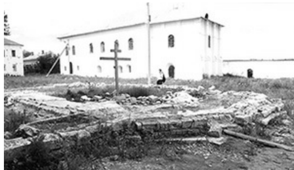
Fig. 14.30. Louzhetskiy Monastery in Mozhaysk. The foundation of a destroyed XVII century church with old Russian headstones used as construction material. According to the writings on the headstones, we see the remains of construction works conducted in 1669 or later. Photograph taken in 2000.
