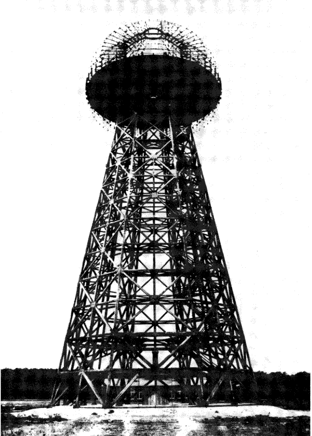
Figure 84. Transmitter at Wardencllyffe, erected in 1901 for purposes of "world telegraphy." (Long Island Plant)
