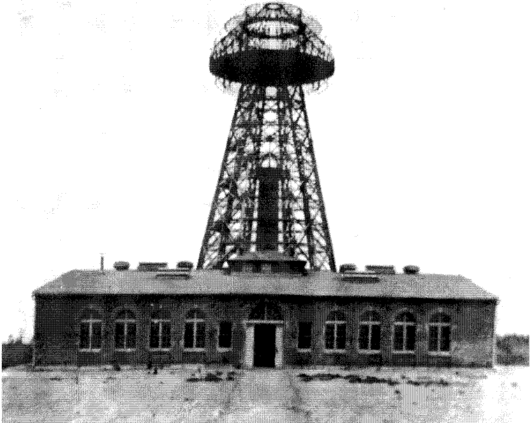
Figure 85. View of the plant. (Long Island Plant.)
