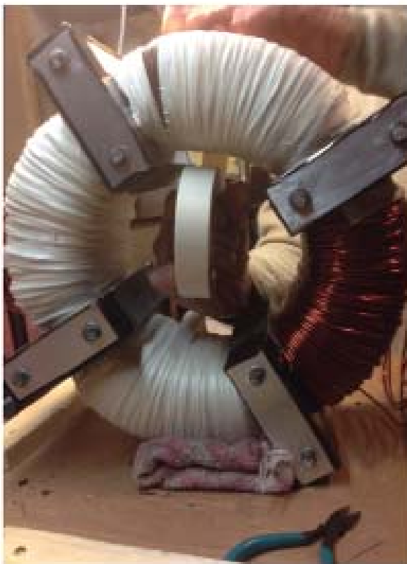
Installing outer wrap on core
